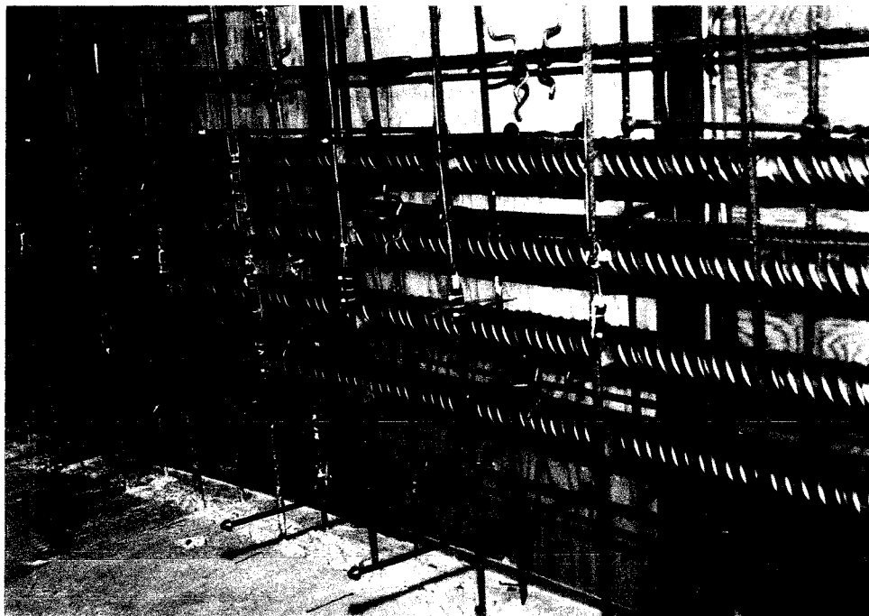
Figure 4.15 1.0DC Duct Arrangement (Close-Up).
