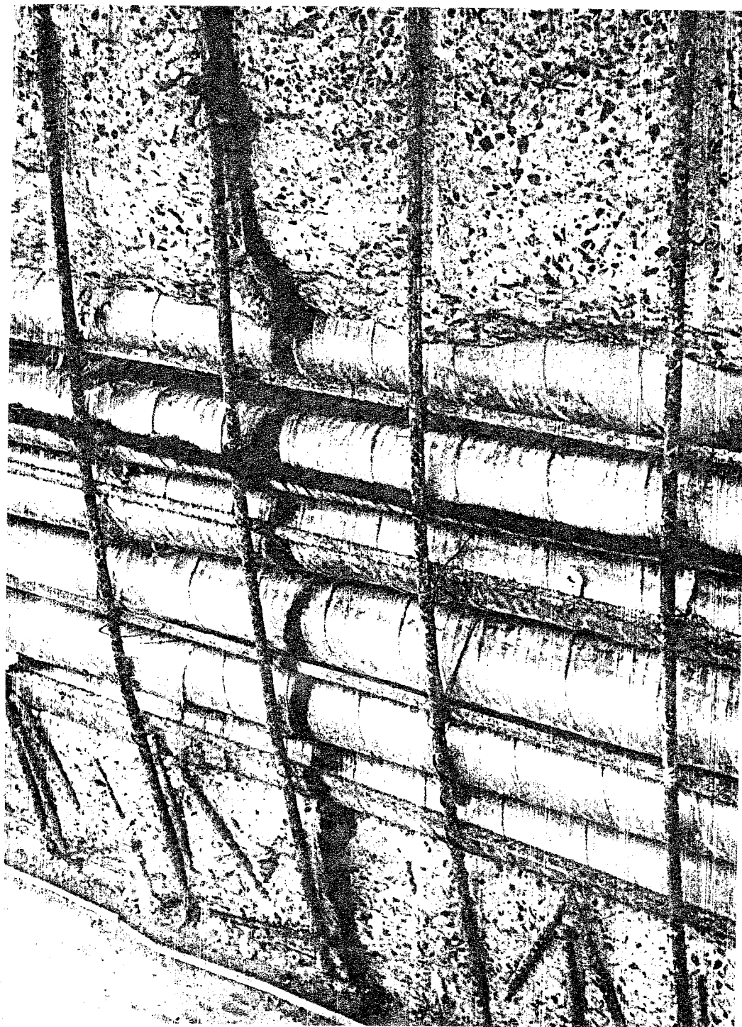
Figure 1.9 Kapiolani Close-up View During Repair (from Ref. 8).
