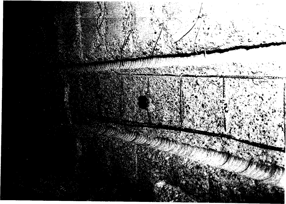
Figure 6.9 1.0DC Failure Plane After Removing Concrete Panel.
