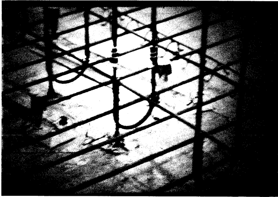
Figure 4.8 Stirrup Alignment System.
