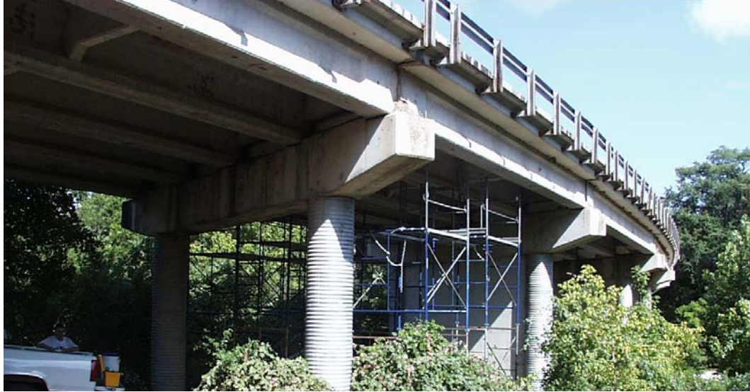
Figure A.17 Photograph of Wimberley Bridge
