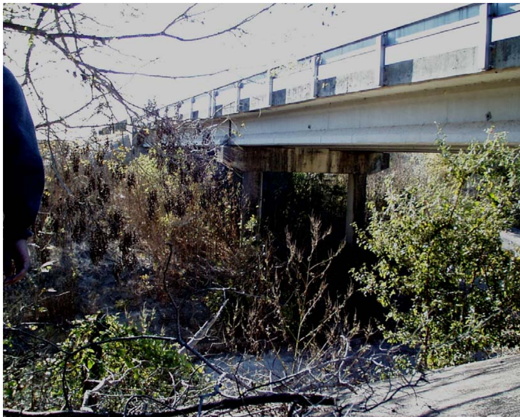
Figure A.13 Photograph of Willis Creek Bridge
