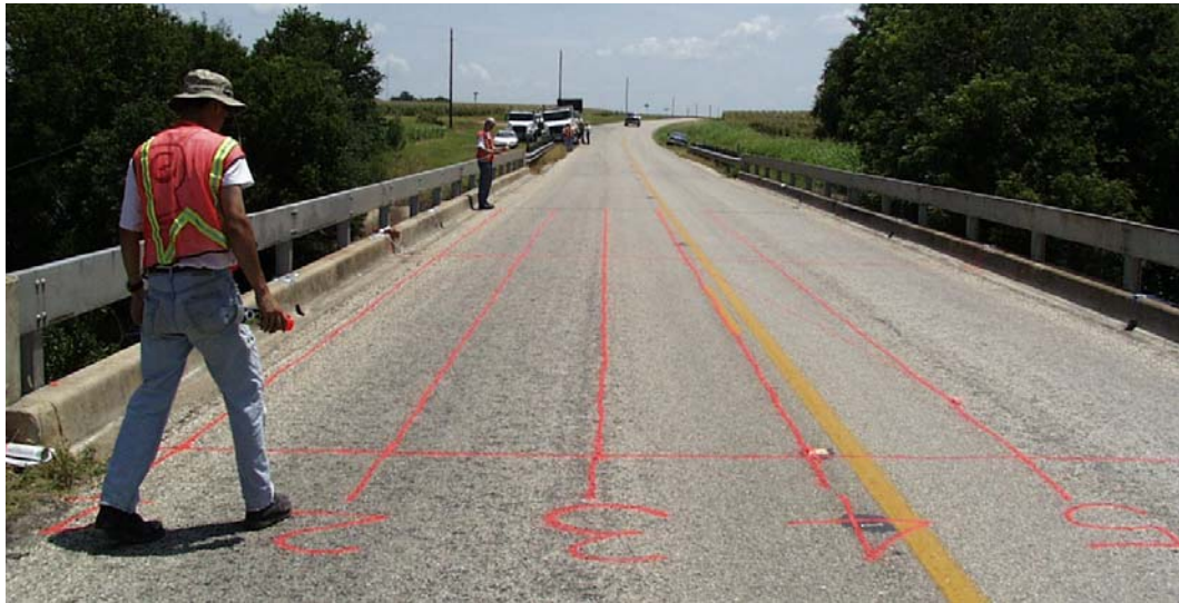
Figure 3.18 Photograph of Load Paths at Willis Creek Looking East
