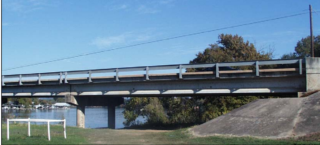
Figure A.5 Photograph of Lake LBJ Bridge
