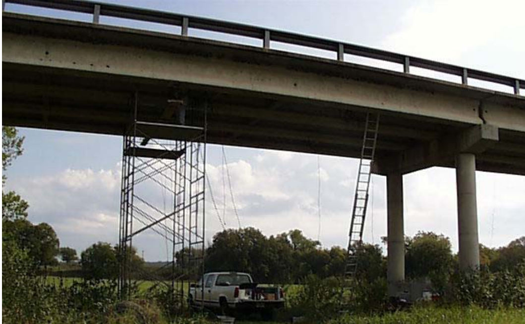
Figure A.9 Photograph of Lampasas River Bridge
