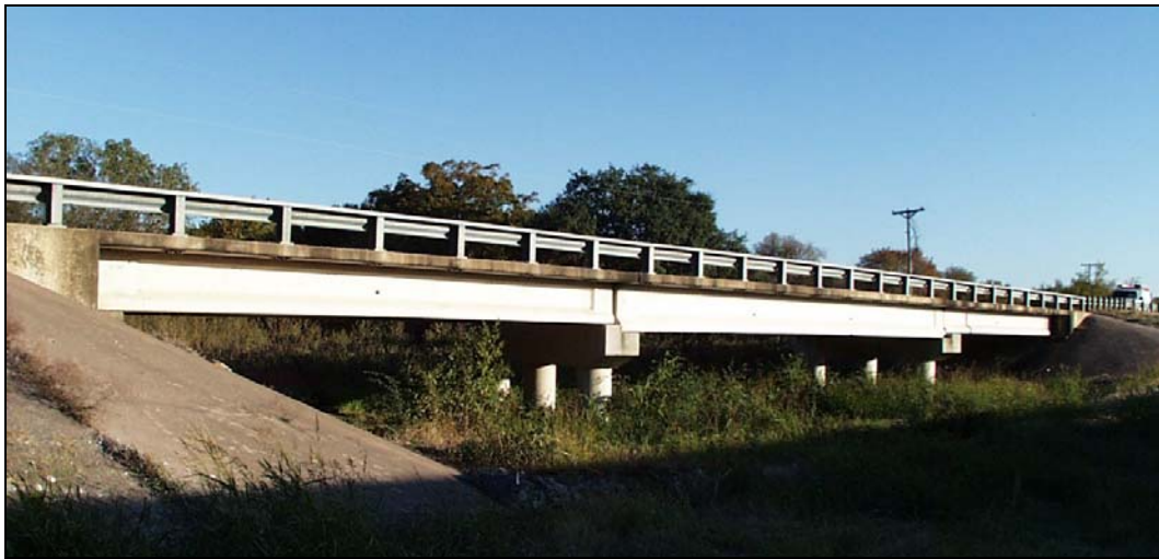
Figure A.1 Photograph of Chandler Creek Bridge
