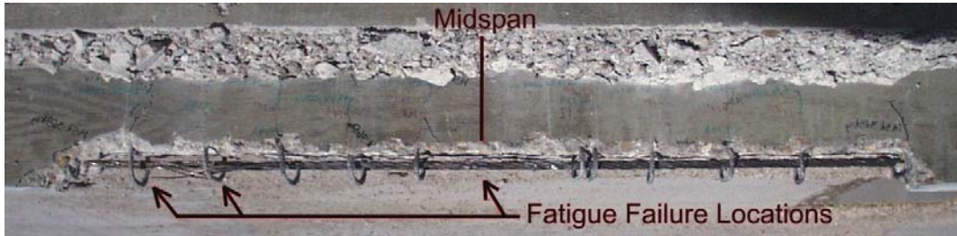
Figure 6.54 Photograph of Beam 5 After Removal of Concrete to Expose Strand (Heller 2003)
