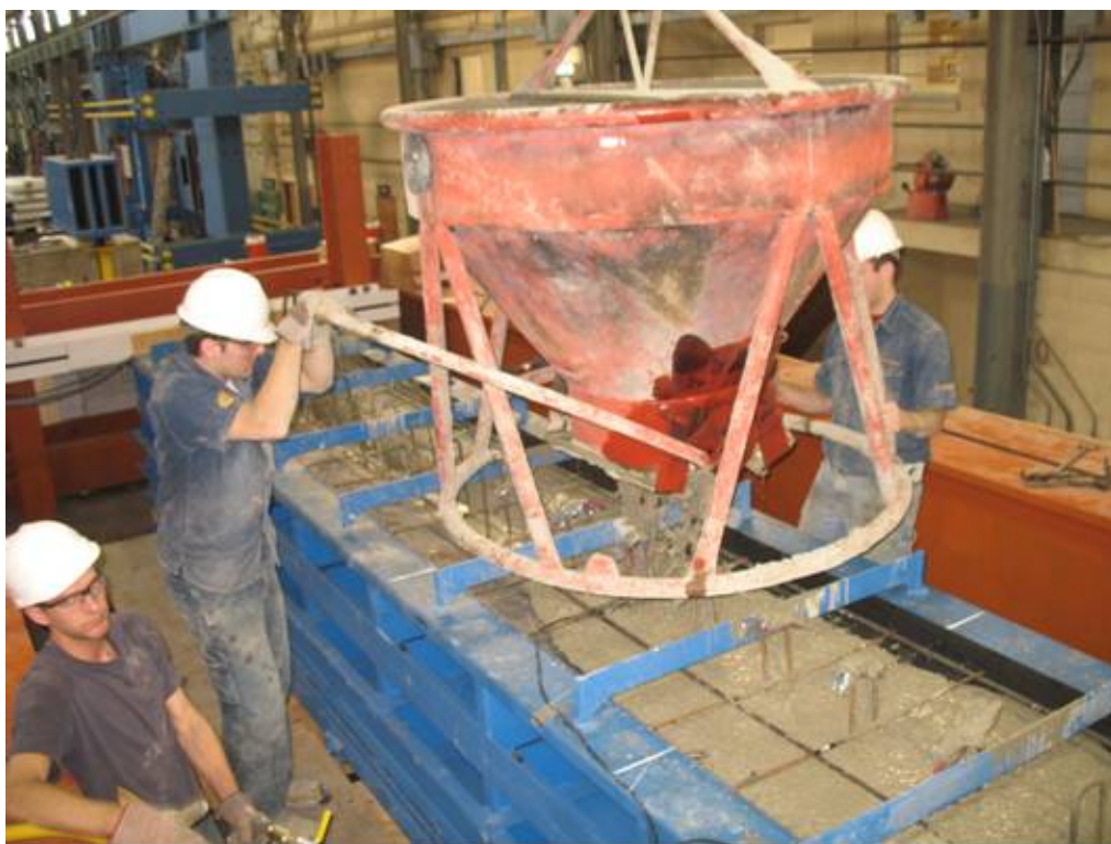
Figure 3-46: Concrete placement using a 1 cy hopper
