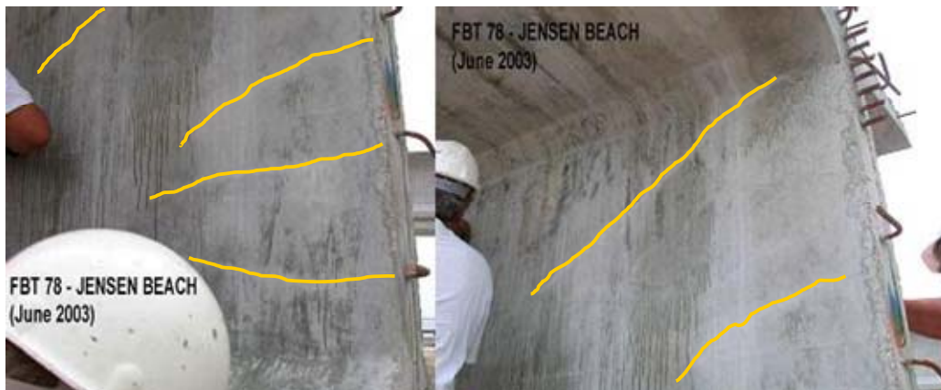
Figure 1-1: Bursting and Spalling Cracks in Florida Bulb Tees: Jensen Beach (Courtesy of Jonathan Van Hook, Florida DOT)
