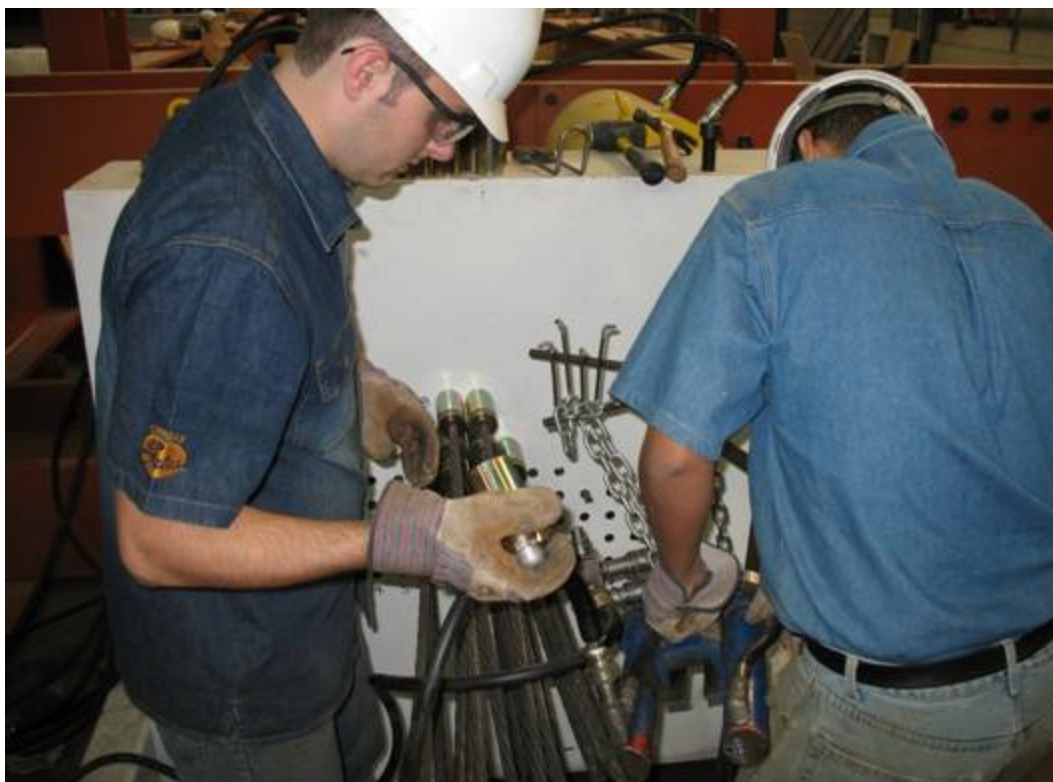
Figure 3-40: Individual strand stressing with mono-strand stressing jack
