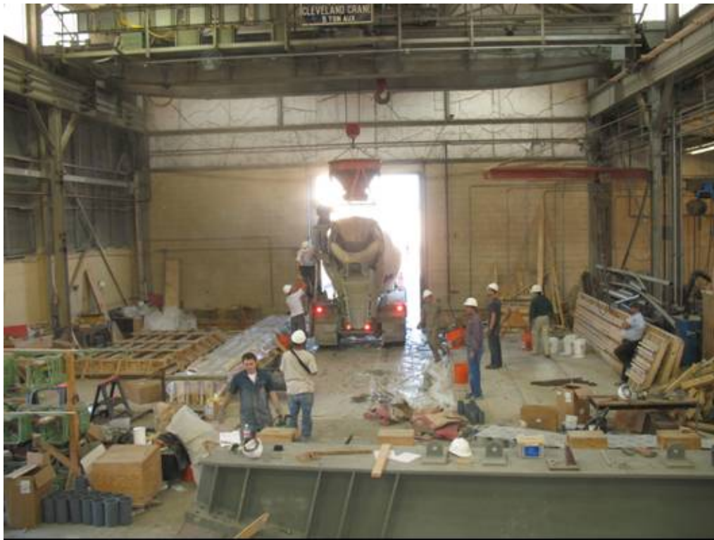
Figure 3-45: Cement being added to the ready mix truck with a 1 cy hopper
