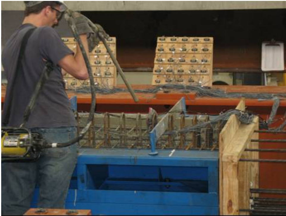
Figure 3-48: Use of an internal rod type vibrator: Tx28 girder
