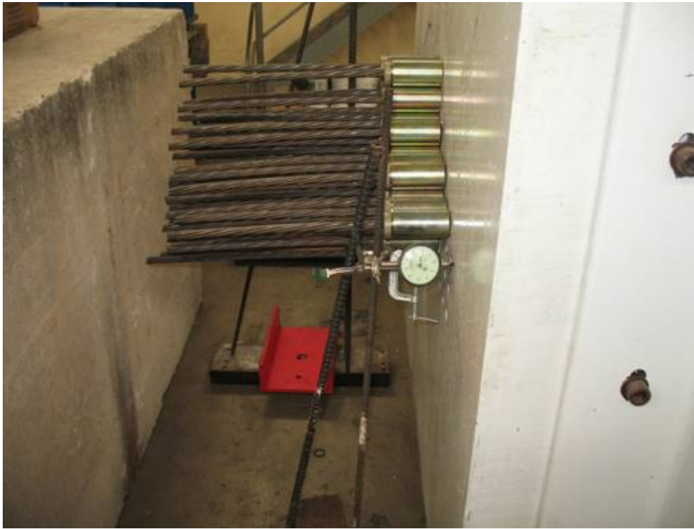
Figure 3-43: Dial gauges used at dead end of prestressing bed to measure frame deflection
