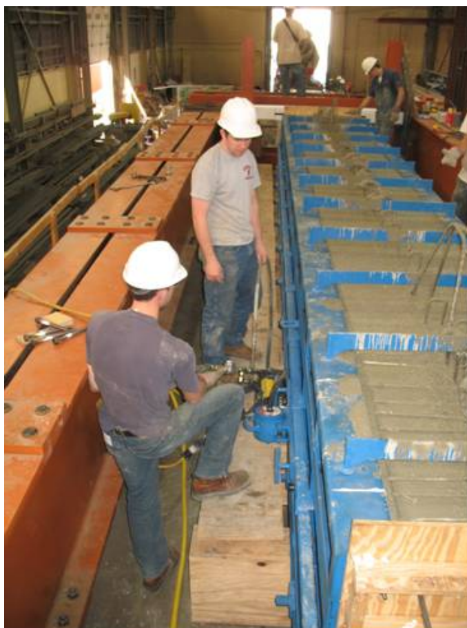
Figure 3-47: Form vibrator being used on a Tx28 girder
