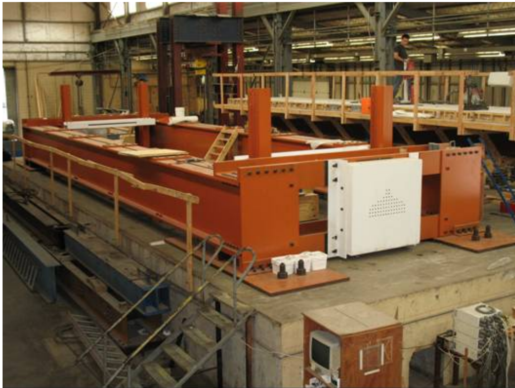
Figure 3-19: Completed Pretensioning Bed
