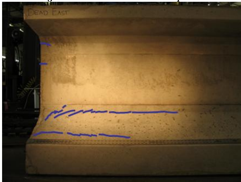
Figure 4-32: Tx46 Dead end photo with crack pattern
