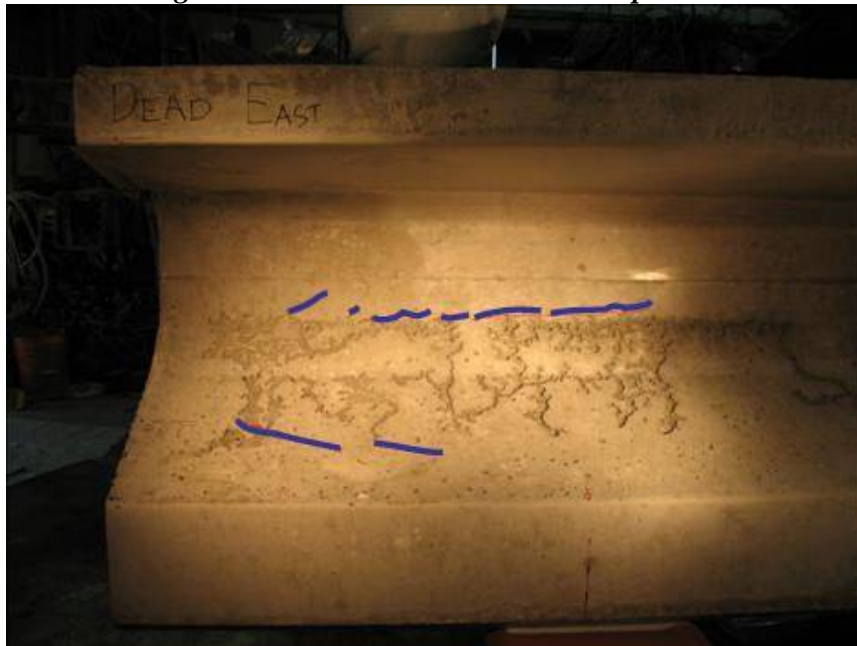
Figure 4-15: Tx28-I Dead end photo with crack pattern
