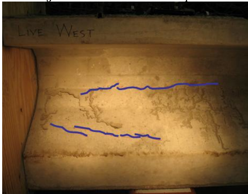
Figure 4-13: Tx28-I Live end photo with crack pattern
