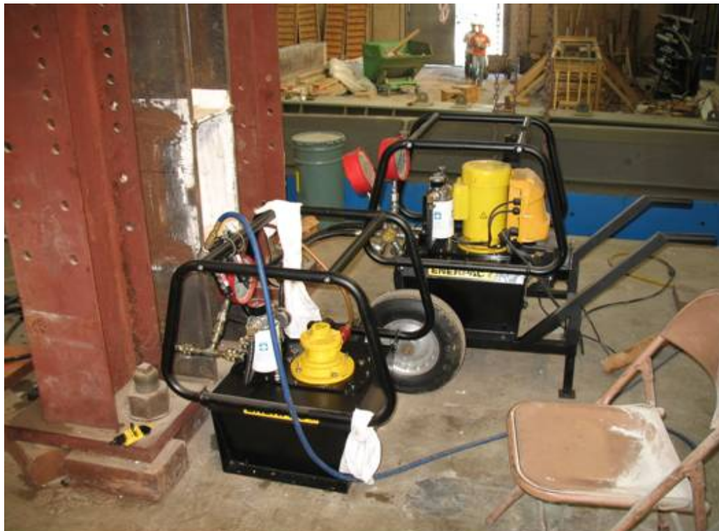
Figure 3-41: Hydraulic pumps used to control the application of prestressing force through four 400-ton rams
