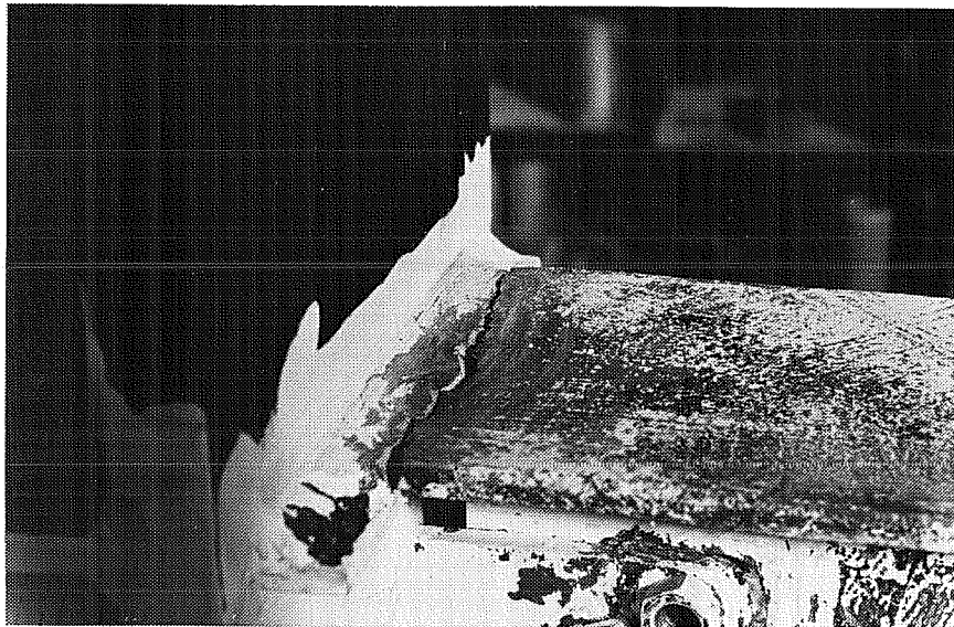
Figure 3.11 - Top Flange Failure in Specimen 3
