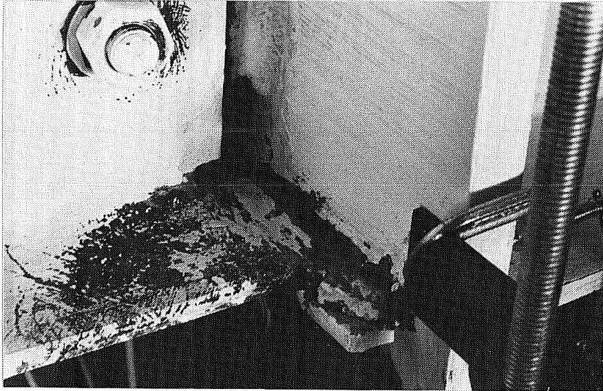
Figure 3.2 - Bottom Flange Failure in Specimen 1
