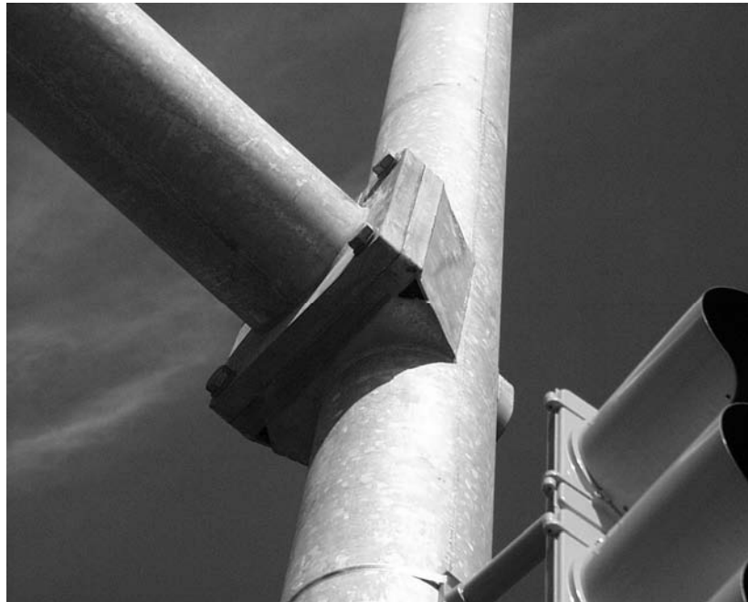
Figure 1.2 Built-Up-Box Connection Detail
