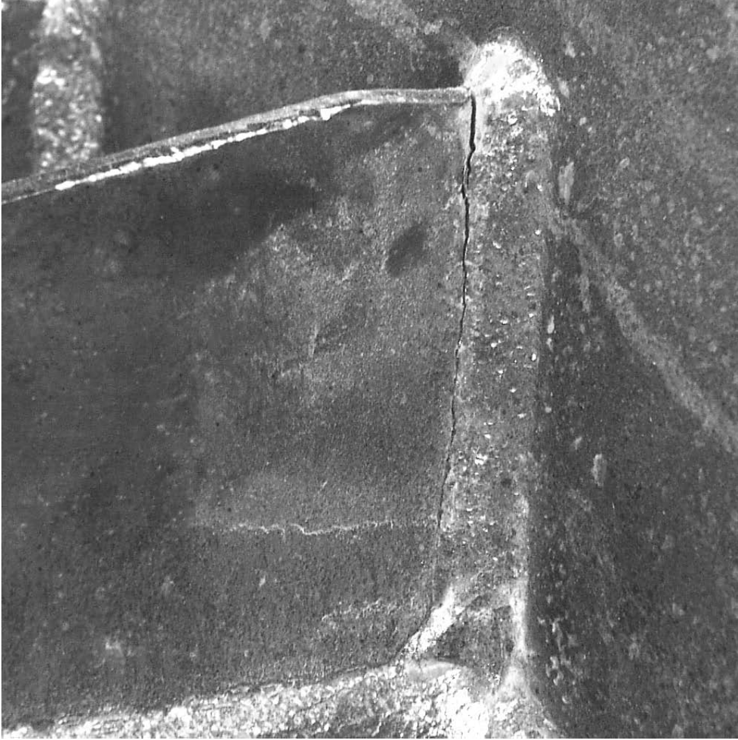
Figure 7.25 Failure of U-Rib Stiffened Specimen
