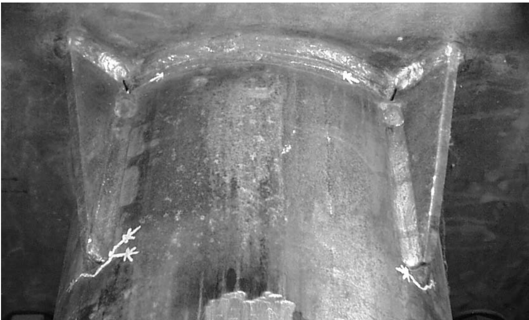
Figure 7.12 Failure of VALN 6x3/8@45 Specimen – Paint lines at termination of stiffeners represent extents of visible cracking, and painted arrows indicate visible crack tips in socket weld toe, specimen tested at 12 ksi stress range
