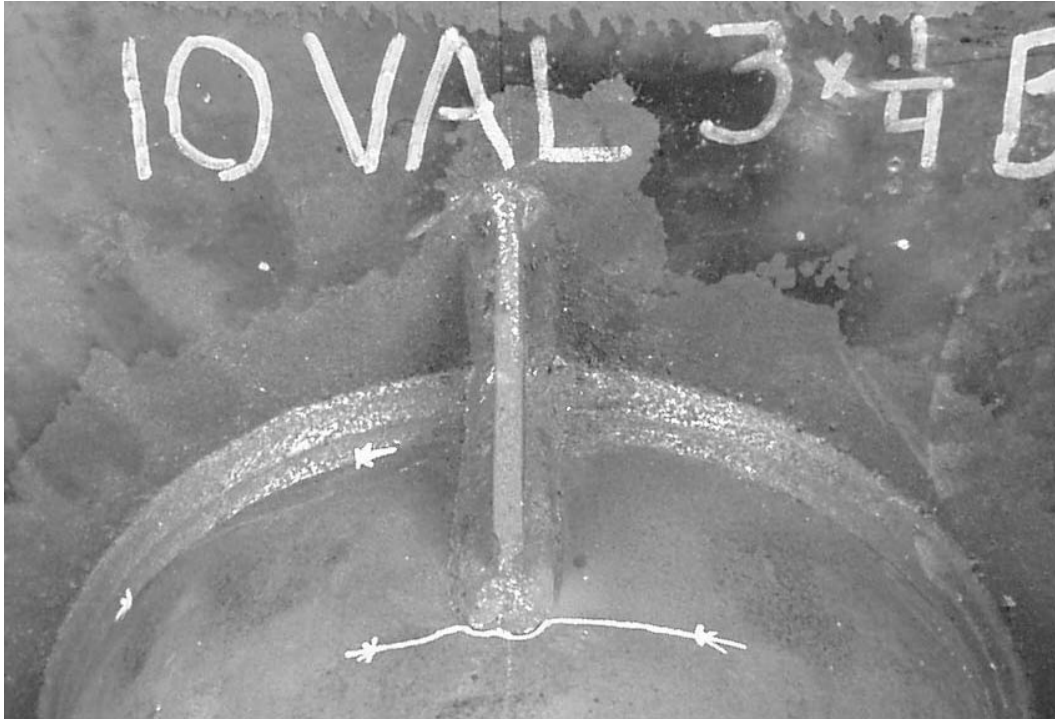
Figure 7.8 Failure of VAL 3x1/4 Specimen – Note: Paint line at termination of stiffener represents extent of visible cracking, and painted arrows indicate visible crack tips in socket weld toe
