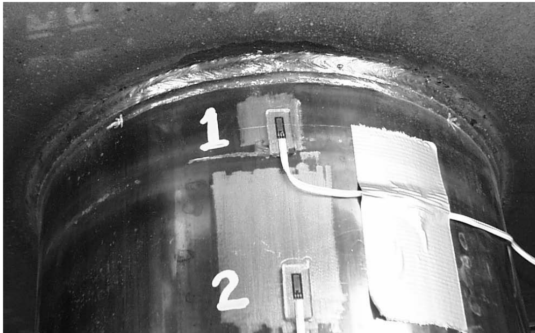
Figure 7.31 Failure of Full-Penetration Welded Connection Detail Specimen – Paint arrows indicate extent of visible cracking
