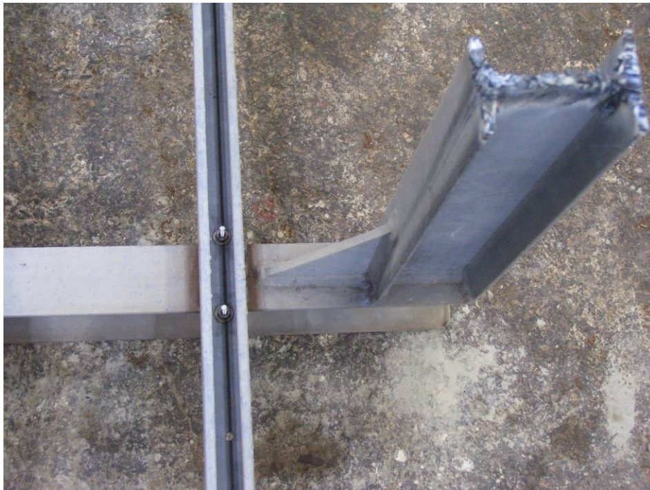
Figure 1.3 Critical Fatigue Detail
