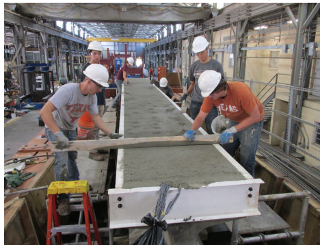
Figure 2: 0.7-inch team casting the deck on the first test specimen
