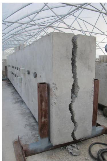
An example of the damage that ASR can cause - Condition of the 5-foot-tall wall segment after completion of the out-of-plane monitoring efforts
