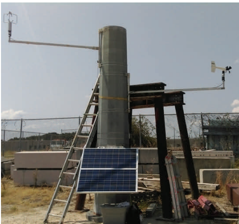
Figure 1: Anemometers and solar panel installed on a mock-up pole
