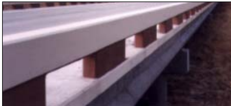
Figure 1.1 – TxDOT T203 bridge barrier with concrete parapet
