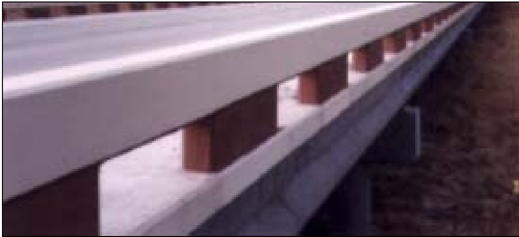
Figure 4.1 – TxDOT T203 bridge barrier with intermittent base and concrete parapet
