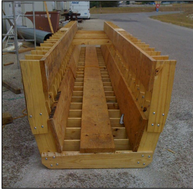
Figure 37: Wooden interior void during construction prior to plywood skin installation
