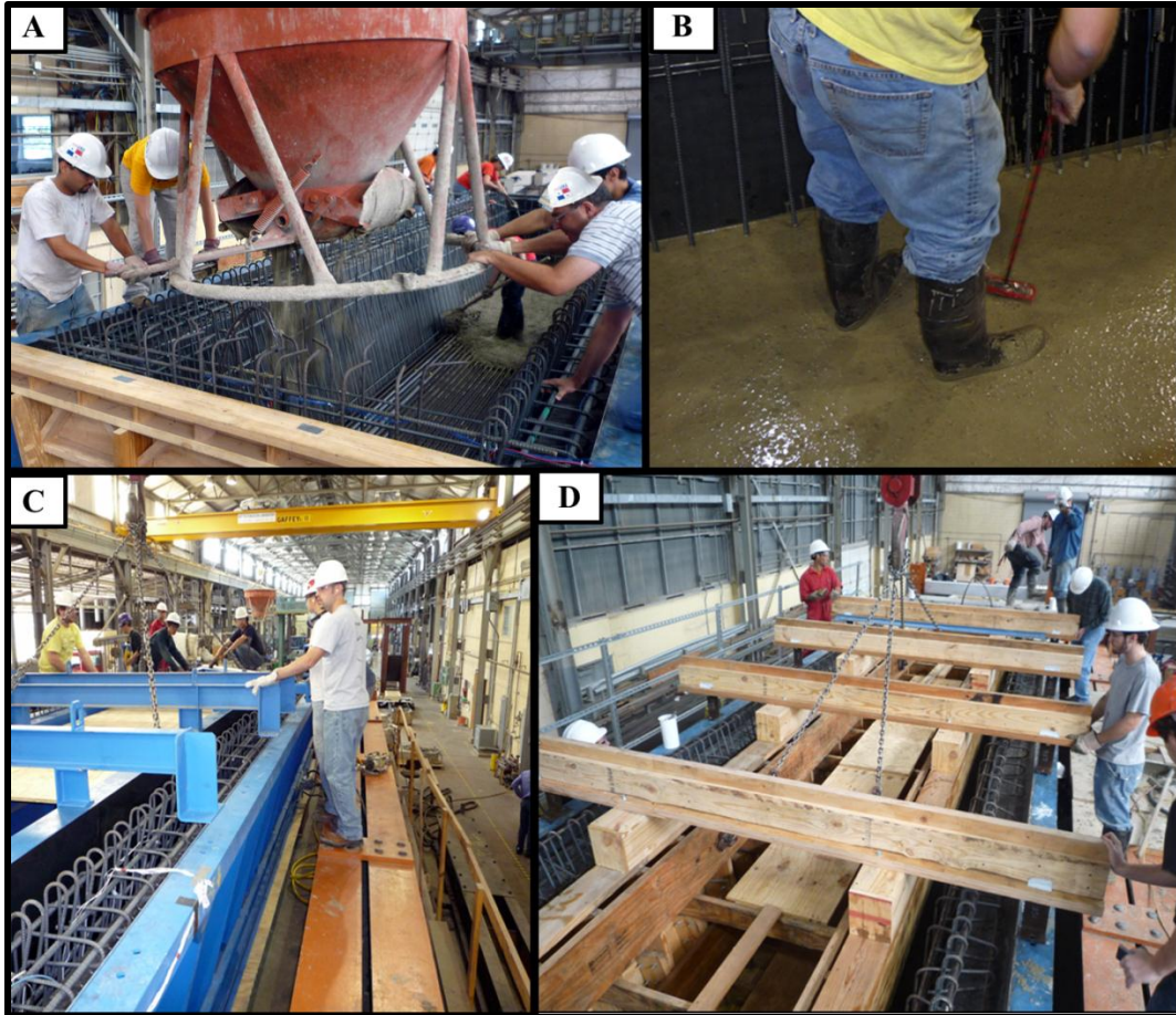
Figure 3-38: U-beam casting procedure: (A) Placement of bottom flange concrete (B) Checking thickness of bottom flange (C) Steel interior void (Beams 1, 2 & 3) installation (D) Wooden interior void (Beam 4) installation
