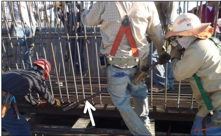
Figure 5-13: Manual Installation of Rebar Chairs for Beam 5
