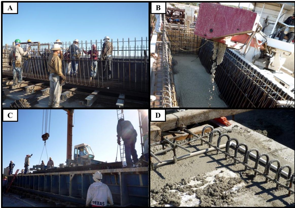
Figure 3-42: Construction sequence of Beam 5
