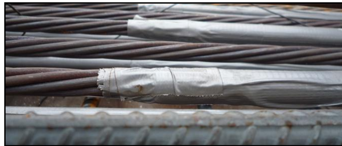
Figure 3-20: Debonding and sealing of strand
