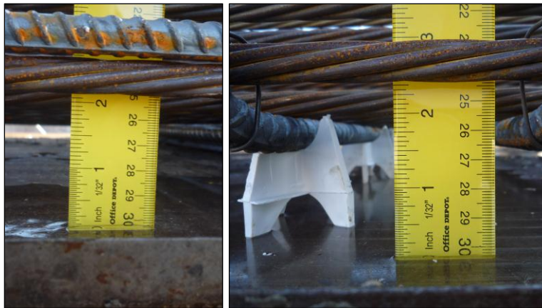
Figure 5-12: Bottom clear-cover in Beam 5
