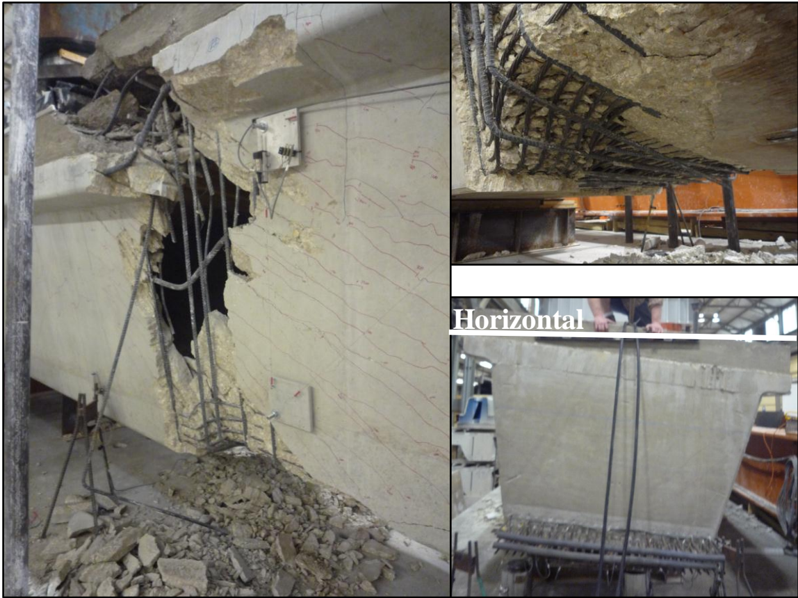
Figure C-9: Beam 5 North Failure
