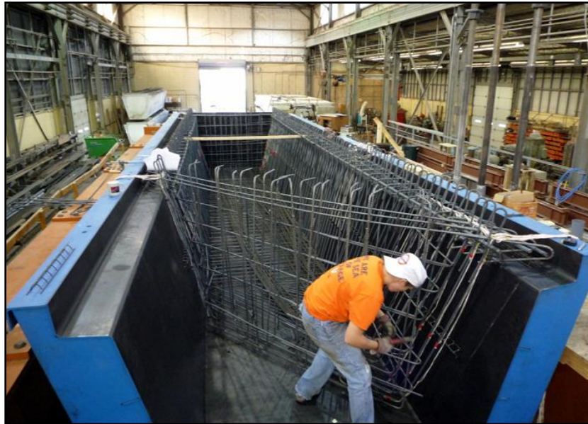
Figure 3-30: Assembly of mild steel reinforcement with sideforms in-place
