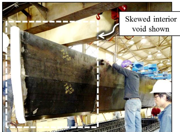
Figure 3-34: Custom interior void from Hamilton Forms
