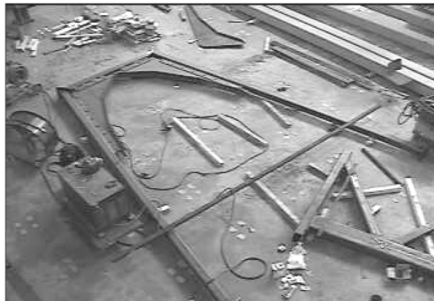
Figure 4.9- Pendulum support frame under construction at FSEL
