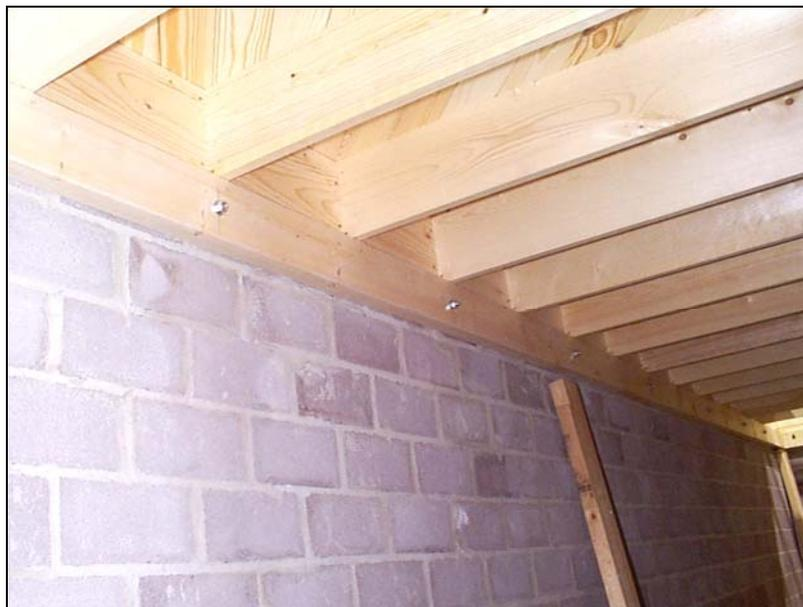
**Figure 3.5** Underside of diaphragm as built (Specimen #1)
