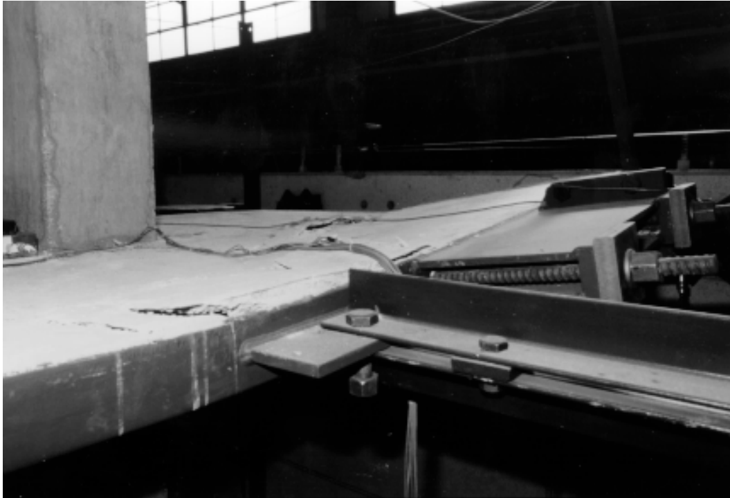
Figure 3.7: Failed Loading System at Third Floor, Viewed From the Southwest
