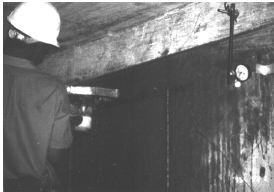
Figure 2.24: Panel Sawing Operation
