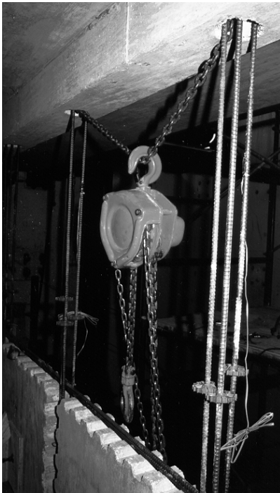
Figure 2.19: Crane Used for Panel Placement
