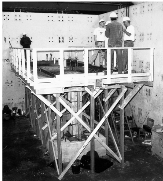
Figure 2.5: First Story Construction
