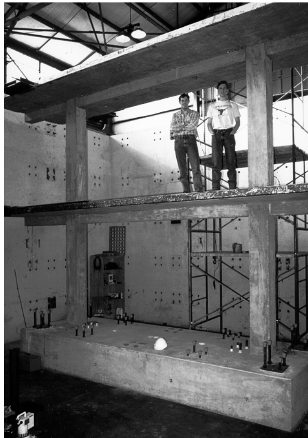
Figure 2.8: Completed Existing Frame
