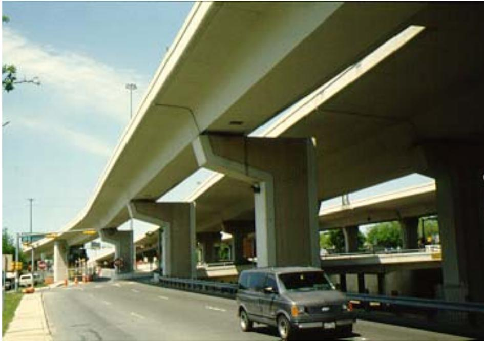
Figure 1.1 Cantilever Bents Supporting Entrance Ramp
