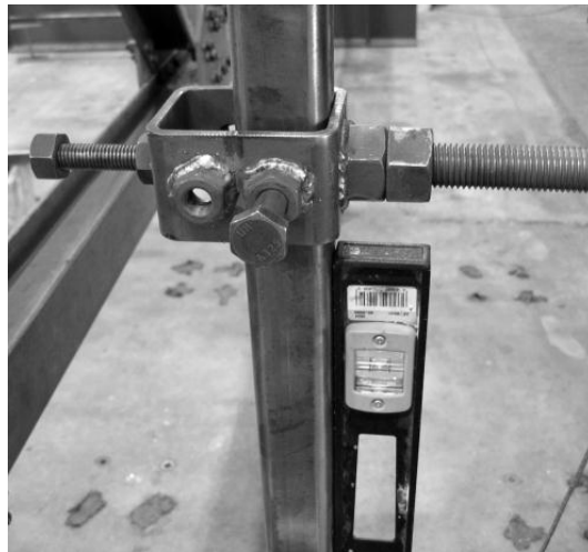
Figure 3.31 Checking of lateral brace vertical alignment
