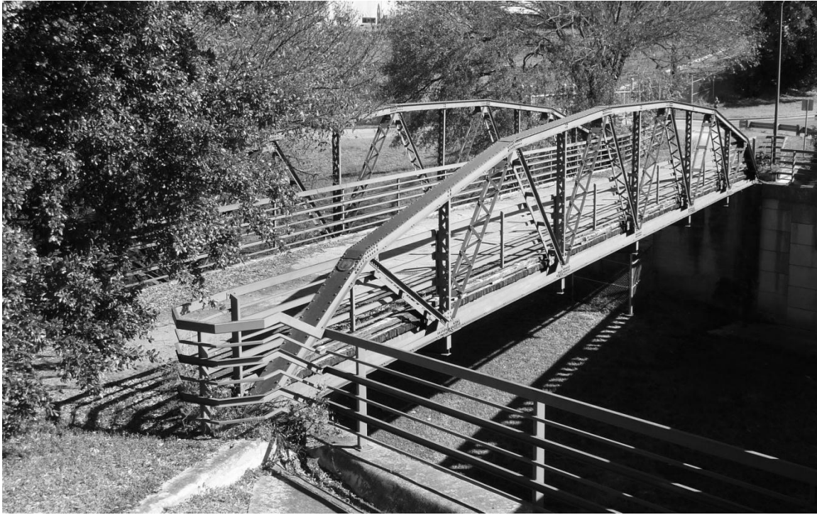
Figure 2.14 Pony truss bridge
