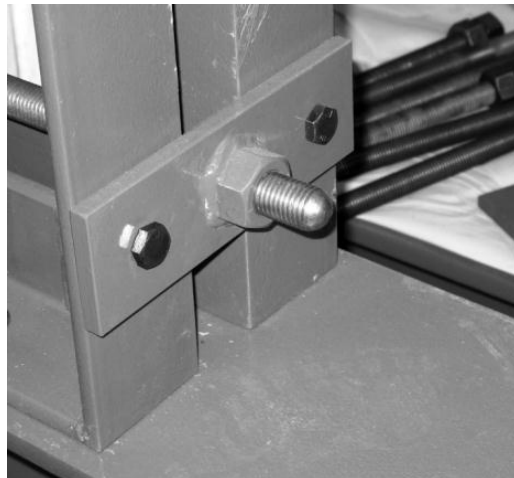
Figure 3.22 Rounded threaded rod at support
