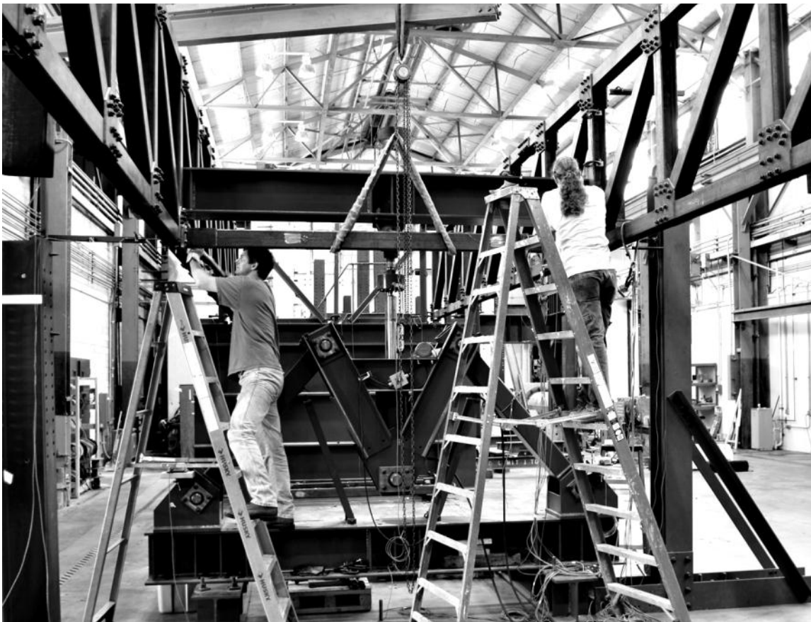
Figure 3.33 Installation of large torsional braces at bottom chord
