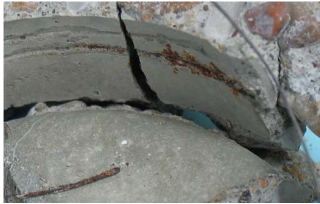
Figure 5-15 Corrosion Along Wire in Prism B25
