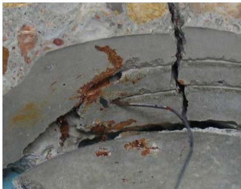
(a) Corrosion at 180° Bend in Wire
