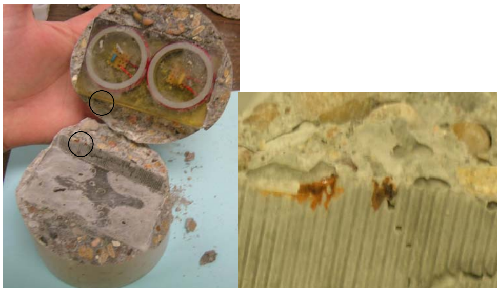
Figure H-8 Interior of Prism A30 Showing Location of Broken Wire
