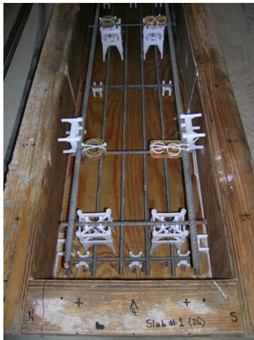
Figure 5-19 Slab #1 Prior to Placing Concrete
