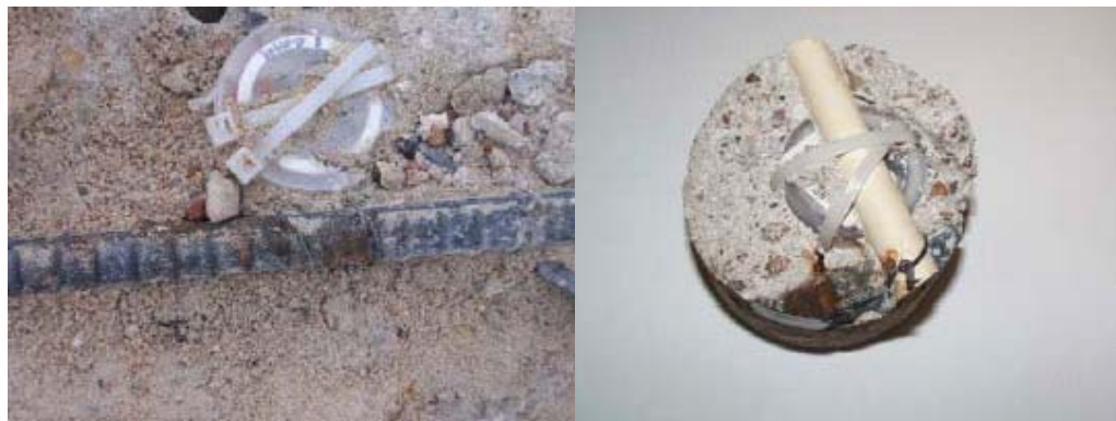
(a) Corrosion on Reinforcement Adjacent to a Basic Sensor at a Crack Location
