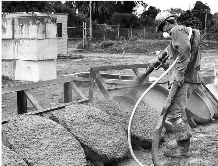
Figure 3-12: Manual Spraying of Shotcrete Panels (ASTM C1550 2010)
