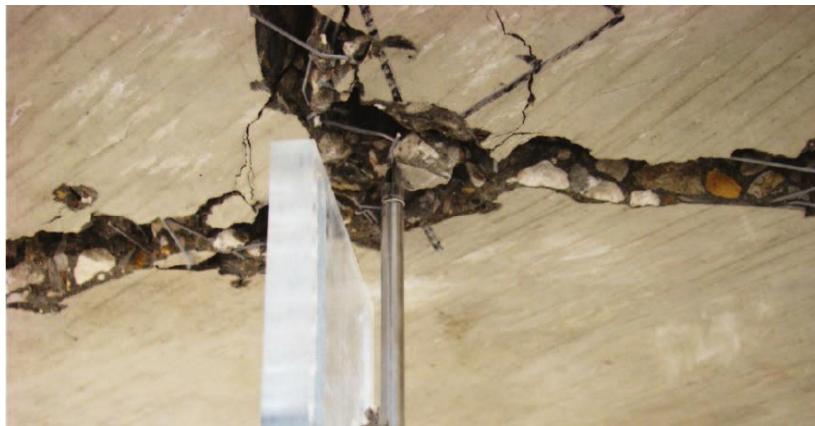
Figure 3-15: View of Underside of ASTM C1550 Test Specimen showing Crack Width vs. LVDT Probe Width at Location of LVDT (S.-H. Chao 2011)
