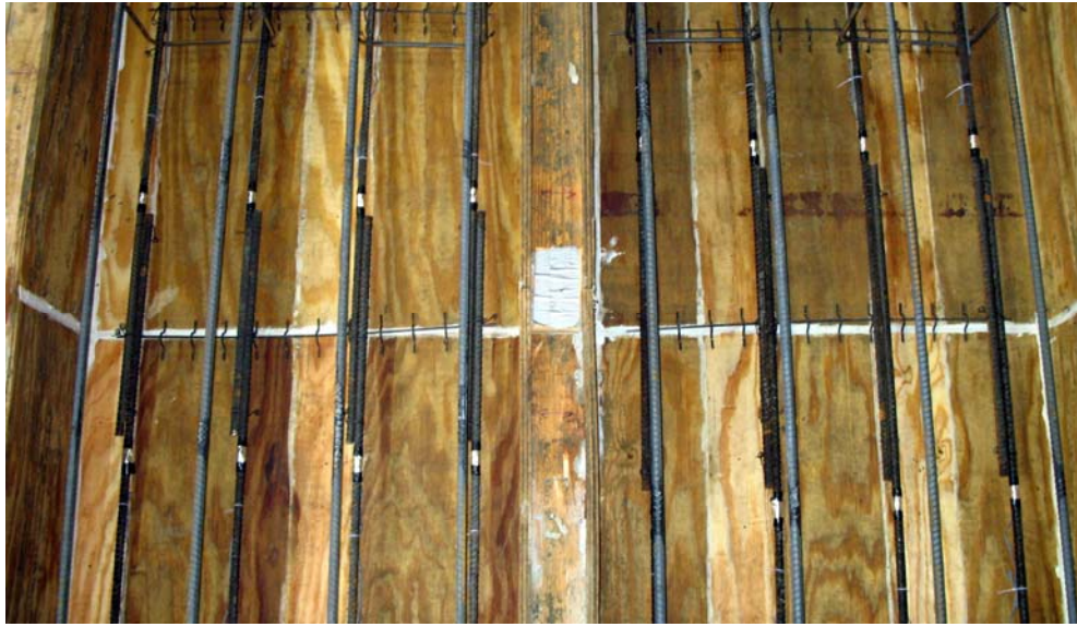
Figure 4-5: Varying splice length among a pair of specimens containing #5 bars
