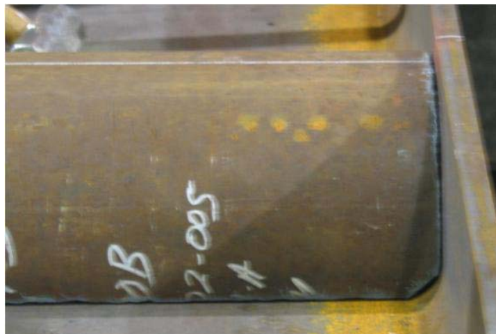
Figure 3.7 Half Pipe Stiffener Fabrication
