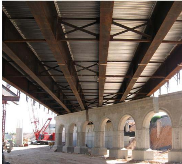
Figure 2.1 Skewed Steel Bridge
