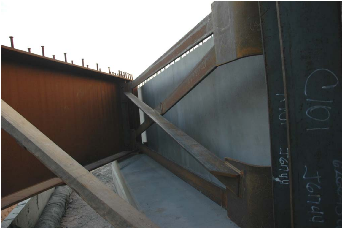
Figure 4.3 End Cross Frame
