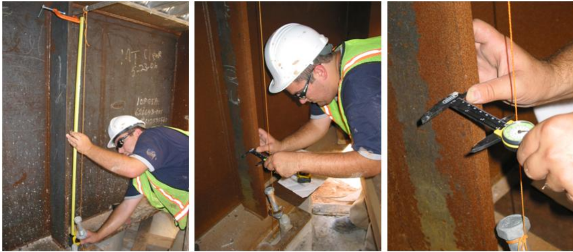
Figure 4.12 Measuring Twist at Girder Ends due to Concrete Deck Placement
