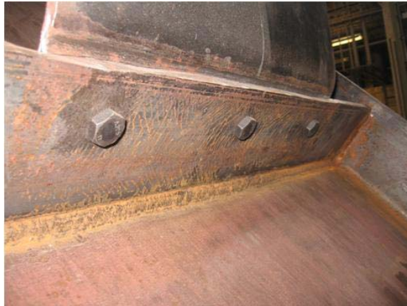
Figure 5.15 Bolted Bent Plate Connection
