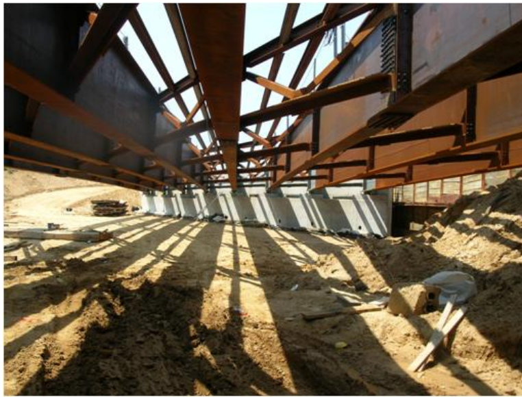
Figure 1.3 Churchman Road Bridge over Interstate 95 in Christiana, Delaware
