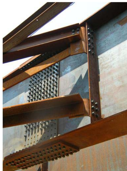
Figure 2.14 Installed Bent Plate Connection
