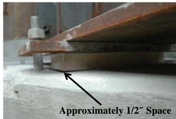
Figure 4.13 Fabreeka Bearing Pads
