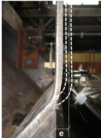
Figure 5.35 Increased Eccentricity to Connection due to Increased Bend Radius
