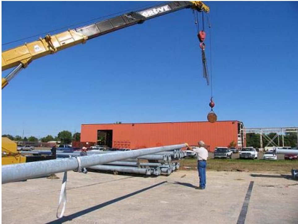
Figure 5.3.1.3 Crane Moving the 500-Pound Circular Weight to the Mast Arm End
