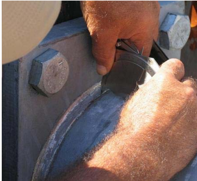
Figure 5.3.3.2 Measurement of UIT Application Groove Using an Undercut Measuring Device
