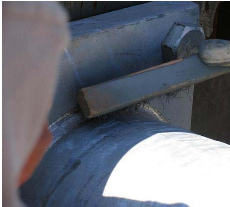
Figure 5.3.3.1 Removal of Galvanization with a Wire Brush
