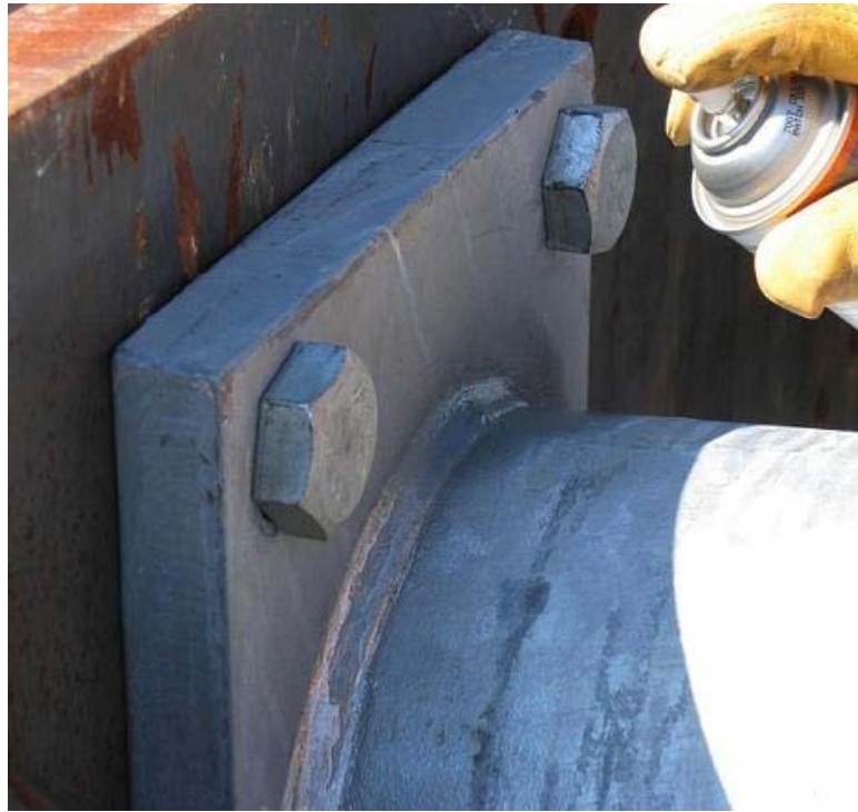
Figure 5.3.4.1 Application of Zinc-Rich Paint
