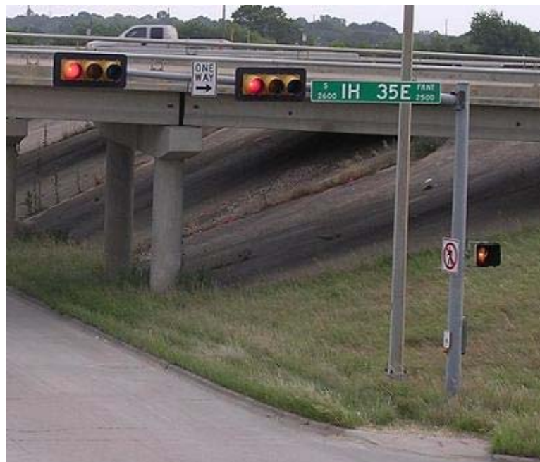
Figure 1.1.1 Typical Cantilever Traffic Signal Structure
