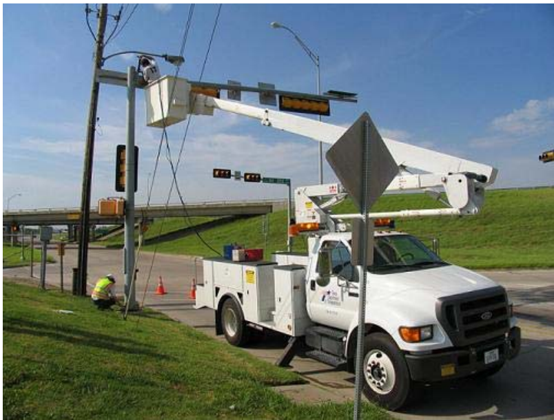
Figure 6.2.2 Mast Arm 1 on the Northeast Corner of the North Intersection of I-35E and Bonnie Brae St. in Denton, TX
