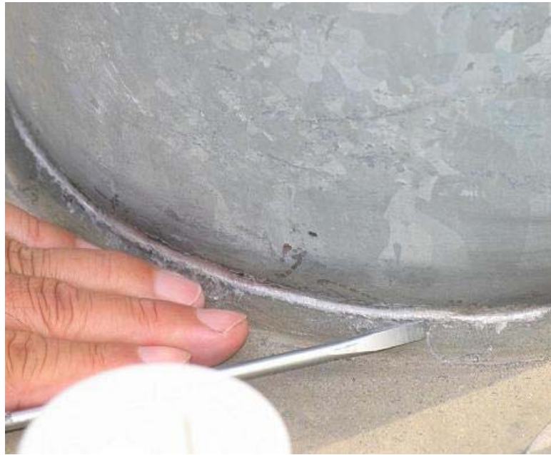
Figure 6.2.2.3 UIT Application at the bottom of Mast 2
