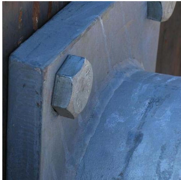
Figure 5.3.2.4 Mast Arm-Baseplate Weld Connection Before UIT Application
