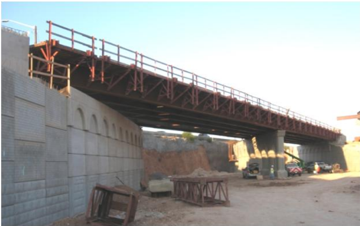
Figure 1.2: Skewed straight steel girder bridge
