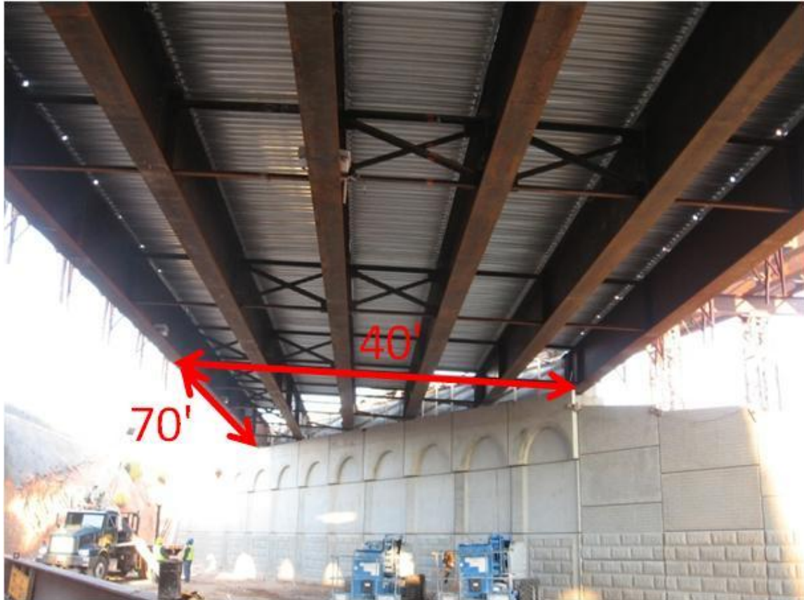
Figure 1.3: Skewed bridge support offset
