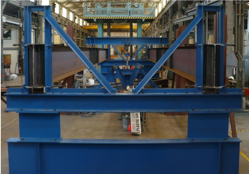
Figure 3.16: GBP1 and GBP2 in the twin girder buckling test frame (looking north)
