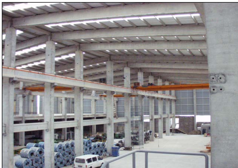
Figure 2.2 Interior Photograph of a Multi-story Precast Building
