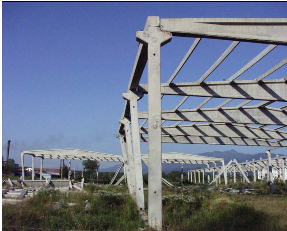
Figure 4.1 Large Transverse Drift Ratios
