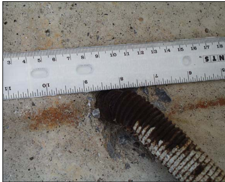
Figure 6.3 Threaded Dowels Used as Corbel Reinforcement
