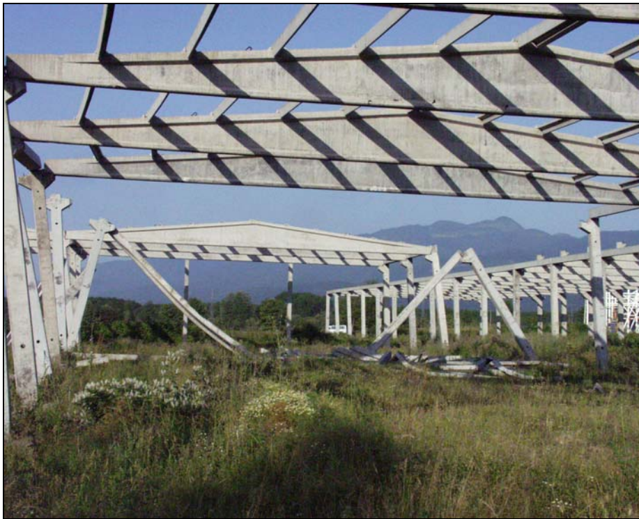
Figure 2.8 Large Drift Ratios Observed in Precast Buildings near Adapazari
