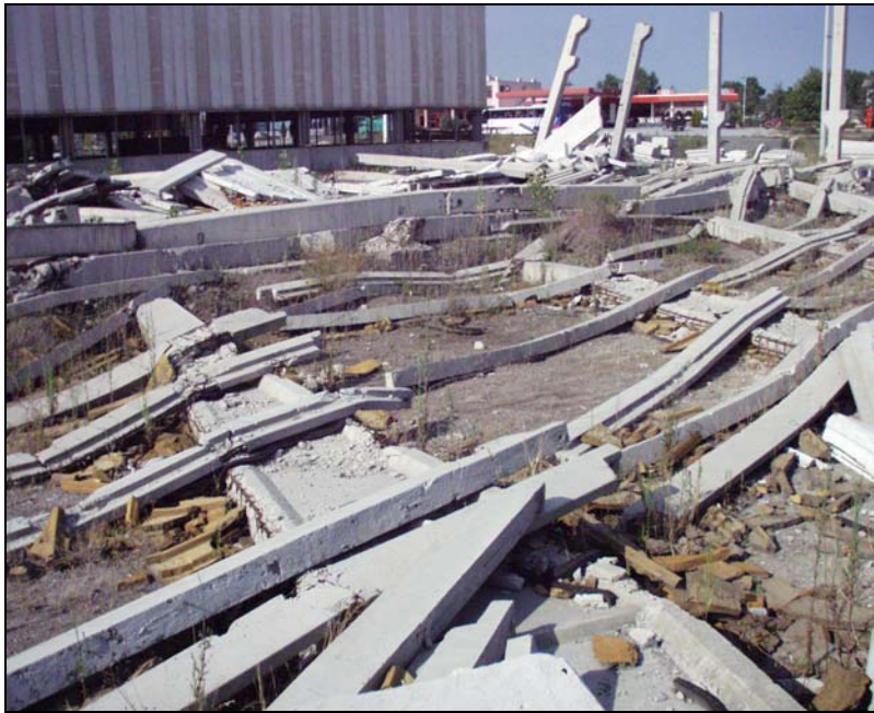
Figure 2.12 General Collapse of a Precast Building near Gölçük
