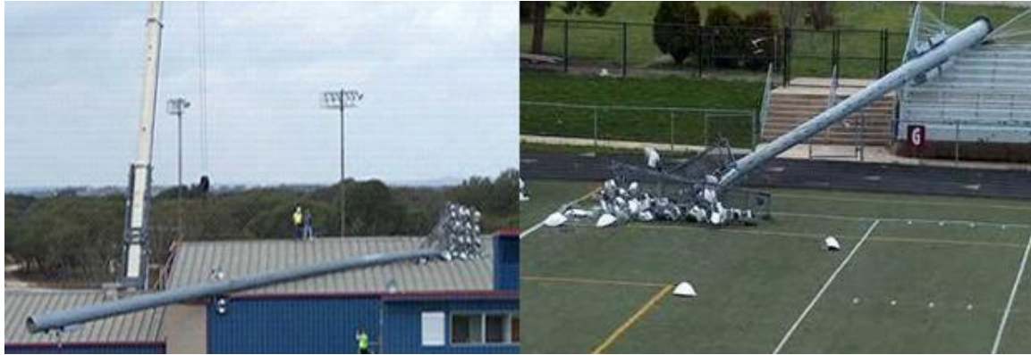
Fig.1.7. Collapse of a stadium sighting Pole over a gymnasium (Left), and in a practice field (Right) (CPSC website)
