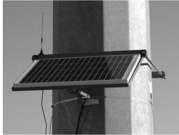
Fig. 3.7. Solar panel and wireless antenna mounted on a pole (El Paso, TX)
