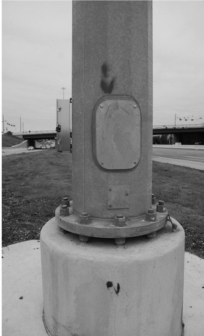
Fig. 3.2. Typical 12 Sided Pole instrumented (Austin, TX).
