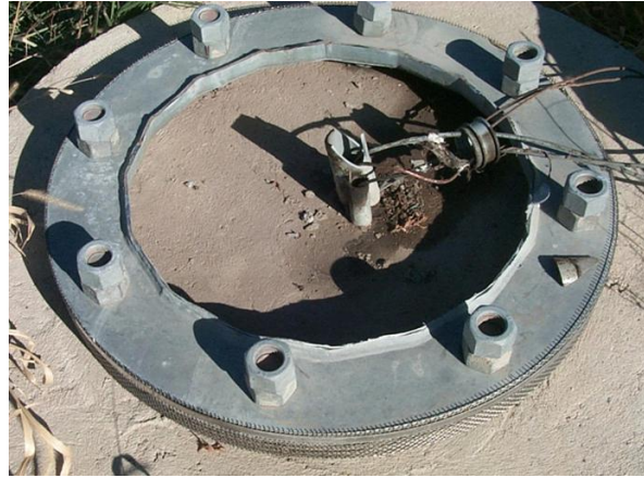
Fig. 1.5. Baseplate of the Collapsed HIMP in Sioux City, Iowa (Warpinski, 2007)
