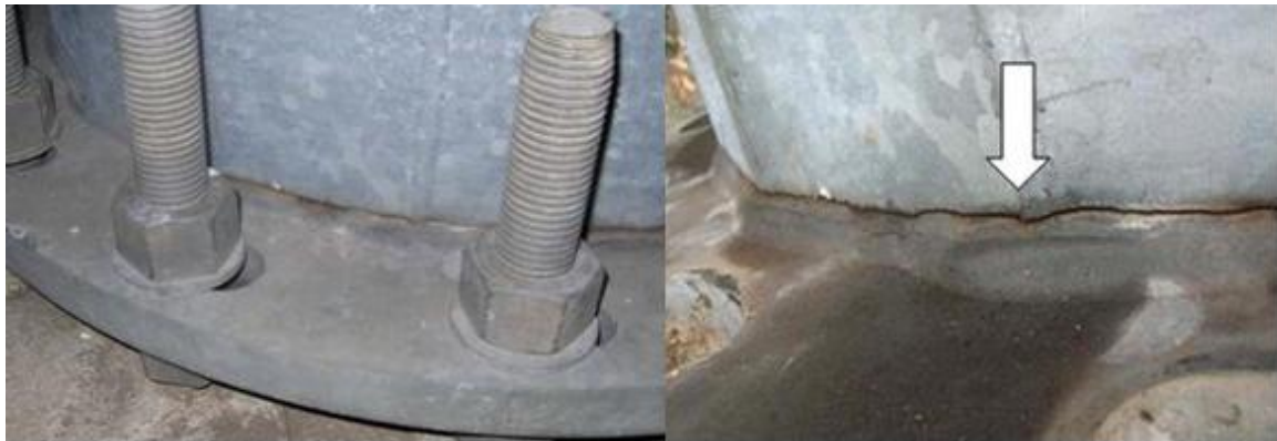
Fig.1.8. Cracks above the weld toe in stadium sighting poles (CPSC website)
