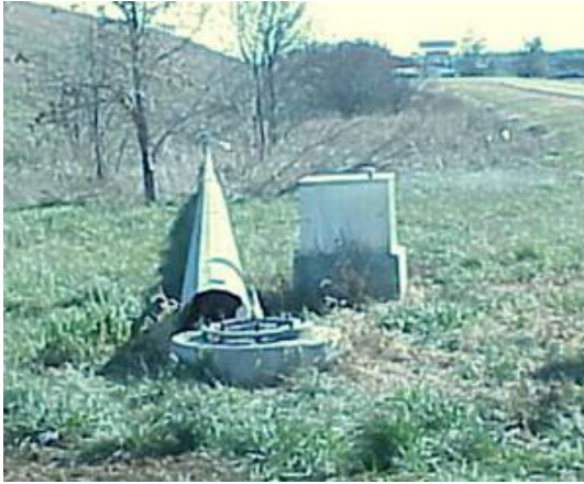
Fig. 1.4. HMIP collapse in Sioux City, Iowa (MTC, 2007)
