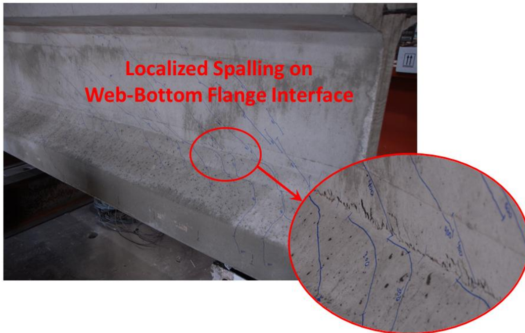
Figure 4-6: Signs of Horizontal Shear (Test 1-0.6-S) at 900 kips
