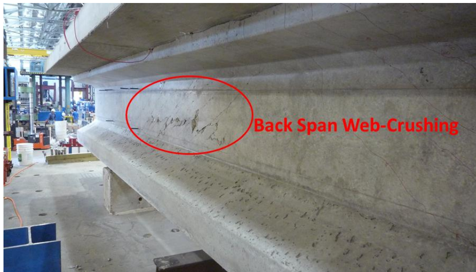
Figure 4-11: Back Span Web Crushing (Test 2-0.5-N)
