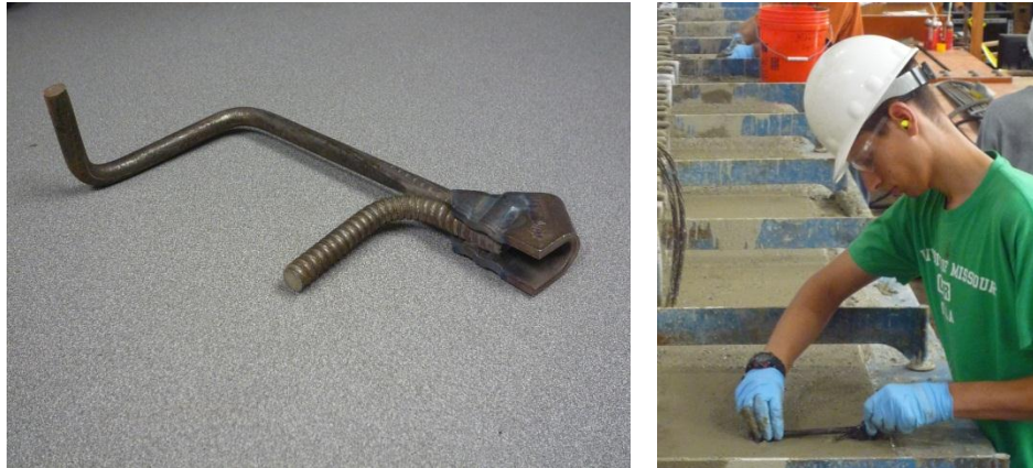
Figure 3-6: Sample Deck Anchor and Installing Deck Anchors
