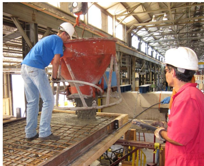
Figure 3-11: Placing Concrete for Deck
