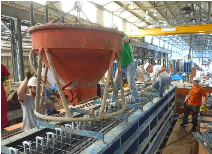
Figure 3-5: Placing Concrete for Tx46
