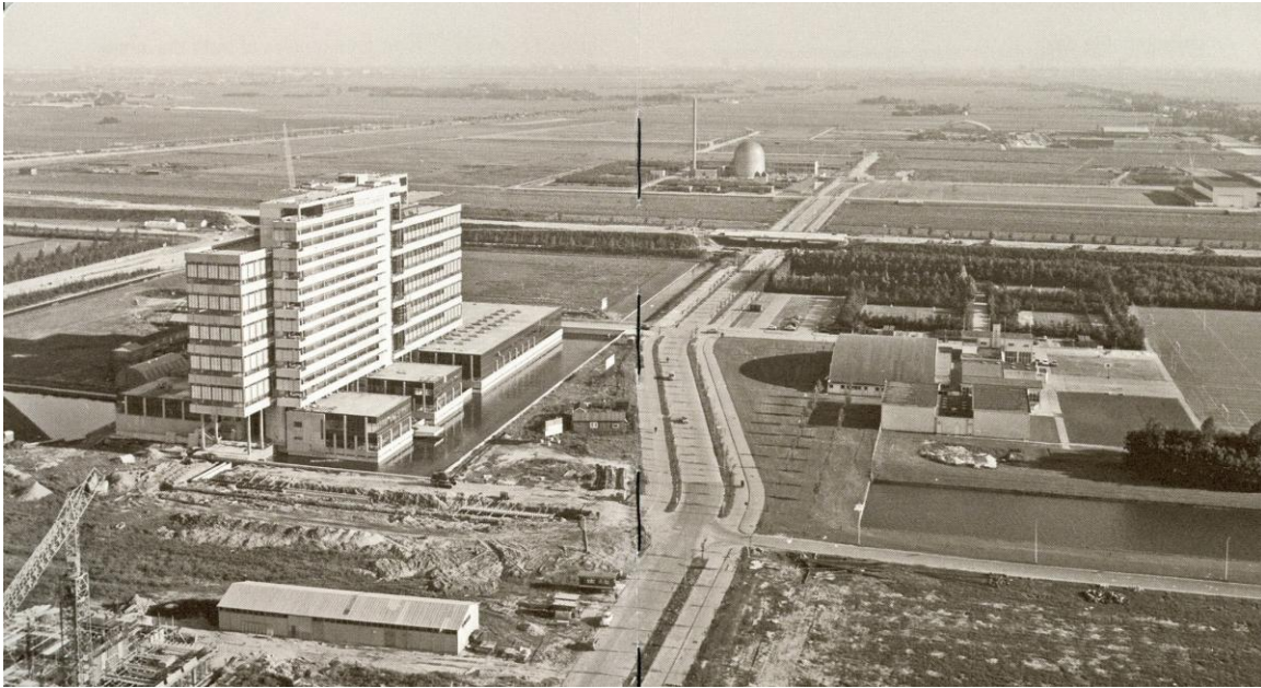
Figure 1.1 The FOA and Surroundings Shortly After Construction (TU Delft 2008)
