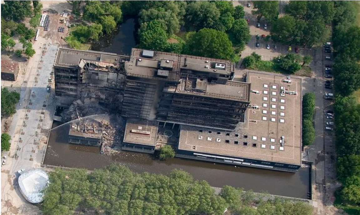
Figure 1.11 Aerial View of the Bouwkunde After the Collapse of the NW Wing
