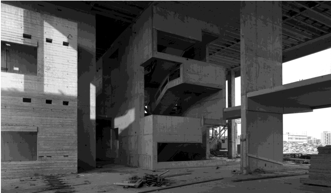
Figure 2.4 Stairwell and Wall During Construction
