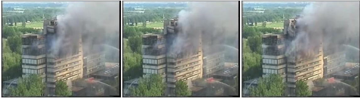
Figure 3.3 Photos of Collapse (note the rotation of the upper NW wing)
