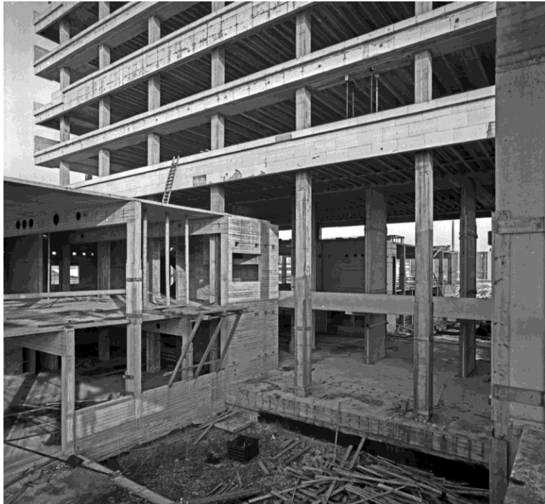
Figure 2.5 Columns and exterior girders during construction
