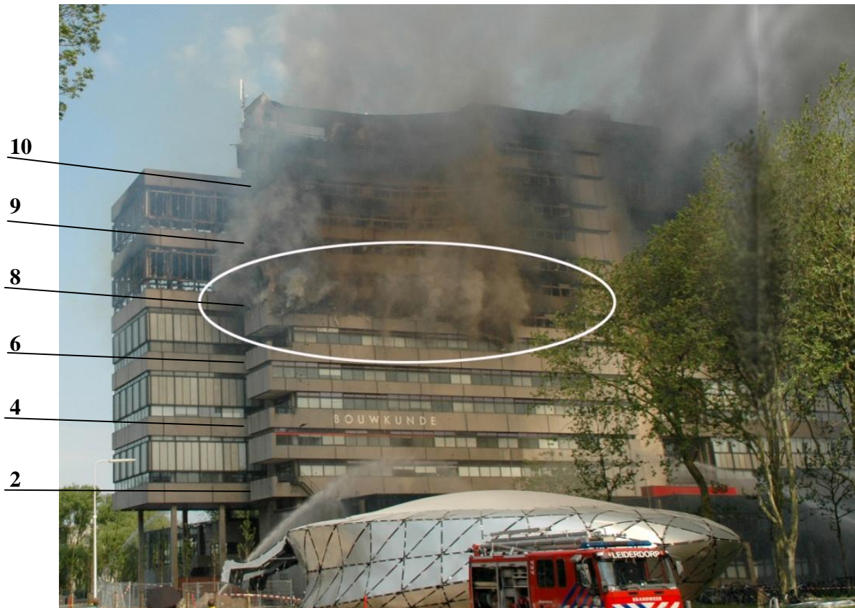
Figure 3.2 NW Wing at the Onset of Collapse (©Rob Jastrebski)
