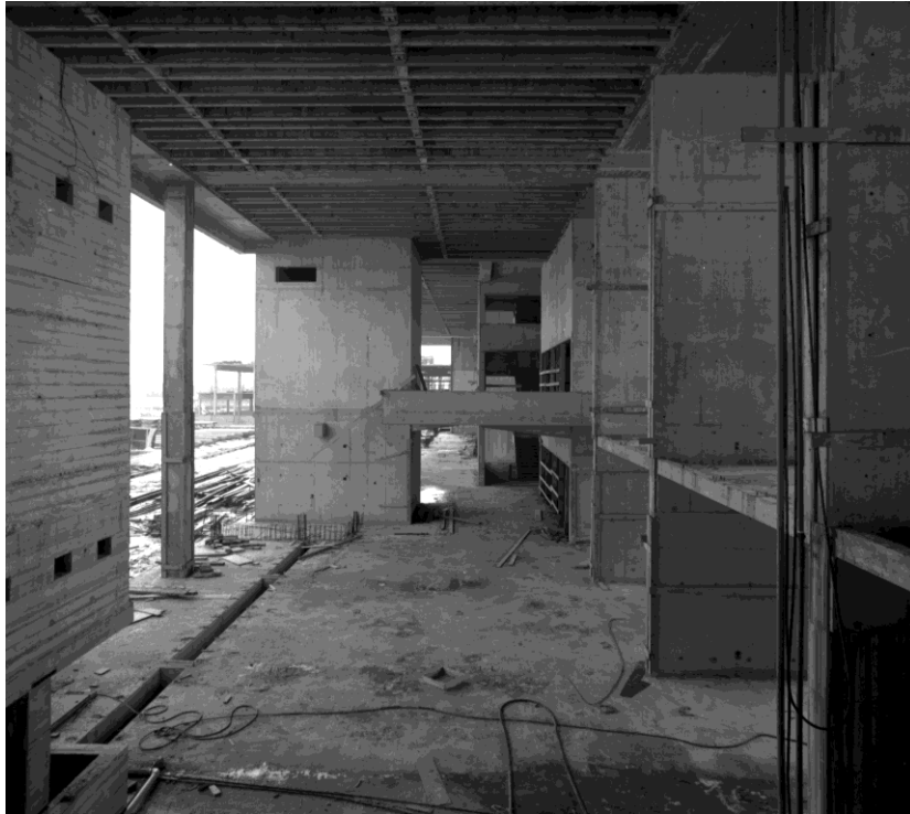
Figure 2.3 Walls and Joists During Construction
