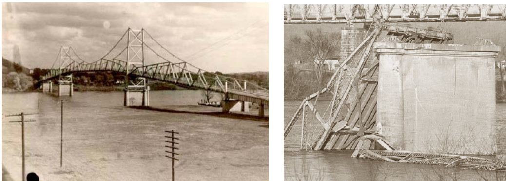
Figure 1.1: Silver Point Bridge Before and After Failure (Conner, Dexter, and Mahmoud, 2005)
