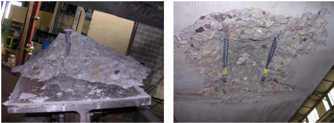
Figure 4.1: Failure Cone (a) Around Stud (b) Cone Void in Slab
