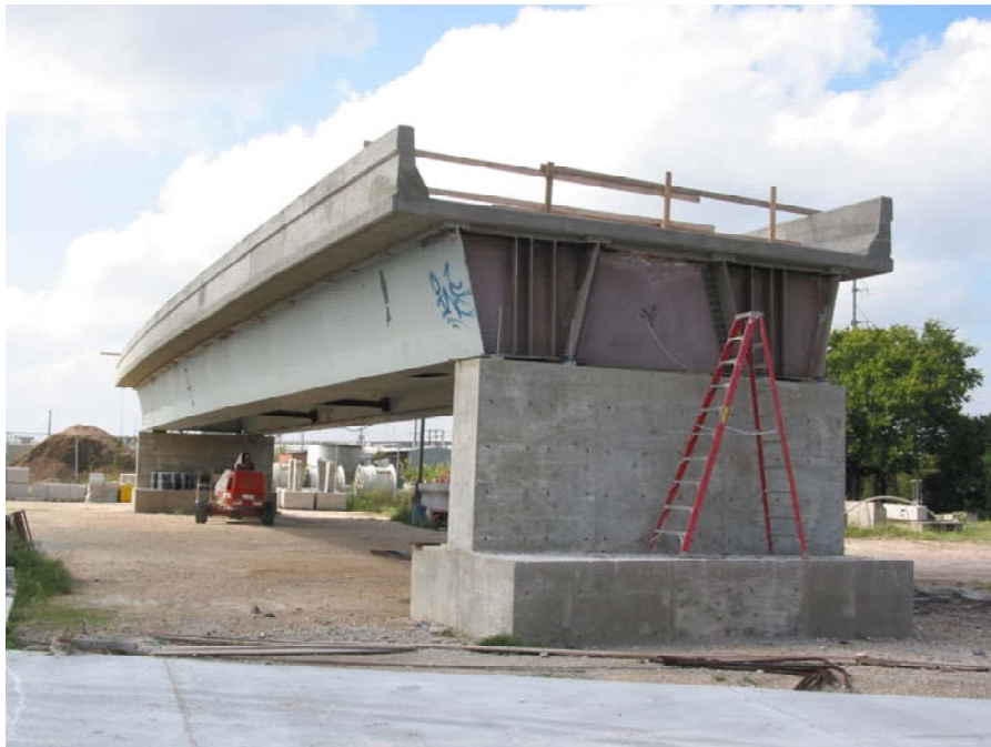
Figure 1.3(a): Picture of FSEL Test Bridge
