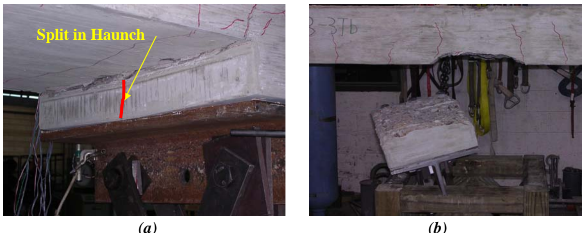
Figure 4.3: Series I Failures (a) Splitting of Haunch (b) Separation of Haunch
