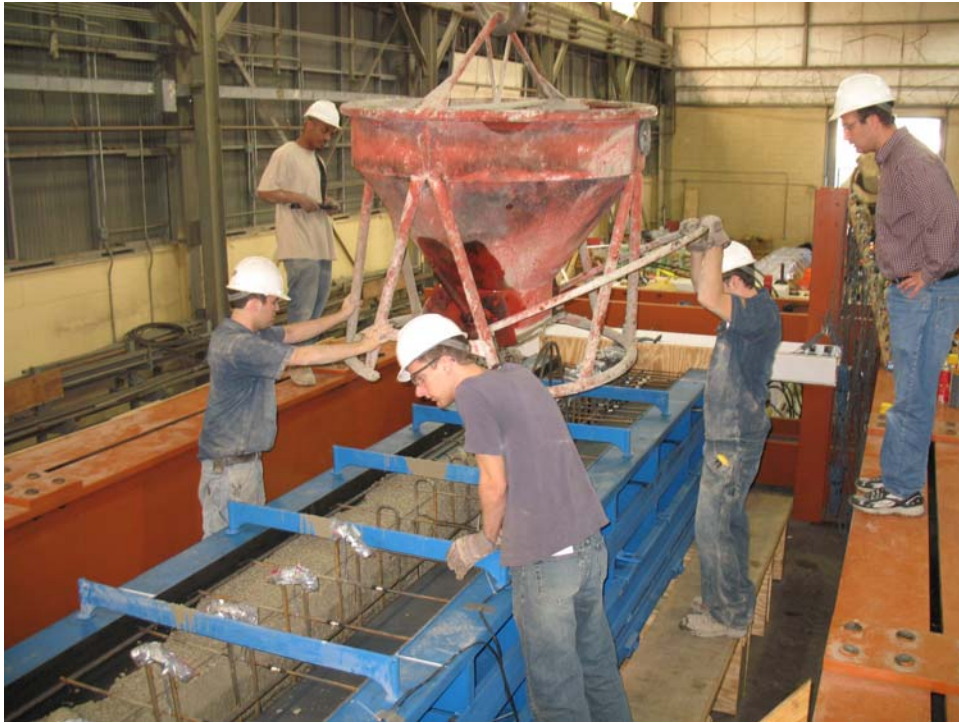
Figure 3- 13: Casting Operation for Tx Girder
