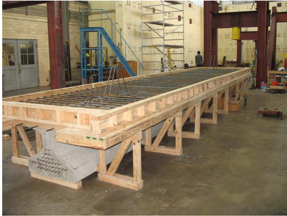
Figure 3- 18: Tx28 girder before casting of deck.
