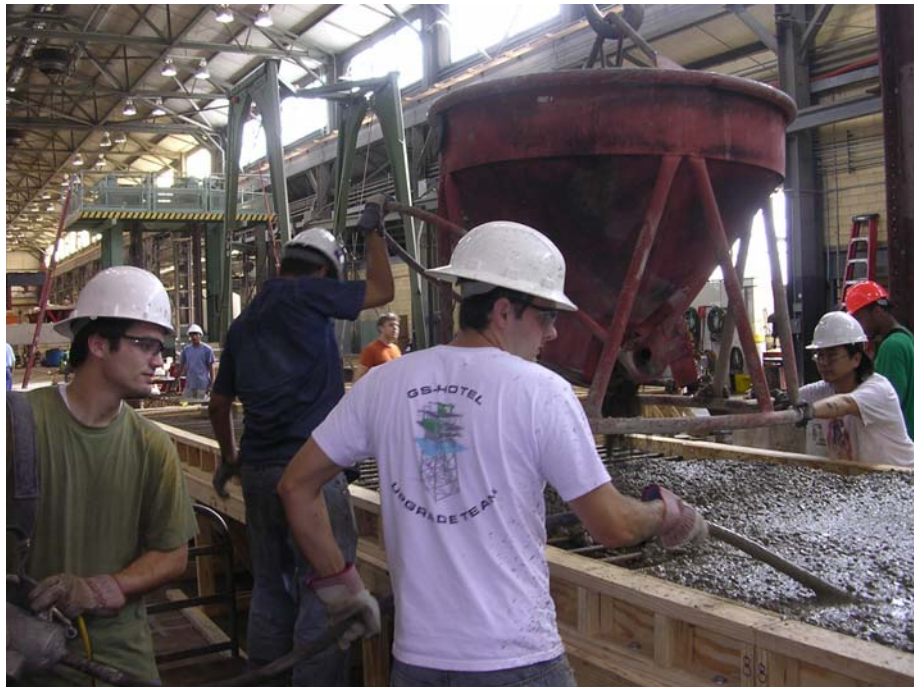
Figure 3- 19: Casting of composite concrete deck.
