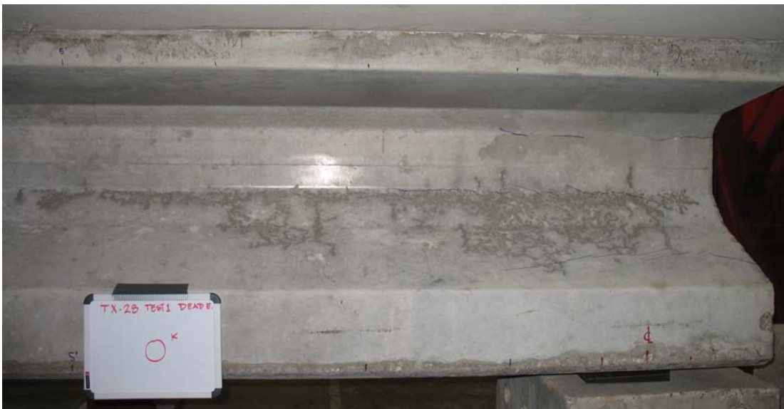
Figure 4- 18: Tx28-I dead end before Test 3.
