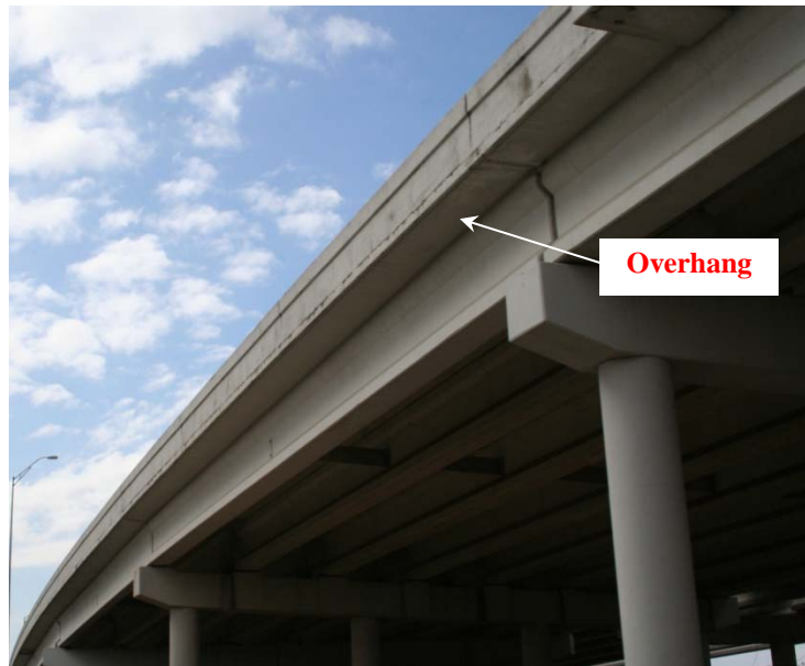
Figure 2-1: Bridge Deck Overhang on Texas I-beam bridge
