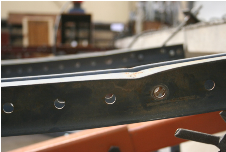
Figure 4-44: Buckled section of #4 C-49 overhang bracket on Tx-28-I
