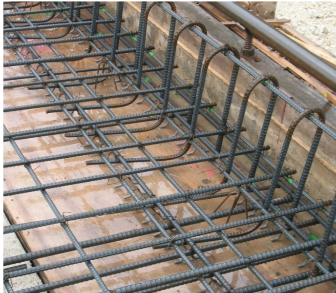
Figure 2-9: Mild steel reinforcing in bridge deck overhang
