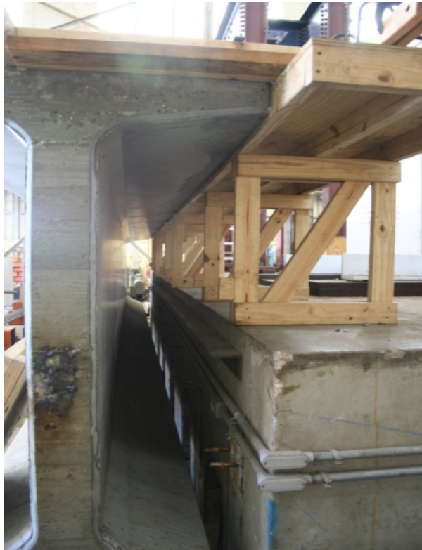
Figure 5-11: Tx-70 fascia girder placed next to overhang formwork
