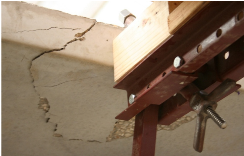
Figure 4-20: Underside of top flange of #4 HF-43-V on Tx-70 at failure zone
