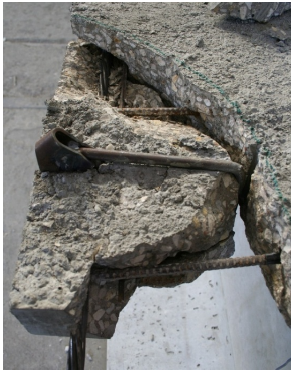
Figure 4-15: Punching shear/tensile failure of #1 HF-43 on Tx-46
