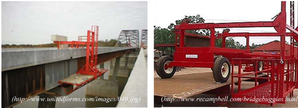
Figure 2-15: Examples of bridge overhang buggies
