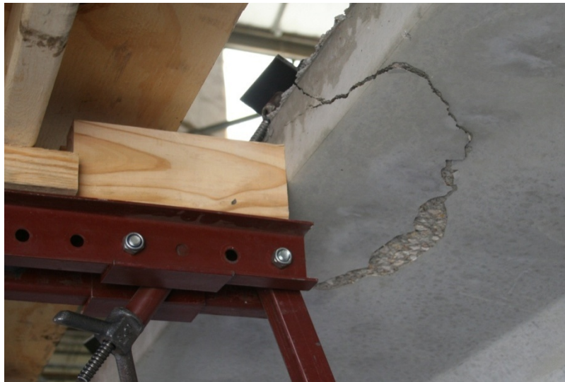
Figure 4-23: Underside of top flange of #4 HF-43-I on Tx-70 at failure zone
