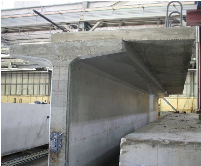
Figure 5-14: Finished precast overhang
