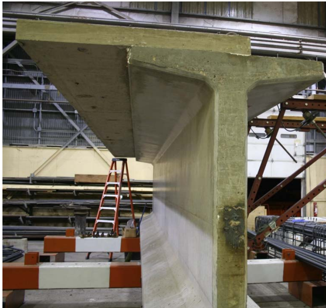
Figure 5-2: Precast overhang on Tx70 girder
