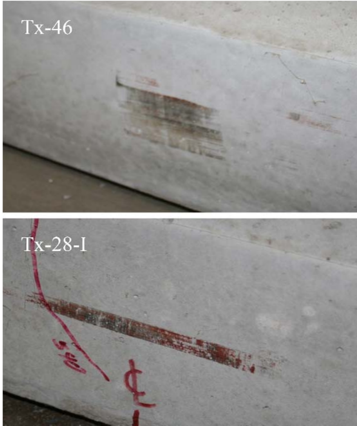
Figure 4-2: Rub marks on bottom flange due to friction
