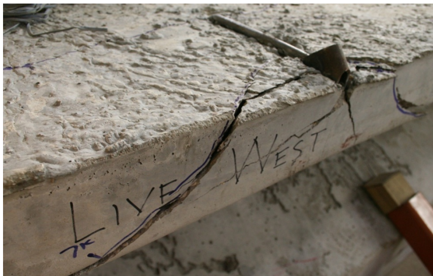
Figure 4-9: Punching shear failure at #2 HF-43 tip on Tx-28-I
