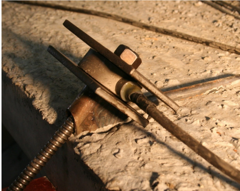
Figure 3-25: Position of pressure washer on hanger
