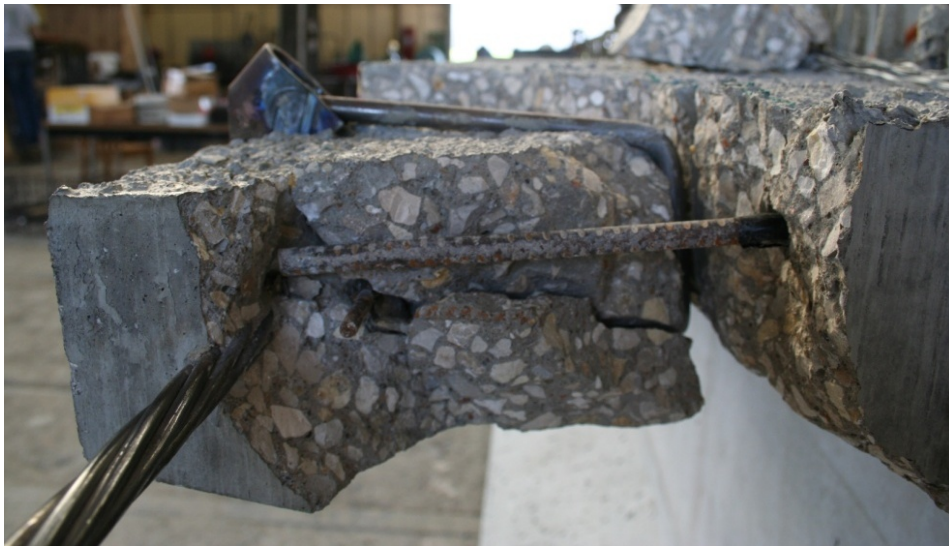
Figure 4-16: Side view of #1 HF-43 failure on Tx-46
