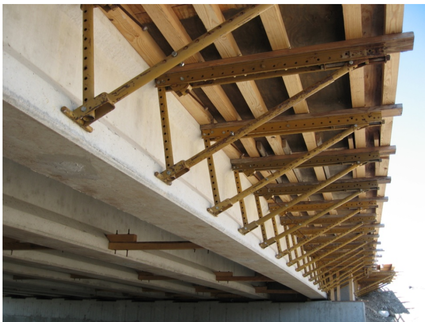
Figure 2-2: Bridge overhang brackets supporting formwork
