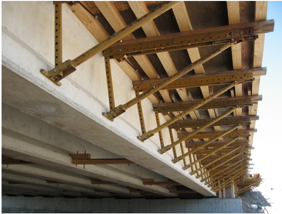
Figure 5-1: Currently used overhang forming system
