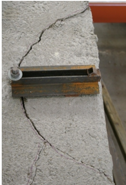
Figure 4-38: Failure of top flange at #1 HF-67-M on Tx-70 Test #1
