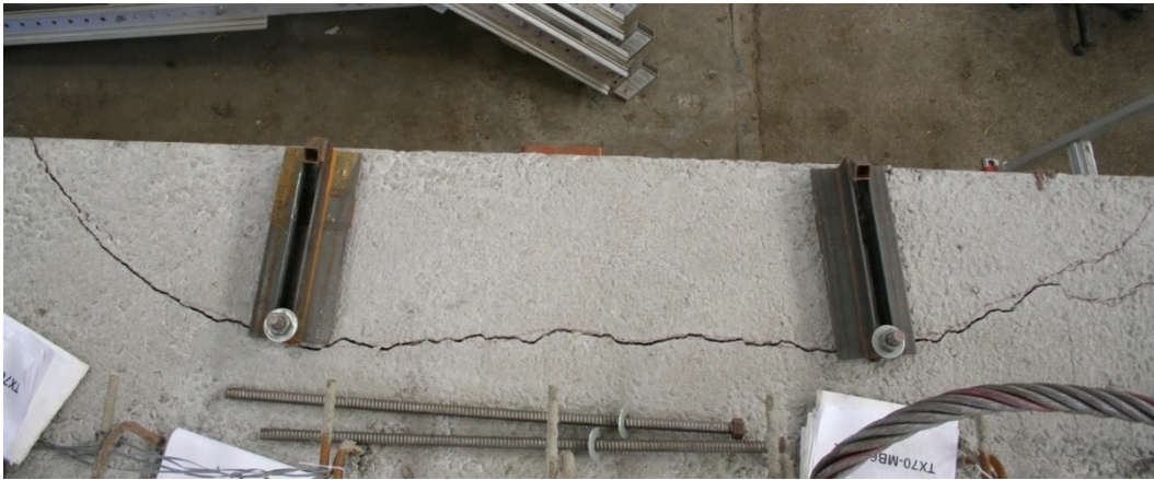
Figure 4-40: Failure perimeter around HF-67-M hanger #3 and #4 on Tx-70 Test 2
