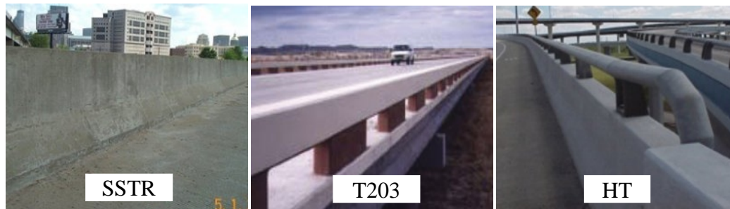
Figure 2-13: Bridge Rails in Texas (Bridge Rail Guide 2005)
