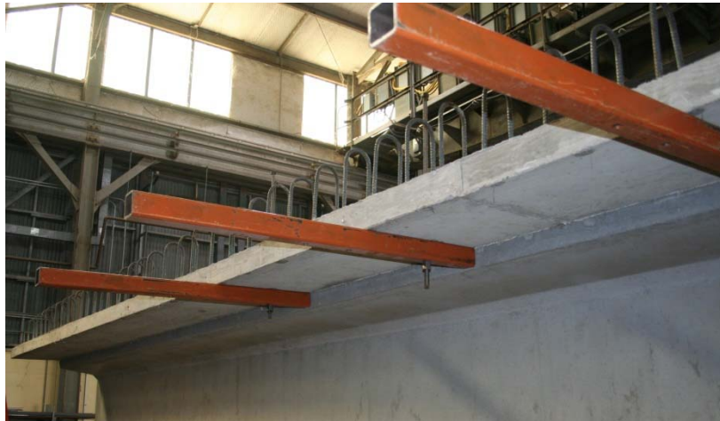
Figure 5-16: Support arms for work platform
