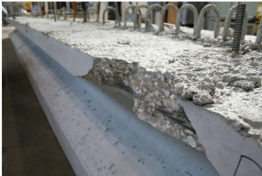
Figure 4-30: Punching shear failure at #1 HF-67 on Tx-28-II
