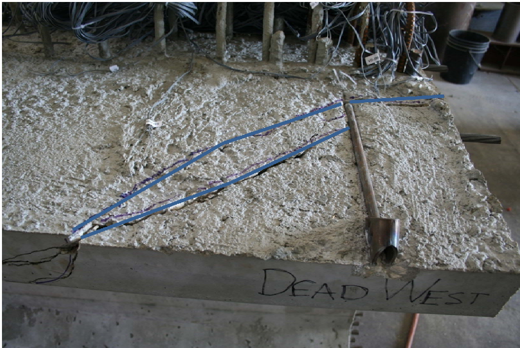
Figure 4-51: Punching shear/tensile failure at #4 C-24 Hanger on Tx-46
