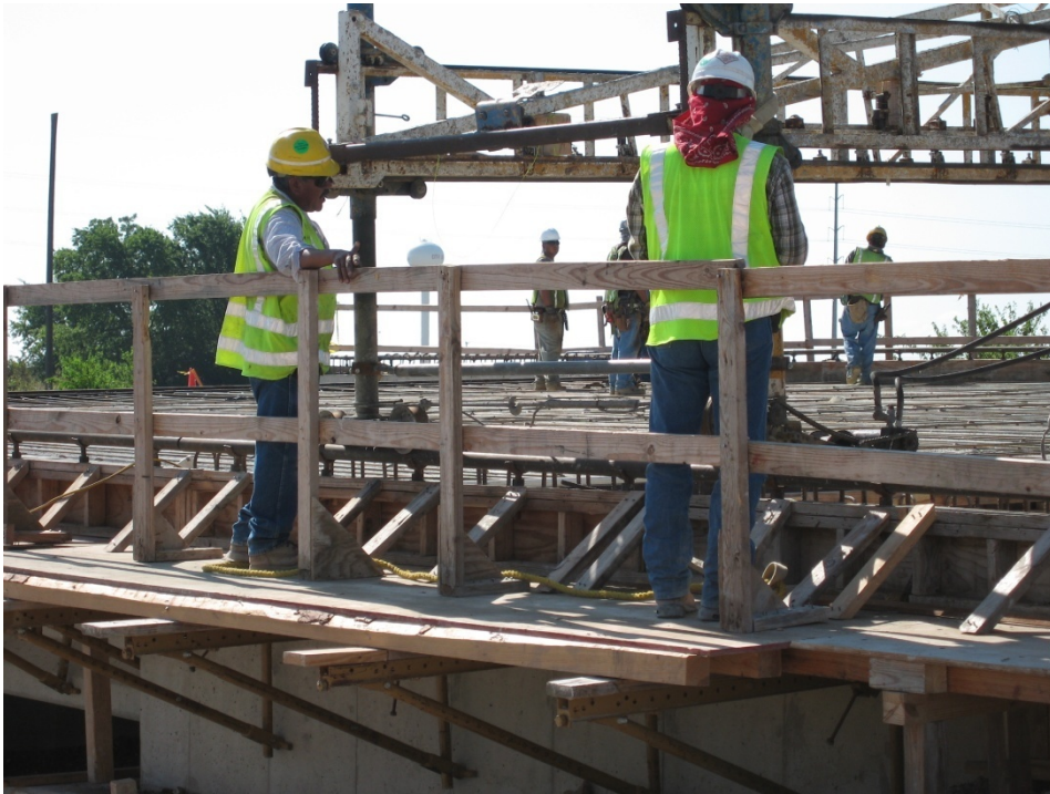
Figure 2-7: Work platform and safety rail
