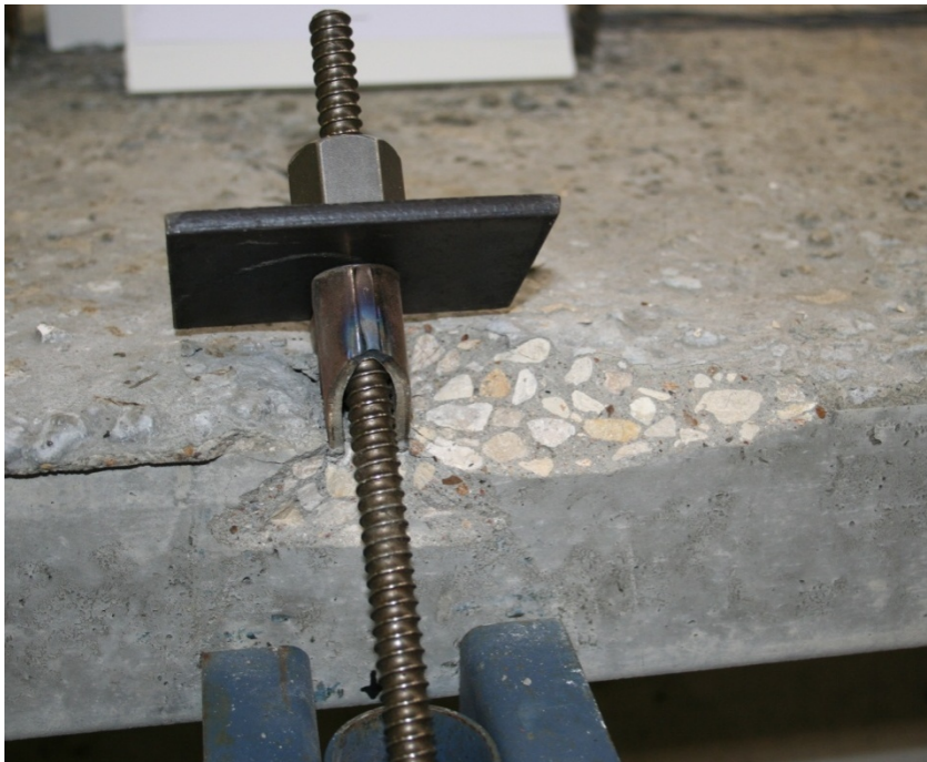
Figure 4-45: Spalling of concrete around #2 C-24 hanger on Tx-28-I
