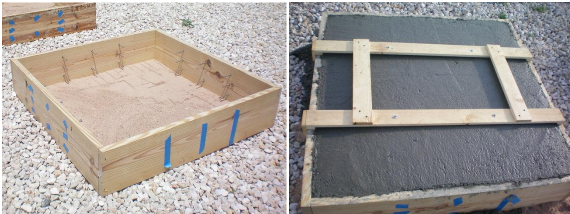
Figure 3.2: On-grade slab before (left) and after (right) concrete placement.
