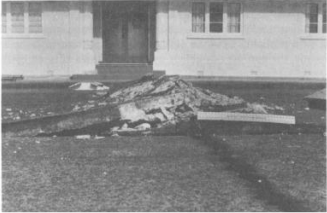
Figure 2.3: Crushing failure of pavement from ASR, from (Swamy 1992).
