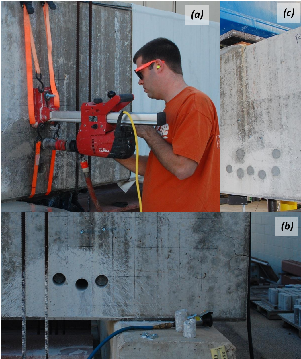
Figure 6.1: Extraction of 2 in. (51 mm) diameter cores from second reactive specimen and repaired core holes.
