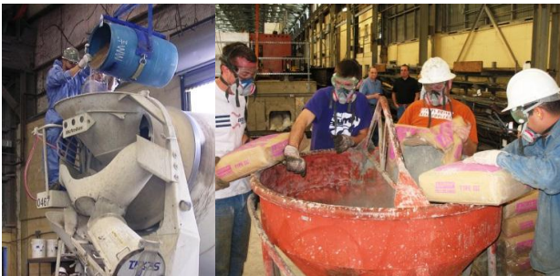
(c) Mix concrete
