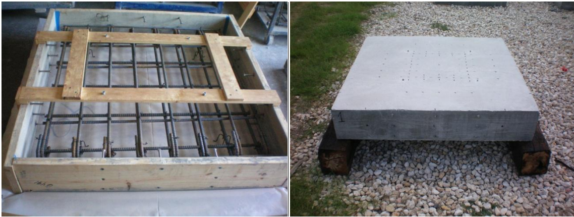
Figure 3.5: Bridge deck forms (left) and completed specimen on rail ties (right).
