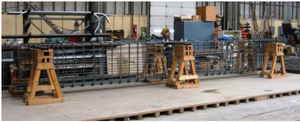
(a) Construct reinforcement cage
