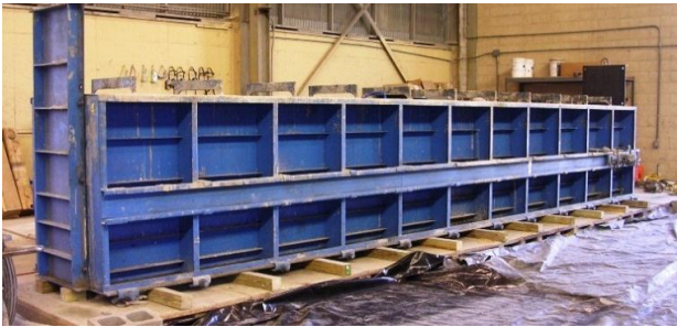
(b) Erect formwork, place cage inside
