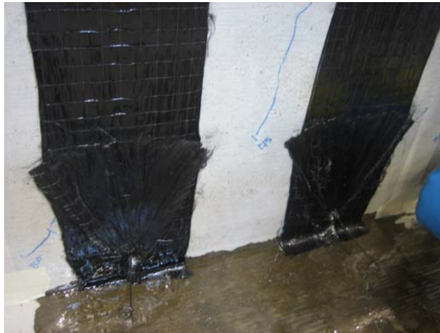
Figure 2-45 Completed installation of CFRP anchors
