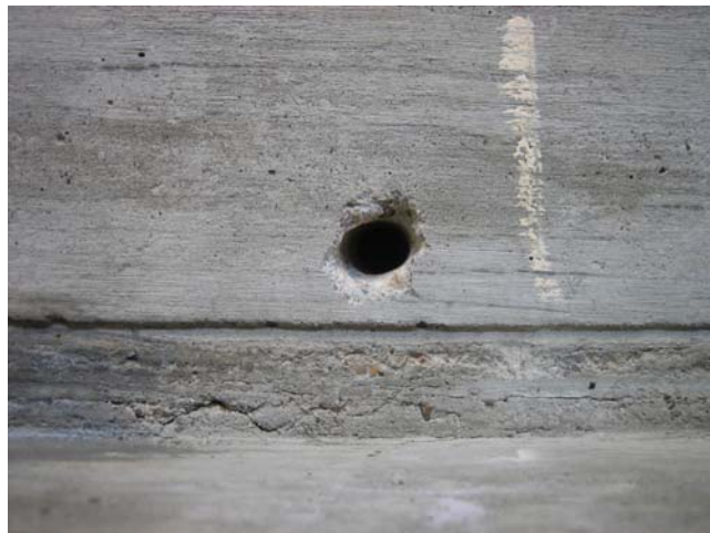
Figure 3-17 Drilled and cleared anchorage hole
