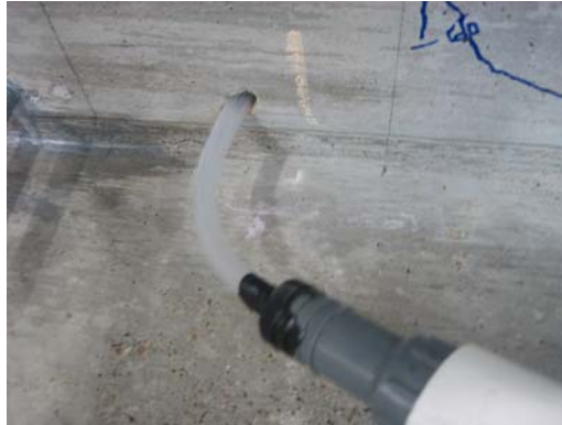
Figure 3-16 Removing debris from the anchorage hole
