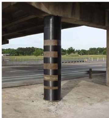
Figure 2-6 CFRP used in an axial confinement application (Yang, 2007)
