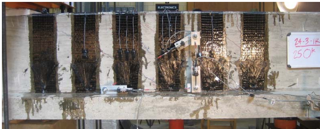
Figure 4-13 24-3-1R at 250-kips applied load (132-kips applied shear)
