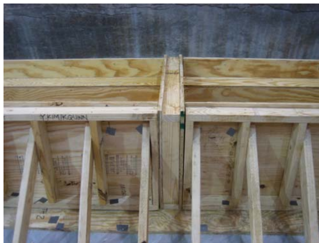
Figure 3-5 Lateral kicker braces and internal form divider
