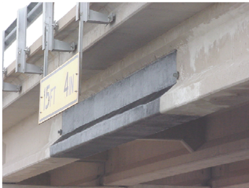
Figure 2-5 CFRP used in shear strengthening (Yang, 2007)
