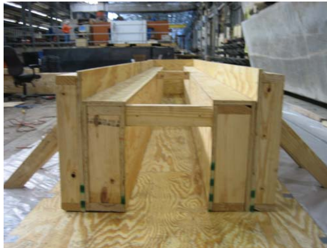
Figure 3-3 Cross section of wood formwork as constructed
