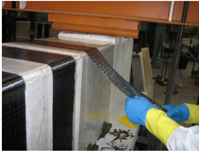
Figure 3-27 Aligning the free end of the installed CFRP strip
