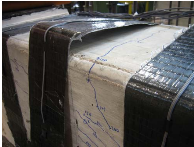
Figure 4-31 Failed CFRP strip observed during 24-3-3
