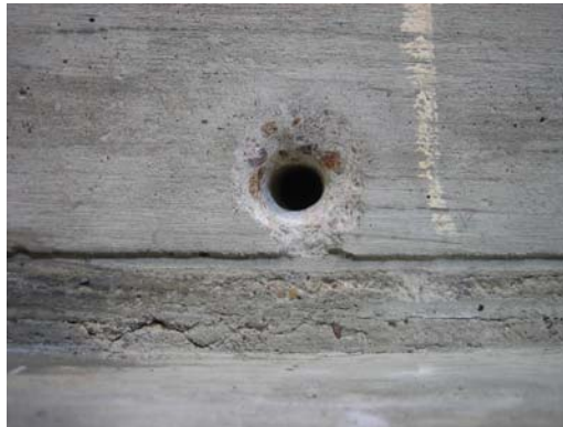
Figure 2-36 Anchor hole rounded with appropriate radius
