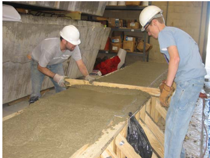
Figure 3-14 Screeding the top surface of the beams
