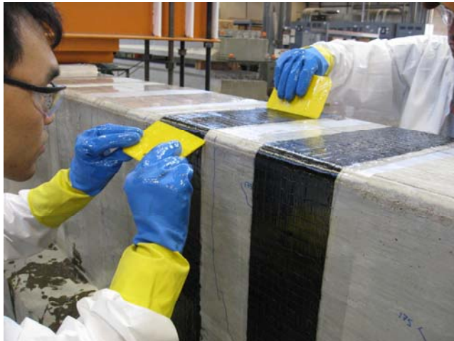
Figure 3-28 Removing excess epoxy from the installed CFRP strip
