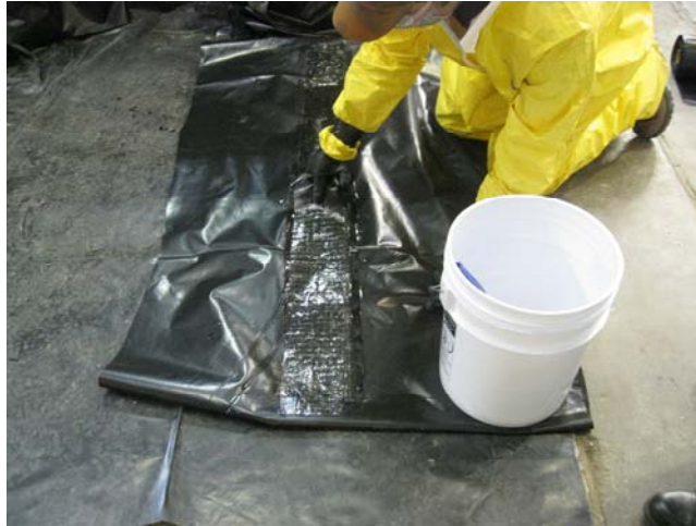
Figure 3-25 Folding the impregnated sheets in half for ease of handling
