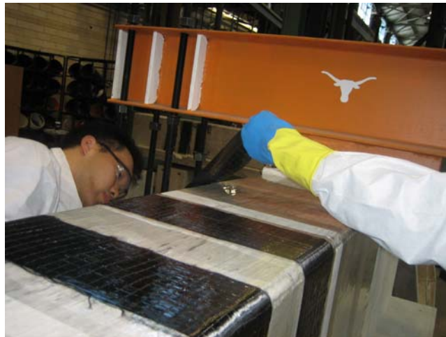
Figure 3-26 Placing the CFRP sheet onto the surface of the beam
