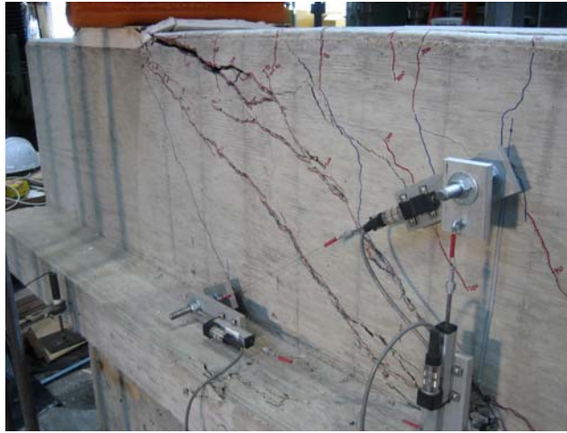
Figure 4-89 Cracking observed in 24-2.1-2
