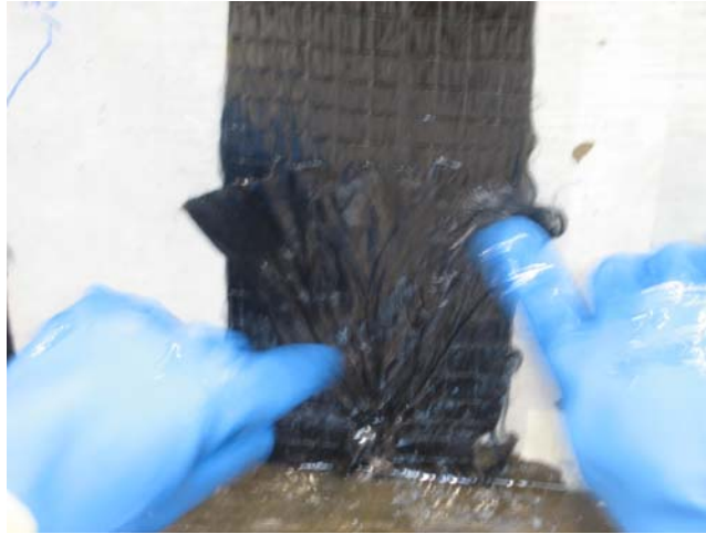
Figure 2-44 Construction of CFRP anchorage fan
