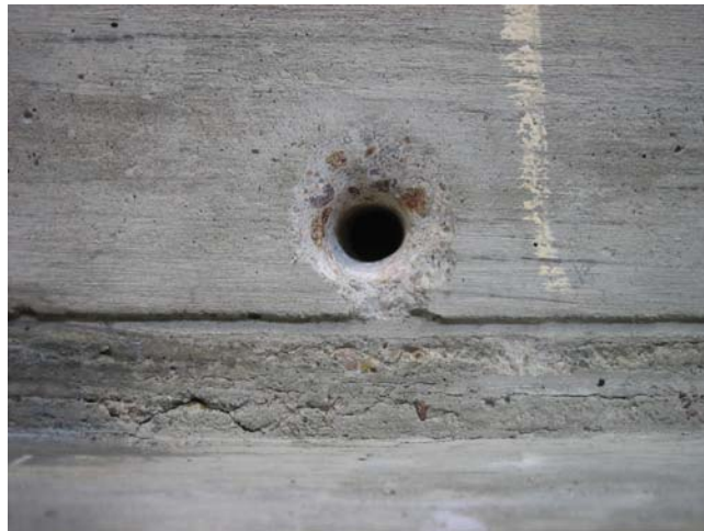
Figure 3-18 Completed preparation of CFRP anchorage hole
