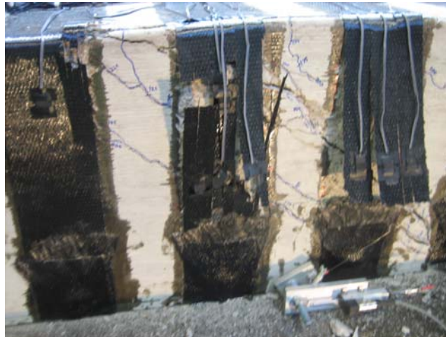
Figure 4-53 Rupture of CFRP strips, test 24-3-5
