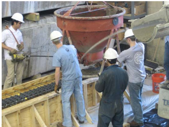
Figure 3-12 Placing concrete within the formwork
