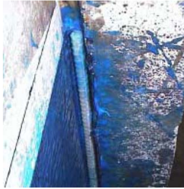
Figure 2-25 Glass FRP rod used to anchor a CFRP sheet a concrete beam (Khalifa, Alkhrdaji, Nanni, & Lansburg, 1999)
