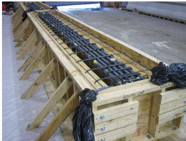
Figure 3-10 A completed reinforcing cage with slab reinforcement installed
