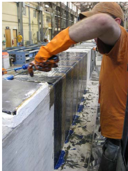
Figure 3-35 Impregnating the CFRP strip while on the surface of the beam
