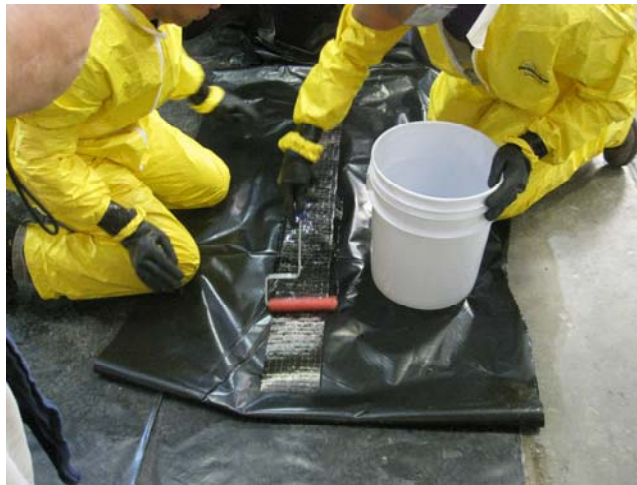
Figure 3-24 Impregnating the carbon fiber sheets with epoxy
