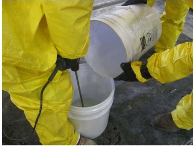
Figure 3-20 Mixing the two components of the epoxy together
