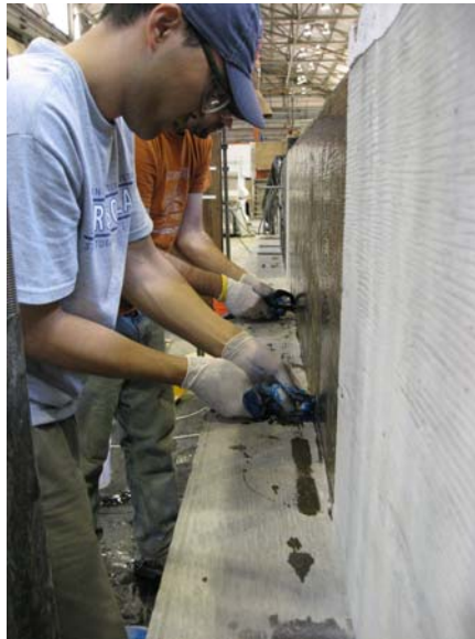
Figure 3-33 Wetting the surface of the CFRP anchor holes
