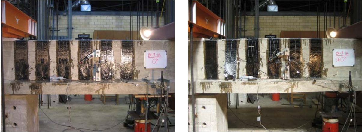
Figure 4-5 24-3-1R before (left) and after (right) loading
