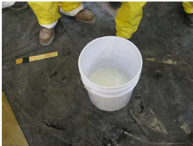
Figure 3-21 Completed high strength structural epoxy
