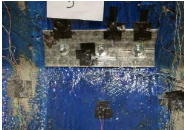
Figure 2-31 A CFRP strip that has slipped out of the discontinuous anchorage (Ortega, Belarbi, & Bae, 2009)
