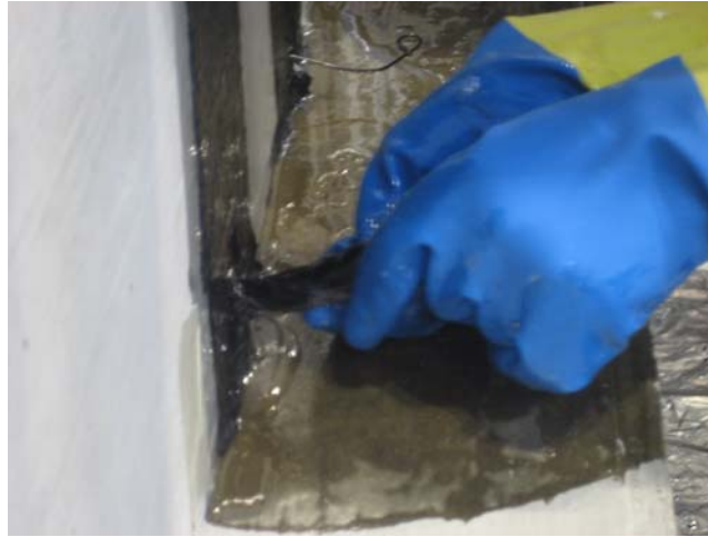
Figure 2-42 Insertion of the CFRP anchor
