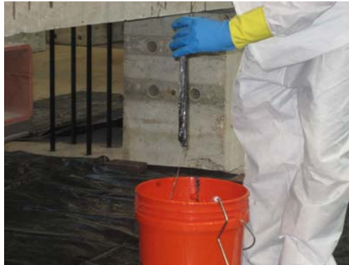
Figure 2-41 Impregnation of the CFRP anchor with high strength structural epoxy
