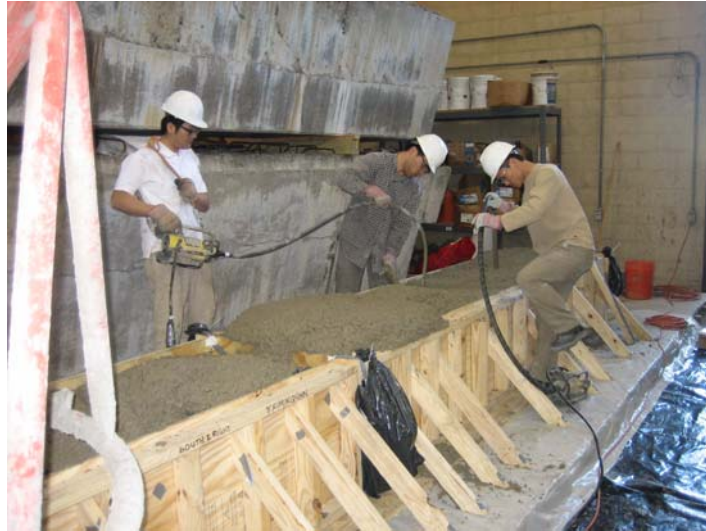
Figure 3-13 Vibrating the concrete
