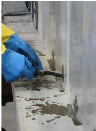
Figure 3-23 Wetting the drilled anchor hole with epoxy
