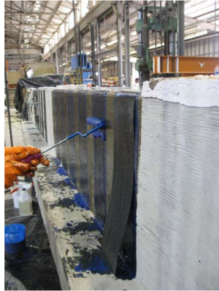
Figure 3-36 Sealing the CFRP laminates with epoxy
