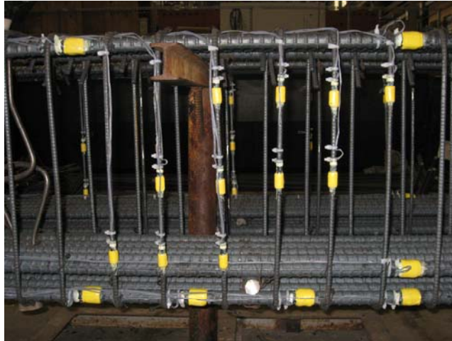
Figure 3-58 Rubber pads served as mechanical protection for the gauges
