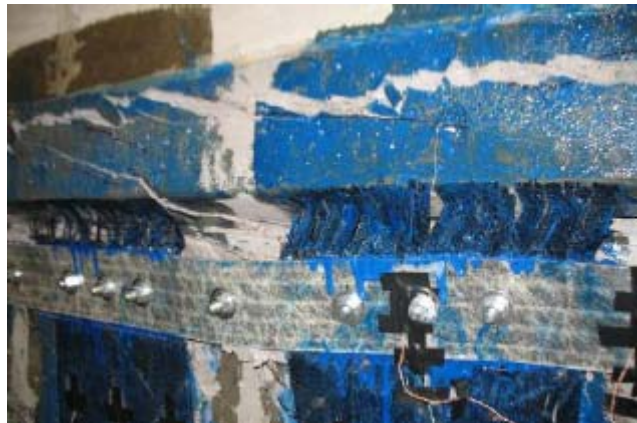
Figure 2-28 Buckling of the continuous CFRP plate observed at failure (Ortega, Belarbi, & Bae, 2009)
