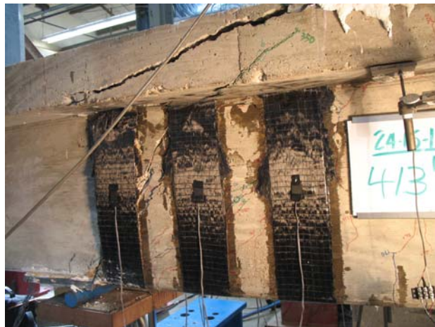
Figure 4-102 Observed failure of 24-1.5-1R2 (east side)
