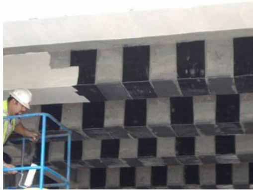
Figure 2-4 CFRP used in flexural strengthening (Yang, 2007)
