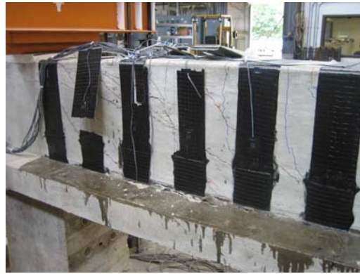
Figure 4-41 Rupture of CFRP strips, test 24-3-4
