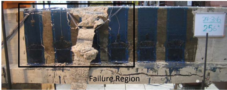
Figure 4-72 Failure region of 24-3-6
