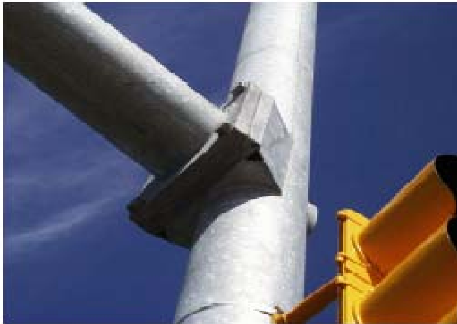
Figure 2.1 Typical Mast Arm Built-Up-Box Connection detail
