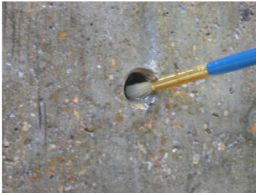
Figure B.2.10 Saturate the holes with the epoxy resin
