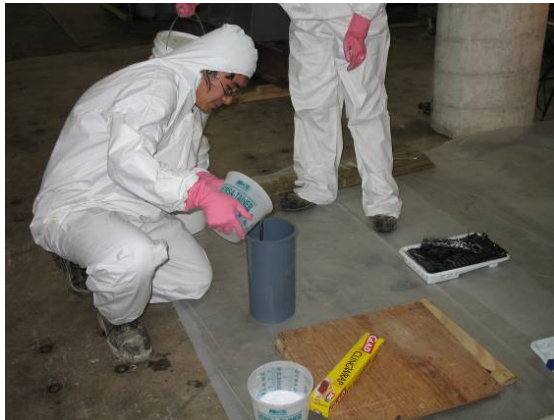
Figure 3.23 Prepare epoxy resin
