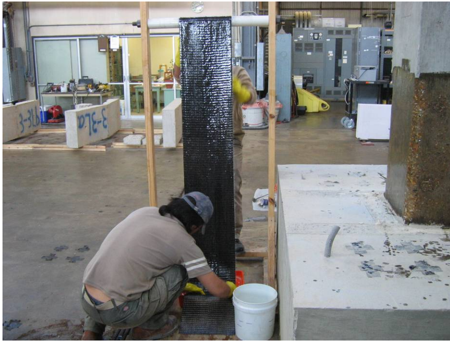
Figure B.2.11 Saturate CFRP jackets with the epoxy resin
