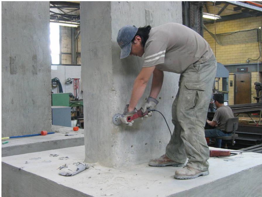
Figure B.2.4 Grind to round the corners
