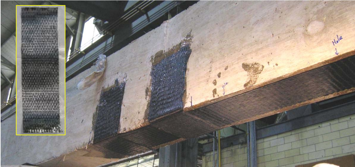
Figure 2.8 CFRP U-wrap
