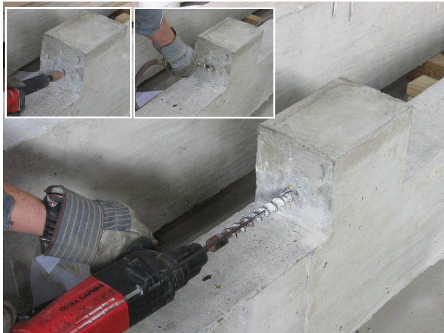
Figure 3.21 Preparation of a hole for connection sheet
