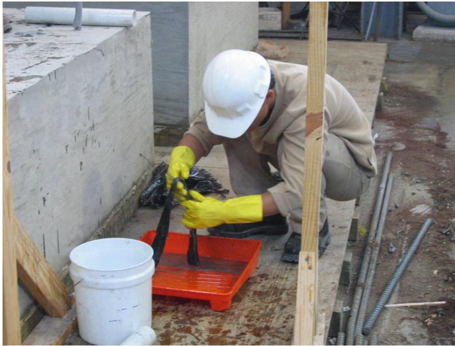
Figure B.2.15 Saturate CFRP anchors with the epoxy resin
