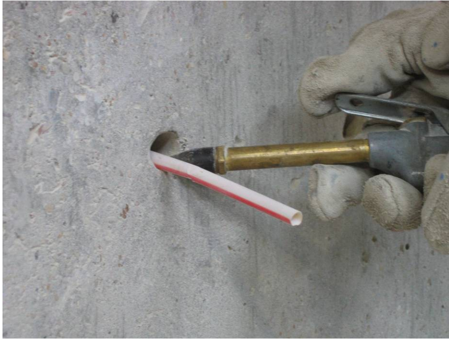
Figure B.2.5 Clean the holes with air compressed
