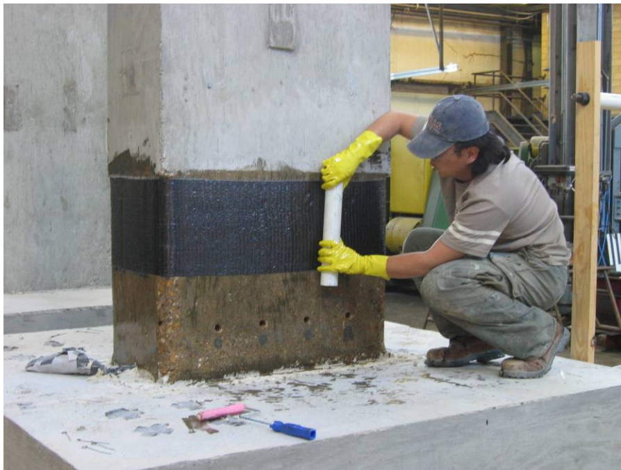
Figure B.2.14 Place the CFRP jackets on the column
