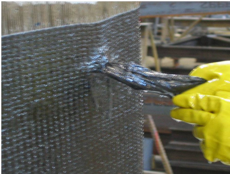
Figure B.2.16 Place the CFRP anchors on the column
