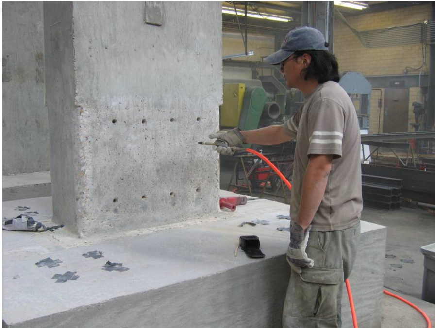
Figure B.2.6 Clean the surfaces with air compressed
