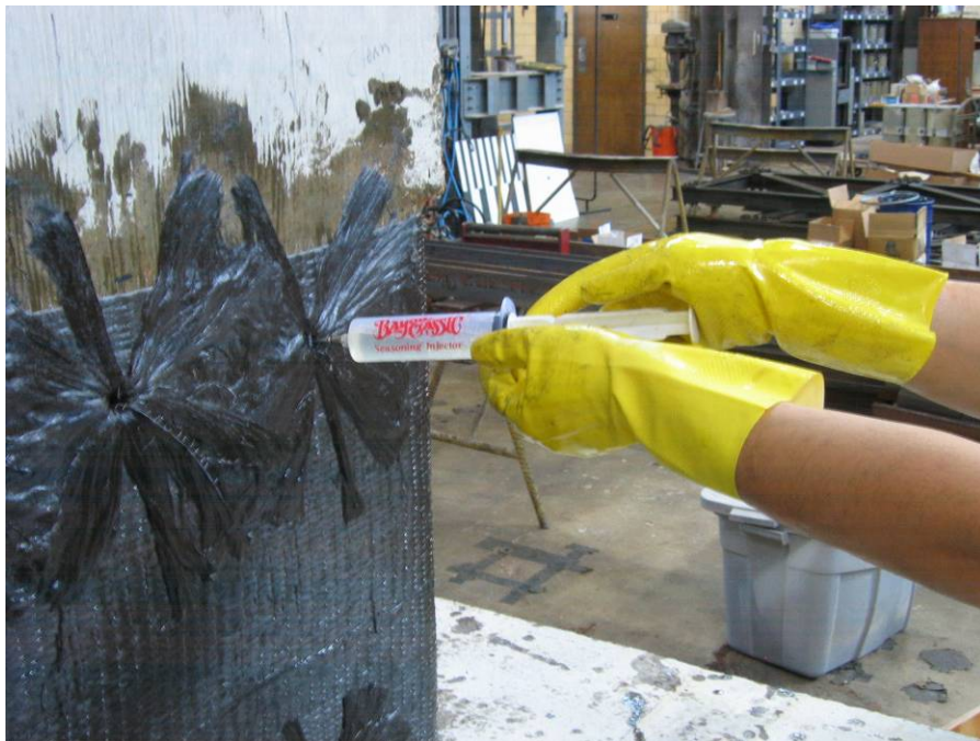
Figure B.2.18 Inject epoxy to fill all voids in anchor hole
