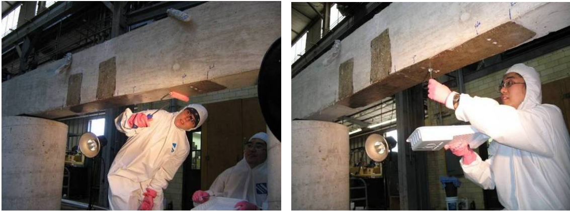
Figure 3.24 Saturate the concrete surface and holes with the epoxy resin
