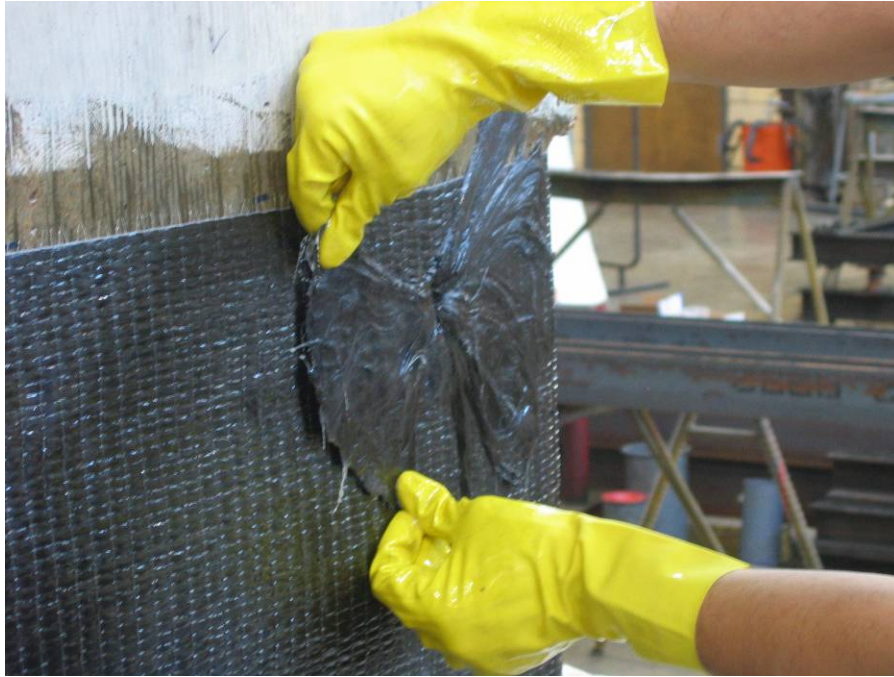
Figure B.2.17 Place the CFRP anchors on the column
