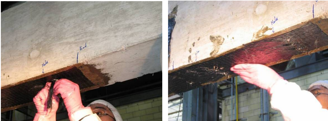
Figure 3.28 Saturate and place the CFRP anchors
