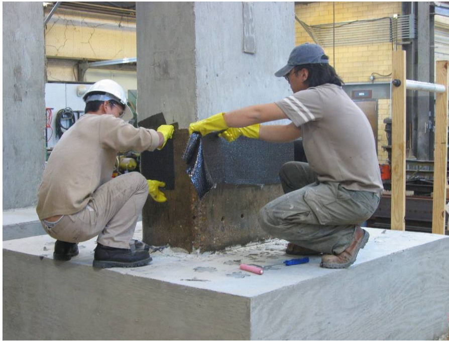
Figure B.2.13 Place the CFRP jackets on the column
