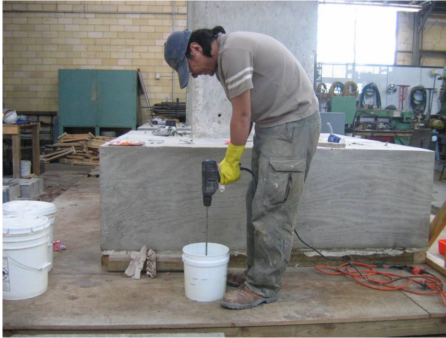
Figure B.2.7 Prepare epoxy resin
