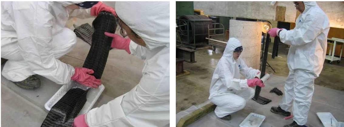
Figure 3.25 Saturate CFRP sheet with the epoxy resin and remove excess epoxy
