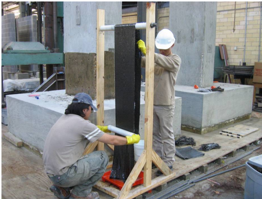
Figure B.2.12 Remove excess epoxy
