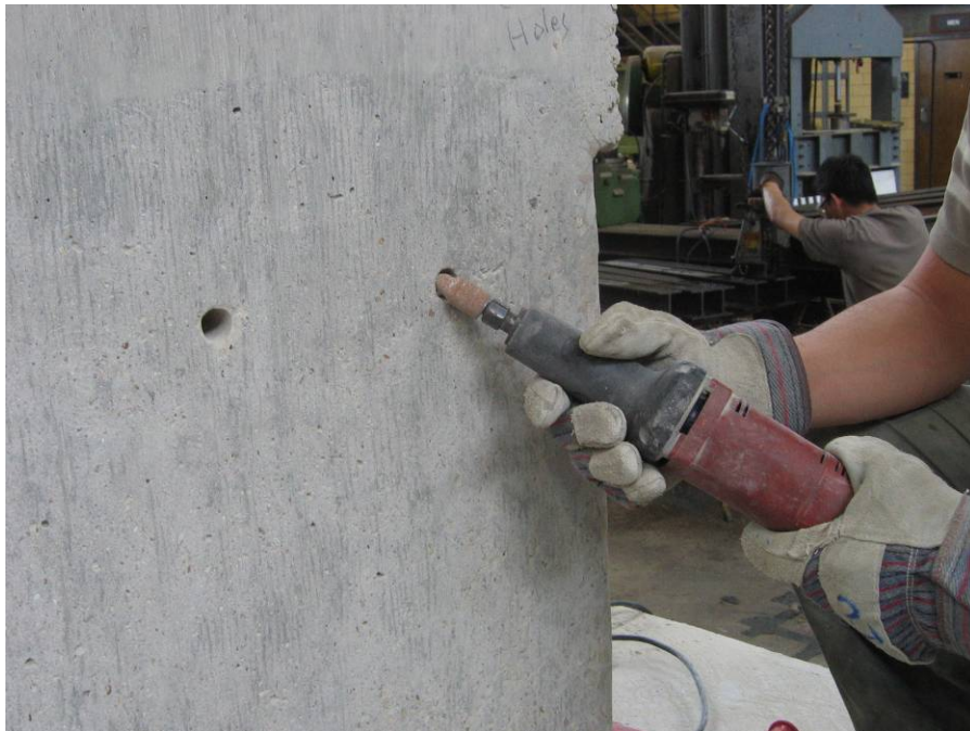
Figure B.2.2 Grind edge of the holes for CFRP anchors
