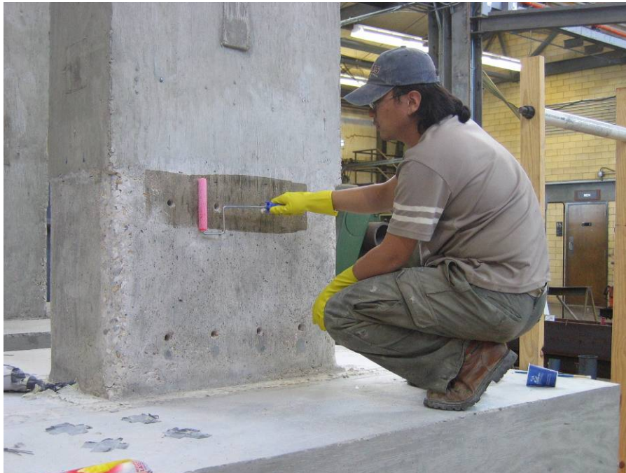
Figure B.2.8 Saturate the concrete surface with the epoxy resin
