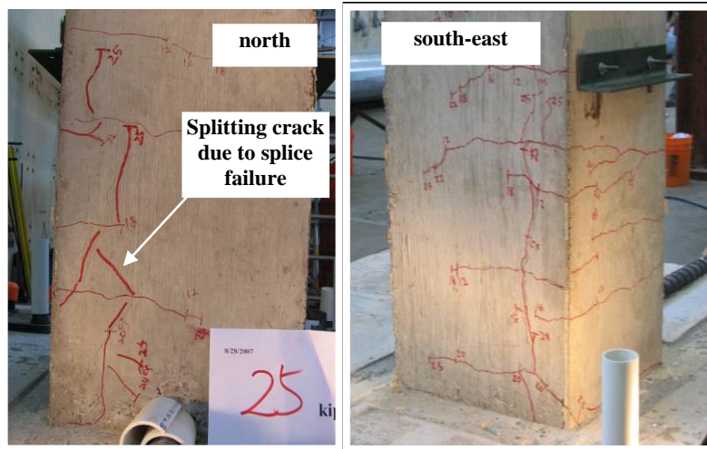
Figure 4.40 Splice failure of 2-A-S8-M before rehabilitation
