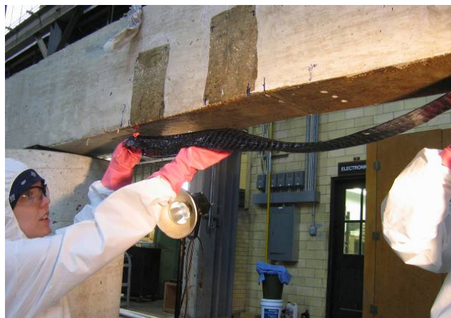
Figure 3.26 Place the CFRP sheet on the beam
