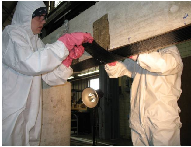
Figure 3.27 Saturate and place the CFRP U-wraps
