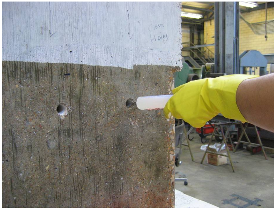
Figure B.2.9 Saturate the holes with the epoxy resin
