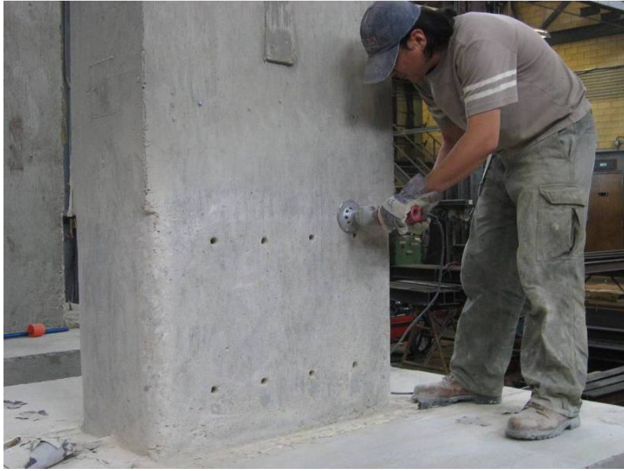
Figure B.2.3 Grind to roughen the concrete surface
