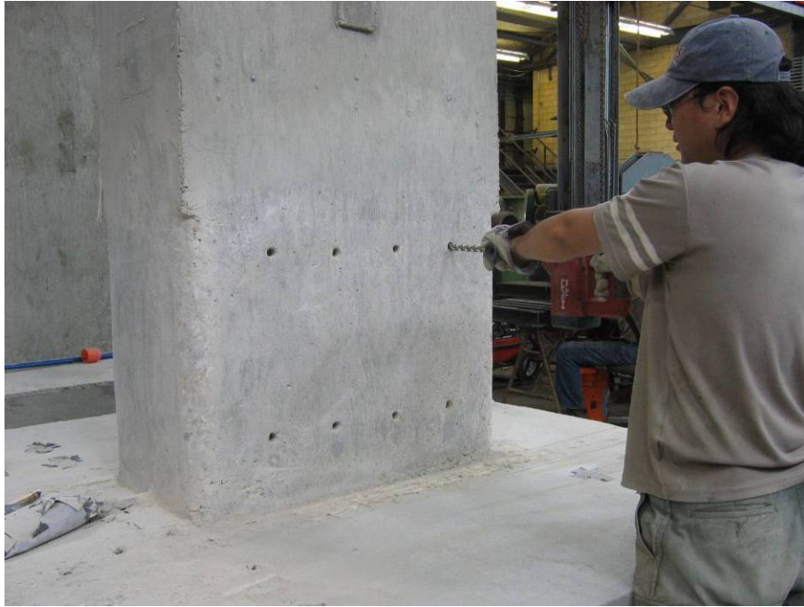
Figure B.2.1 Drill holes for CFRP anchors
