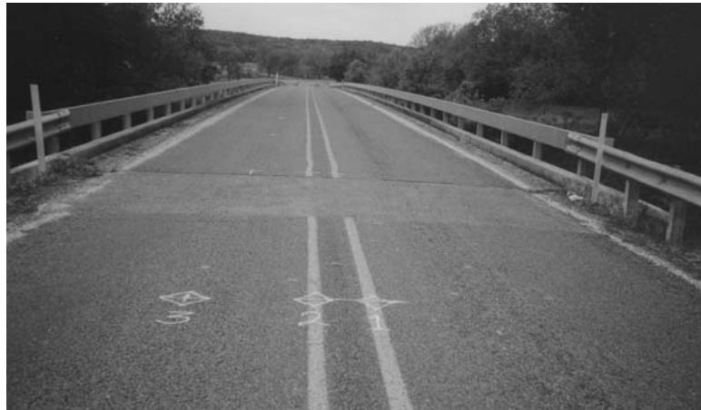
Figure 1.17: The Surface of the Leon River Bridge
