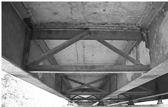
Figure 1.10: K-type and X-type Diaphragms
