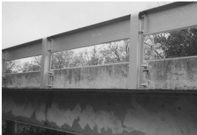
Figure 1.9: A Portion of the Railing on the Leon River Bridge
