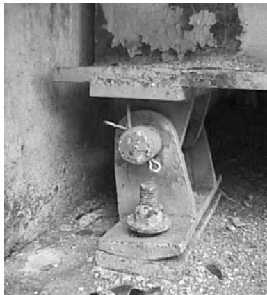
Figure 1.3: A Rocker Support at an Abutment
