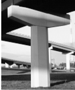
Figure 3.7: Pier with Chamfered Edges
