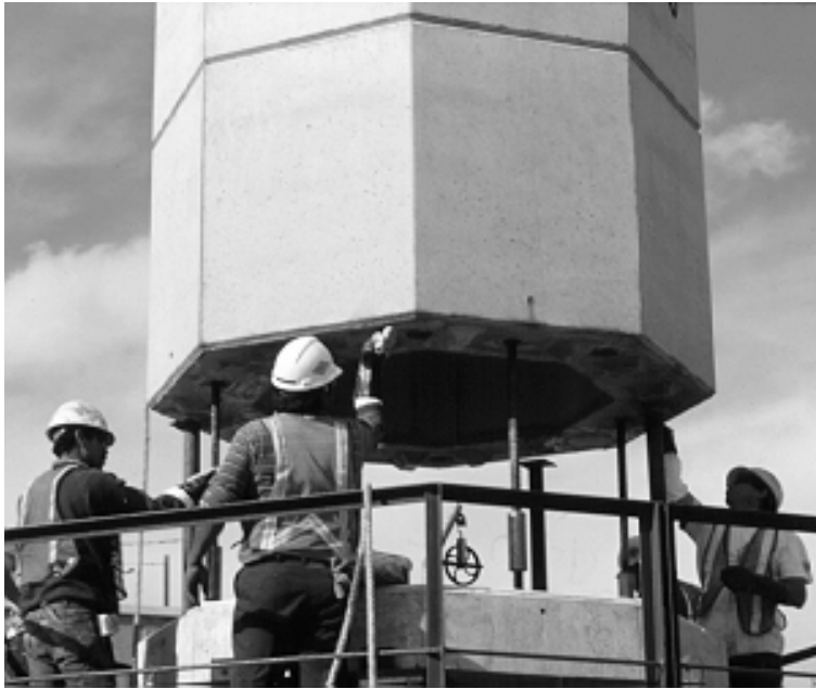
Figure 2.39: Applying Epoxy to Joint Faces
