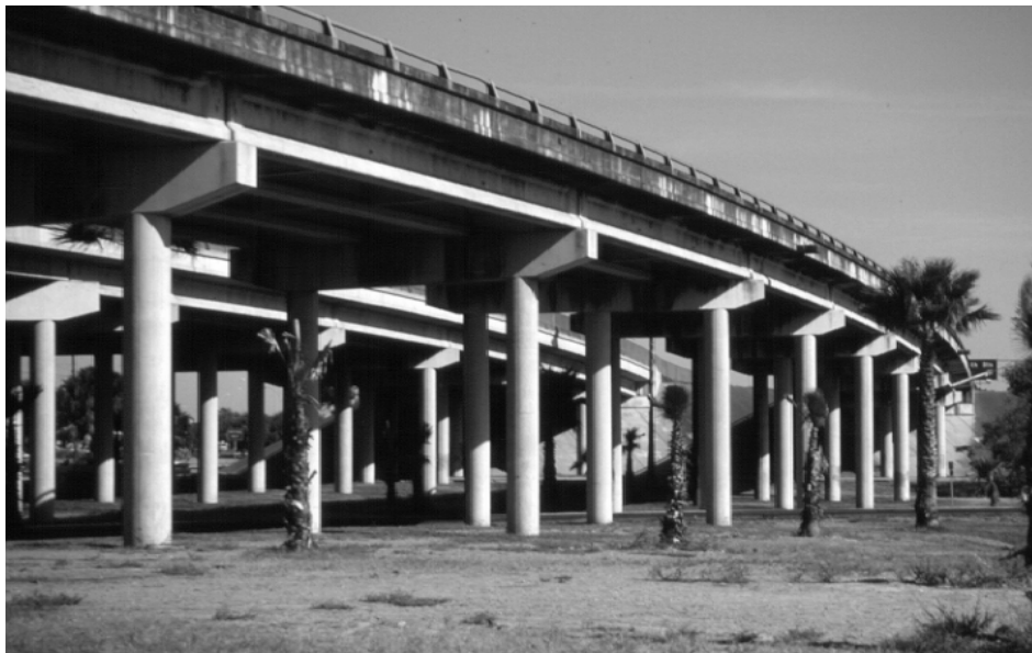
Figure 1.3: "Forest" of Columns
