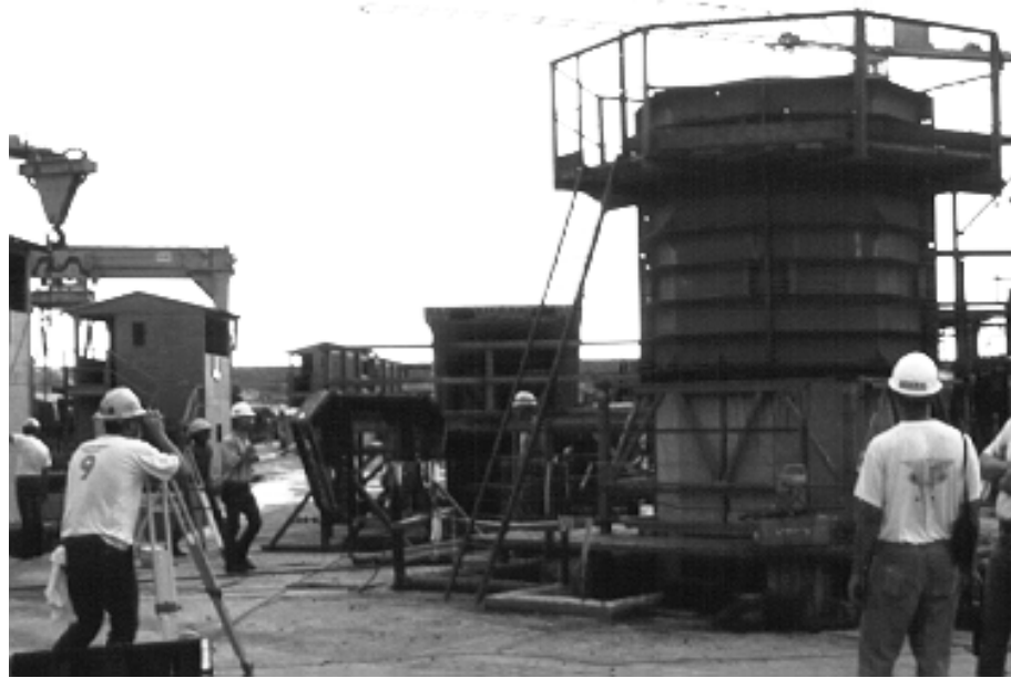
Figure 2.35: Checking Alignment of Segment and Form
