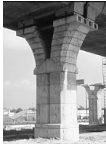
Figure 2.45: Mainlane "Y-Pier" for U.S. 183 Viaduct
