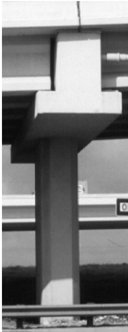
Figure 3.1: Inverted-T Bentcap
