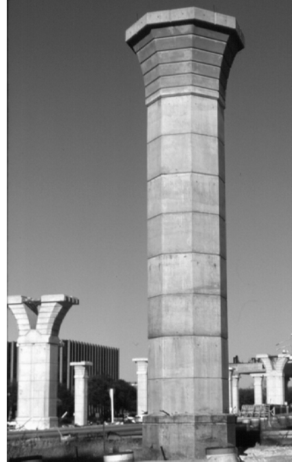
Figure 3.14: False Joints Complement Real Joints in U.S. 183 Viaduct Piers
