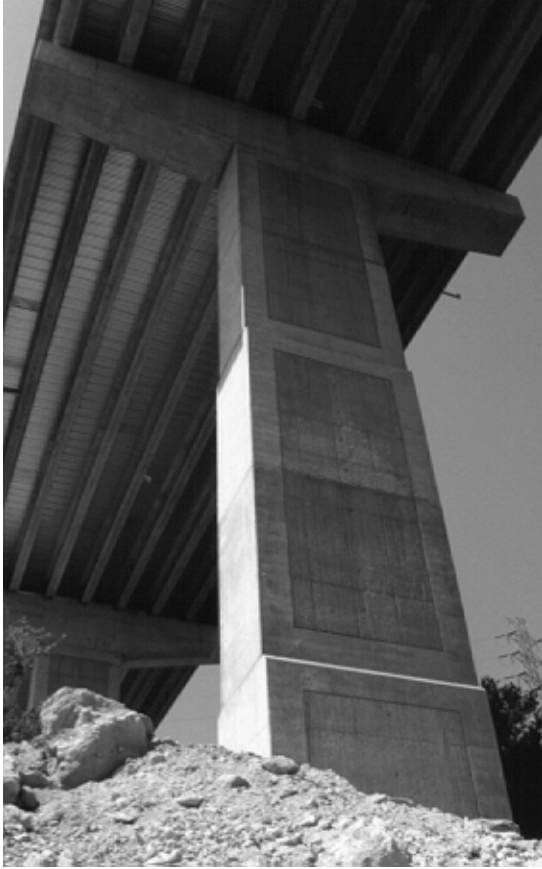
Figure 2.17: Texture Applied with Form Liners
