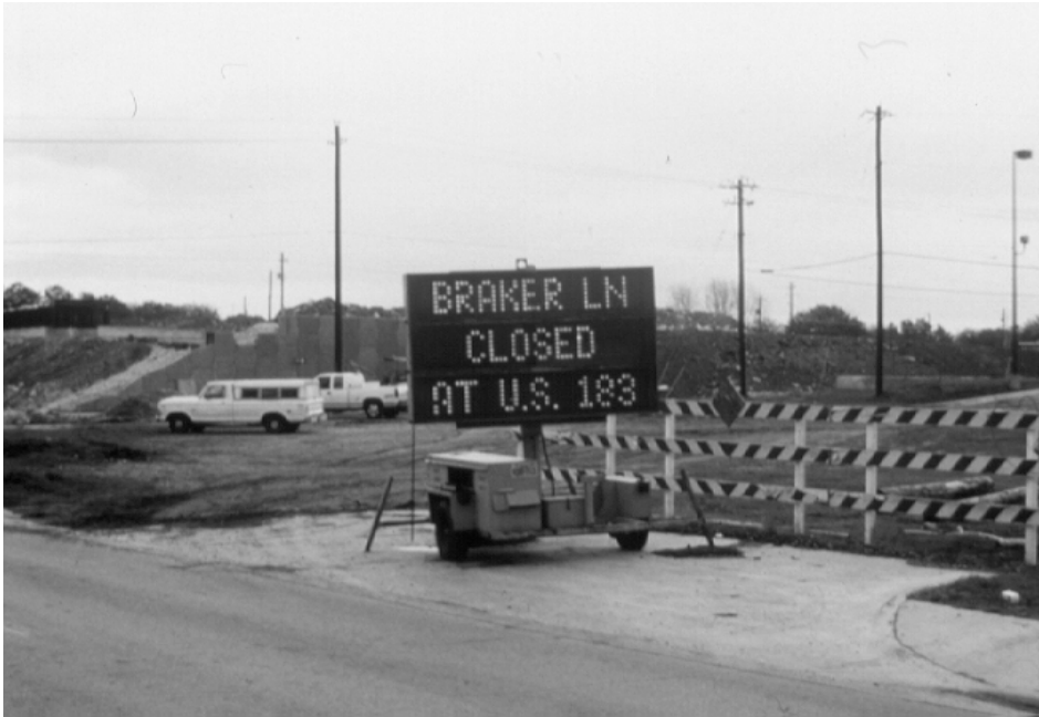
Figure 1.2: Traffic Impediment Due to Construction
