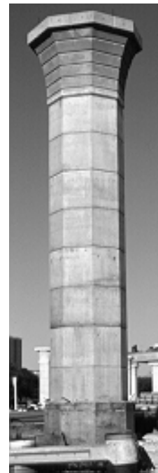
Figure 2.41: Completed Pier for U.S. 183 Viaduct
