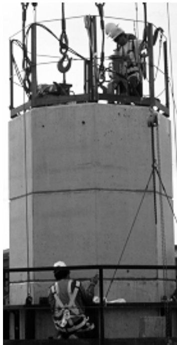
Figure 2.40: Stressing Post-tensioning Bars
