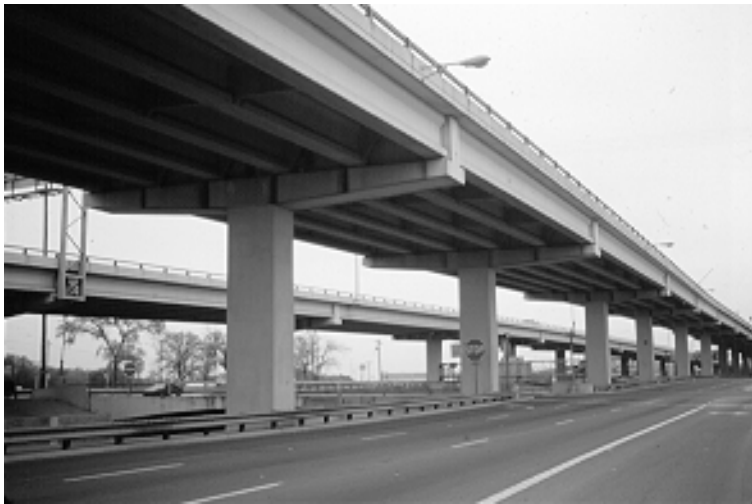
Figure 3.4: Inverted-T Caps with Tapered Soffits
