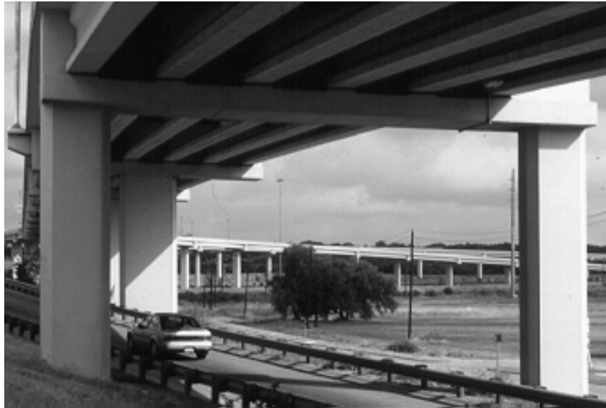
Figure 2.12: Straddle Bent
