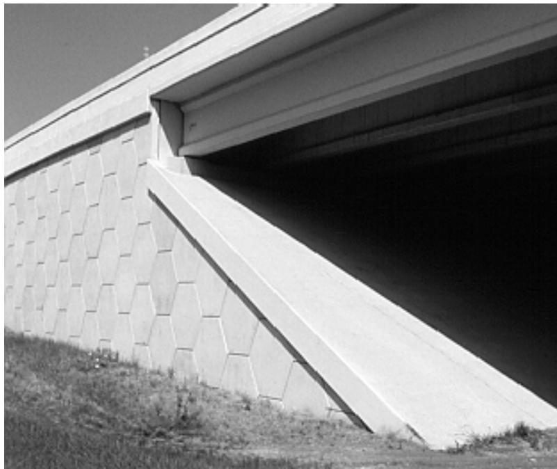
Figure 2.8: "Stub" Abutment with Retaining Wall
