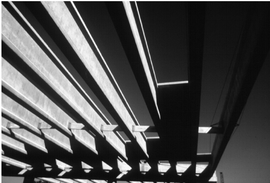
Figure 1.1: Precast, Pretensioned I-Beam Superstructure Construction
