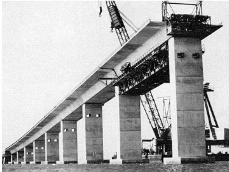
Figure 2.26: Completed Precast Segment Piers for Dauphin Island Bridge (from Ref. 12)
