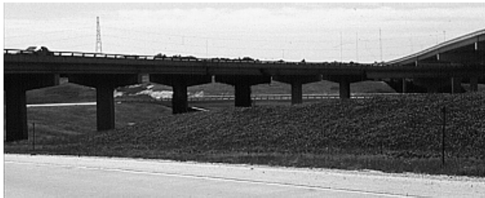
Figure 3.3: Hammerhead Bents Reduce Substructure Transparency
