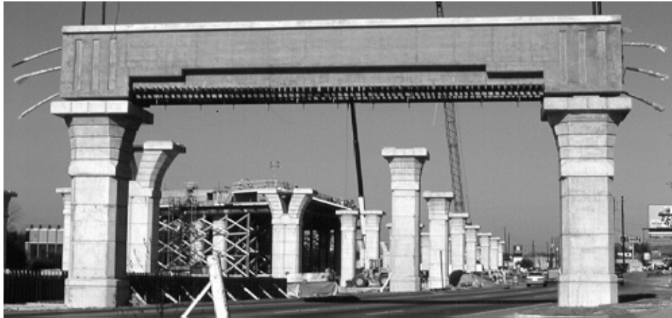
Figure 2.15: Post-tensioned Straddle Bent
