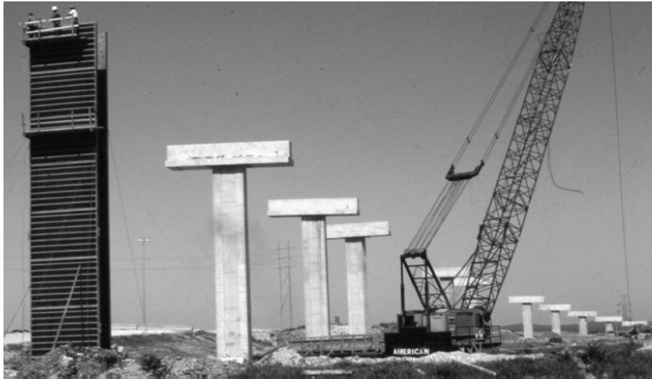
Figure 1.5: Repetitive Substructure Construction
