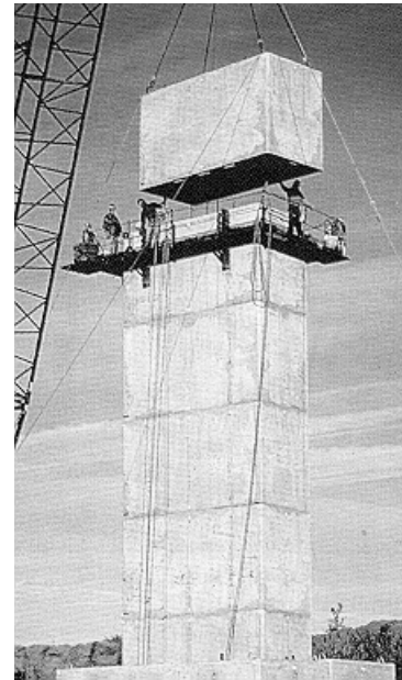
Figure 2.27: Erection of Box Piers for C&D Canal Bridge (from Ref. 13)
