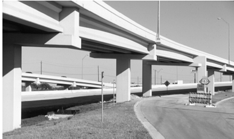
Figure 3.2: Substructure Transparency Enhanced by Inverted-T Caps
