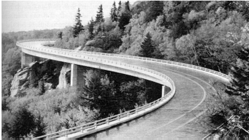
Figure 2.21: Linn Cove Viaduct (from Ref. 7)
