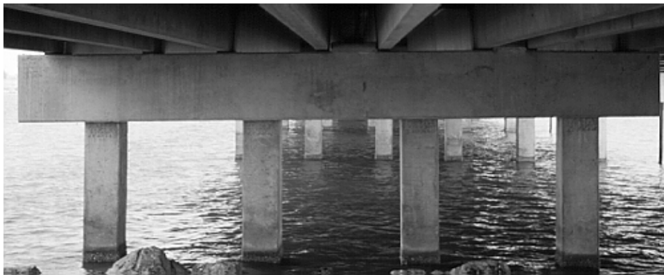
Figure 2.11: Trestle Pile Bent
