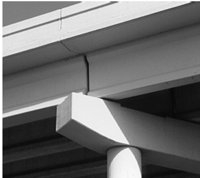
Figure 2.13: Chamfered End of Cap
