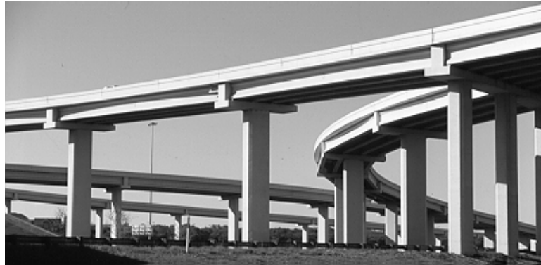
Figure 3.6: Use of Repetitive Elements Results in Orderly Substructure Flow
