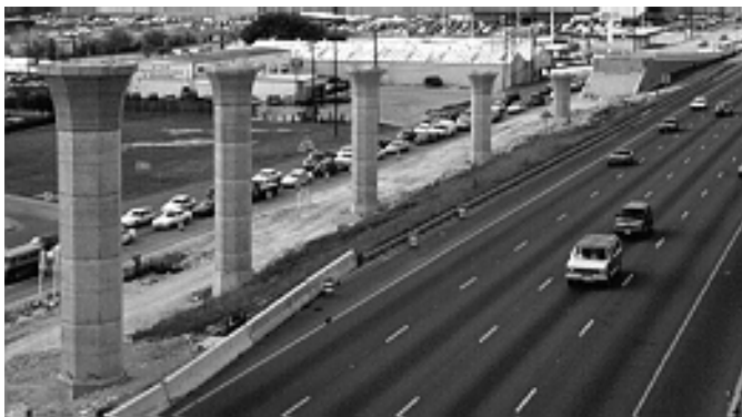
Figure 2.32: Large Ramp Piers for U.S. 183 Viaduct
