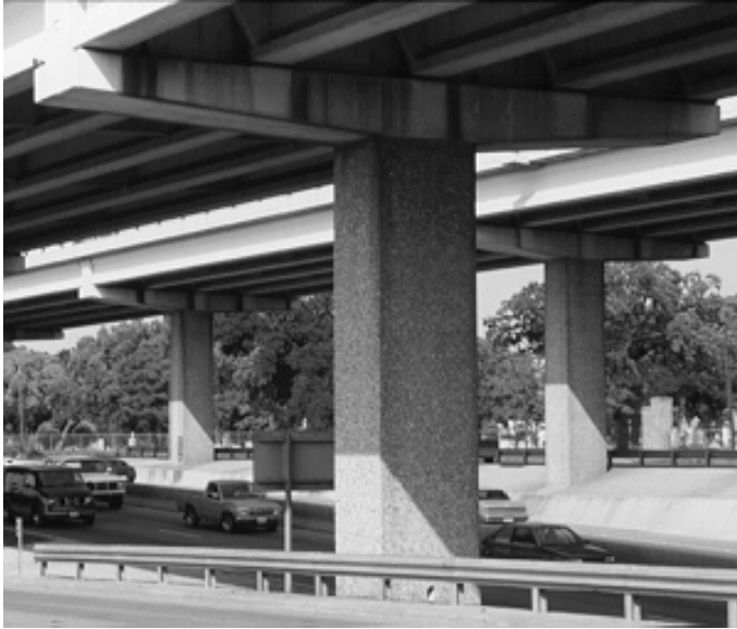
Figure 2.14: Tapered Cap Soffits
