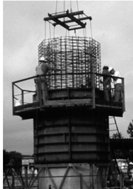
Figure 2.34: Lowering Reinforcement Cage into Outer Form
