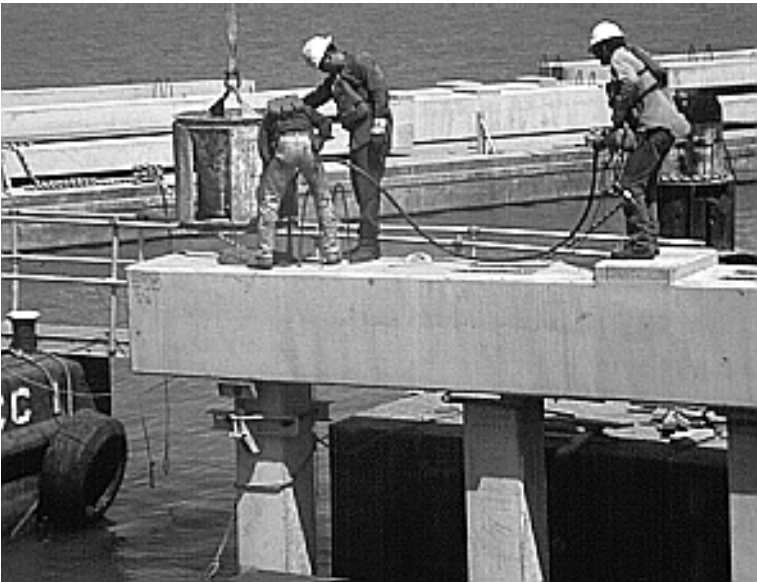
Figure 2.29: Connecting Precast Cap to the Piles for the Redfish Bay Bridge
