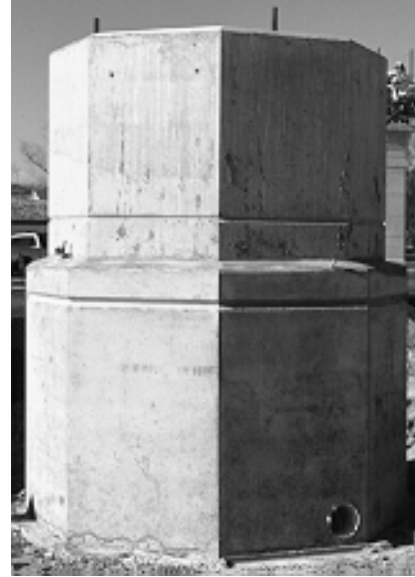
Figure 2.38: Starter Segment with Cast-in-Place Pedestal
