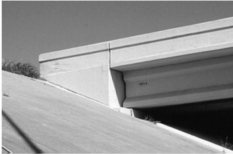
Figure 2.7: Typical "Stub" Abutment with Wingwall
