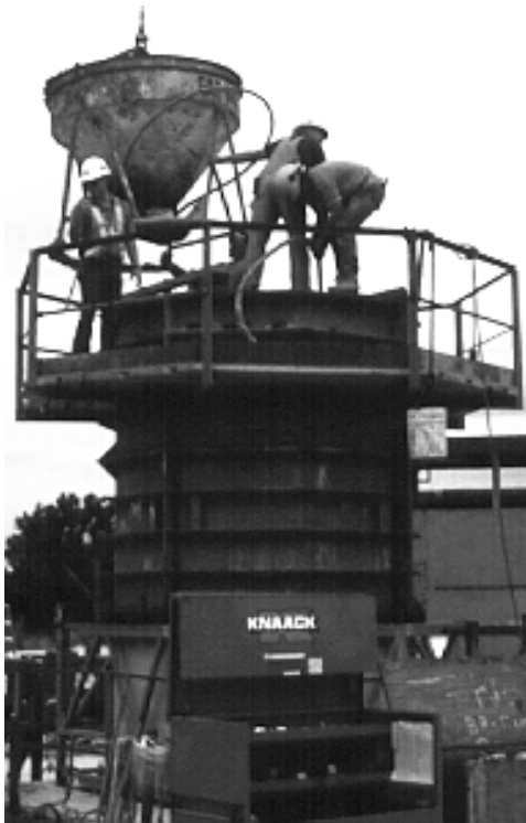
Figure 2.36: Casting Segment Concrete
