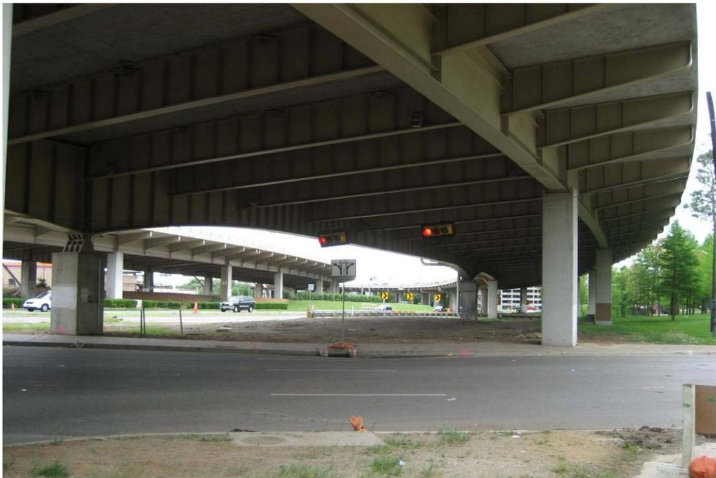
*Figure 1.14: Asymmetrical Columns and Haunches of Section F17S*
