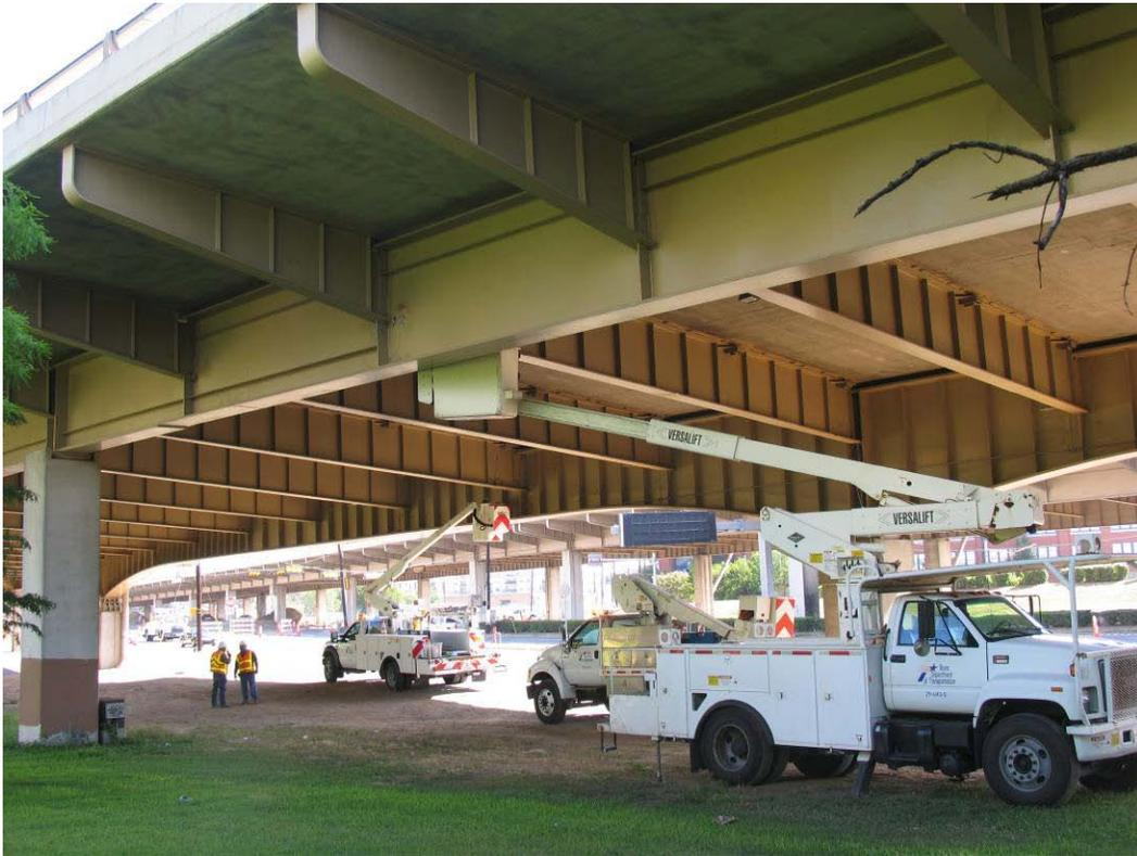
*Figure 2.4: Bucket Trucks used to Place Strain Gages*
