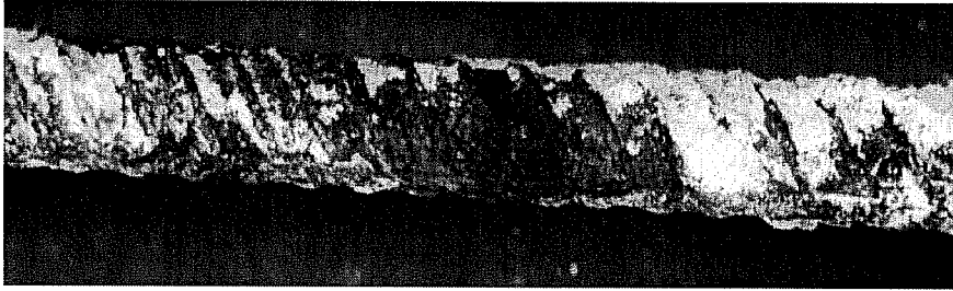
Figure 5.18 Corrosion Outside the Previous Exposed Region (Beam 12).
