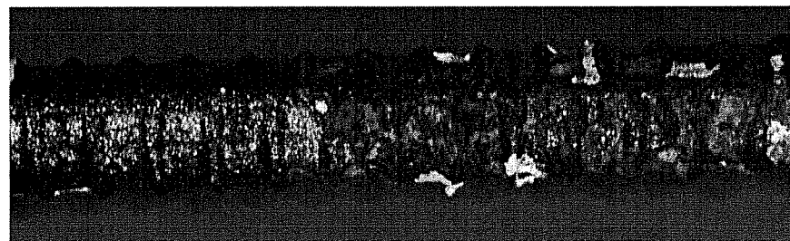
Figure 5.13 Rust Stains Underneath Coating on Epoxy-coated Bar (Beam 12).
