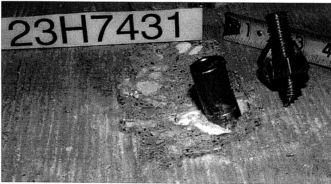
Failure Picture of Test 23H7431, Sleeve M16, Oblique Tension 30°
