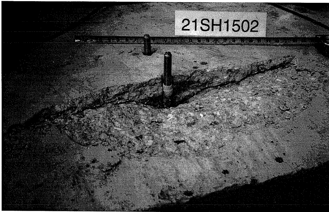
Failure Picture of Test 21SH1502, Spacing of 1.5 * h_{ef} , Sleeve, Static, Concrete Failure at Anchor
