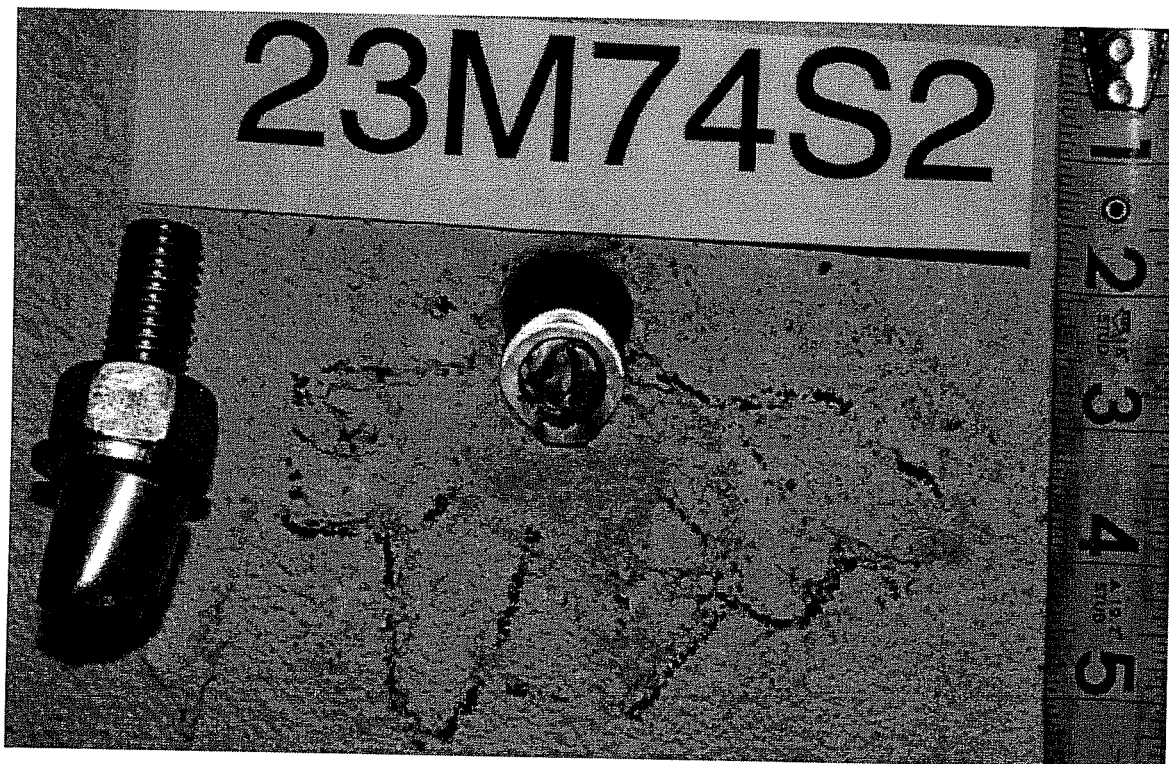
Failure Picture of Test 23M74S2, UC1 5/8", Shear
