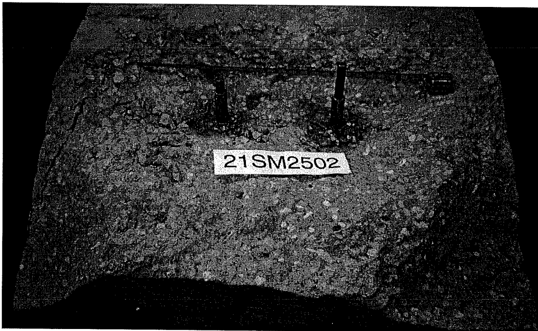
Failure Picture of Test 21SM2502, Spacing of 2.5 * h_{ef} , UC1, Static, Concrete Failure at Both Anchors of Group and Splitting of End of Specimen
