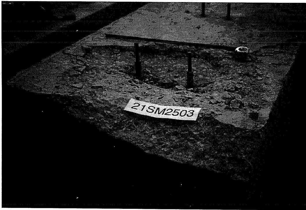
Failure Picture of Test 21SM2503, Spacing of 2.5 * h_{ef} , UC1, Static, Concrete Failure at Both Anchors of Group
