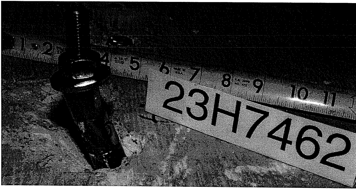
Failure Picture of Test 23H7462, Sleeve M16, Oblique Tension 60°
