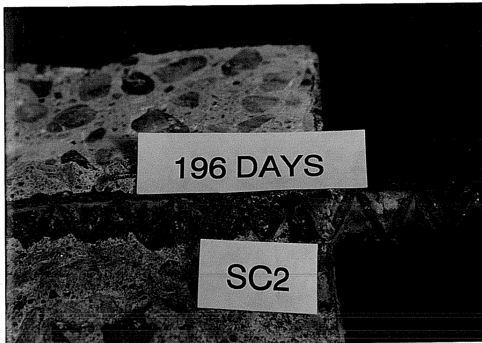
Figure 5- 19 Corrosion locations typical of high ratio zinc silicate specimens
