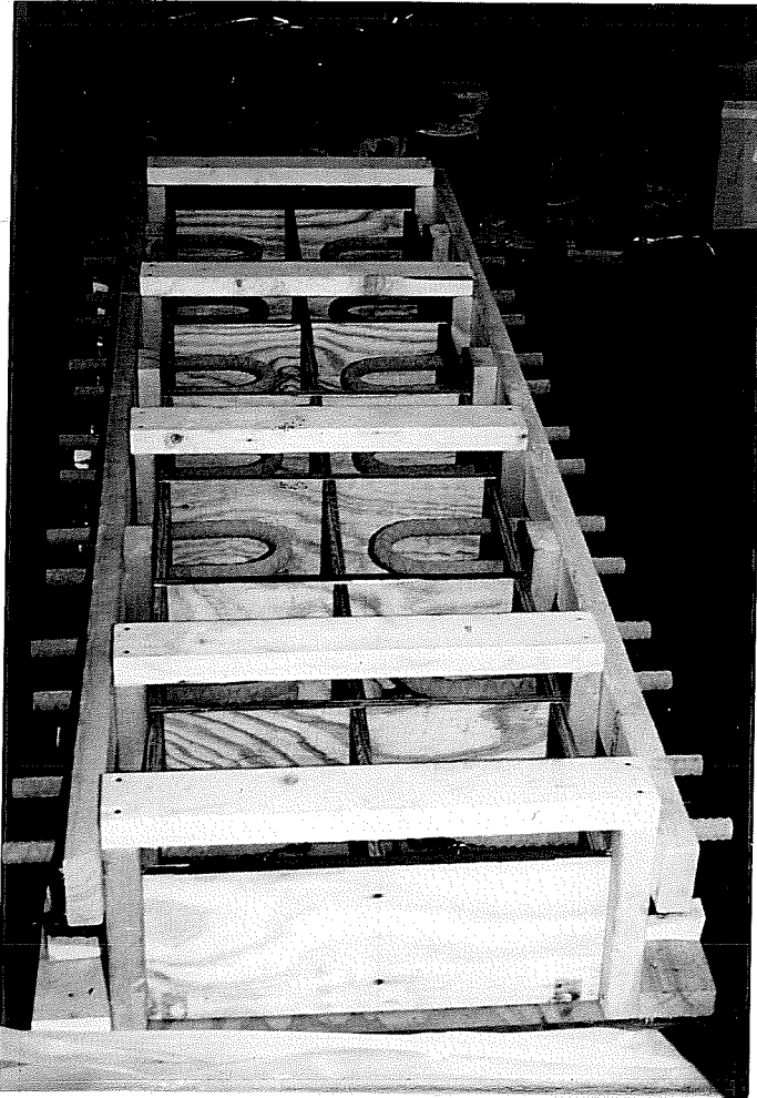
Figure 4-13 Completed macrocell formwork
