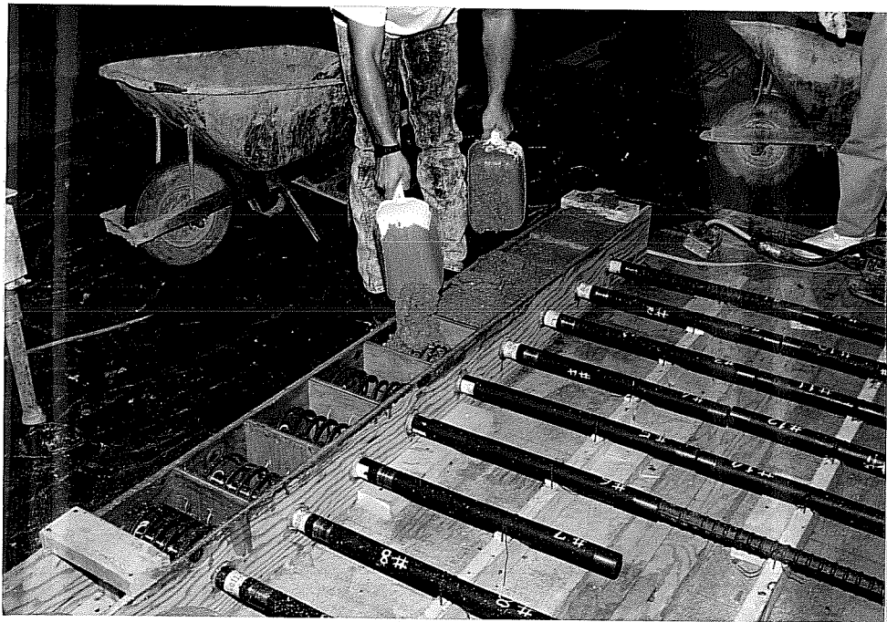
Photo 5.2 Concrete cast in specimens
