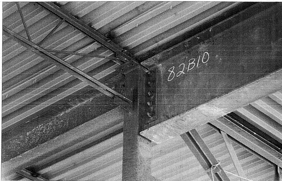
Photograph 7: Tube Column Connection to Wide Flanges and Bar Joists
