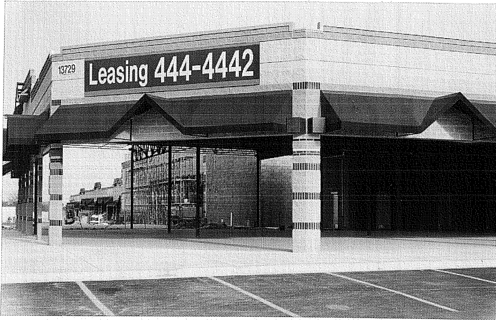
Photograph 5: Tube Columns in a One Story Strip Mall
