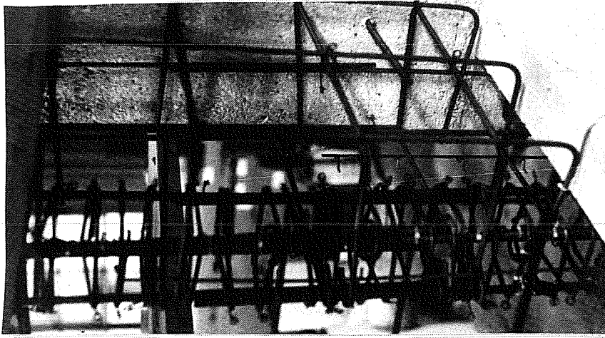
Fig. 2.31 Hooked #3 longitudinal bars in window area
