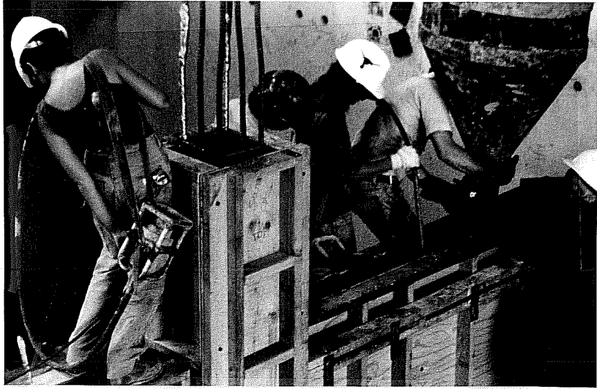
Fig. 2.18 Placing concrete in upper portion of beam form.
