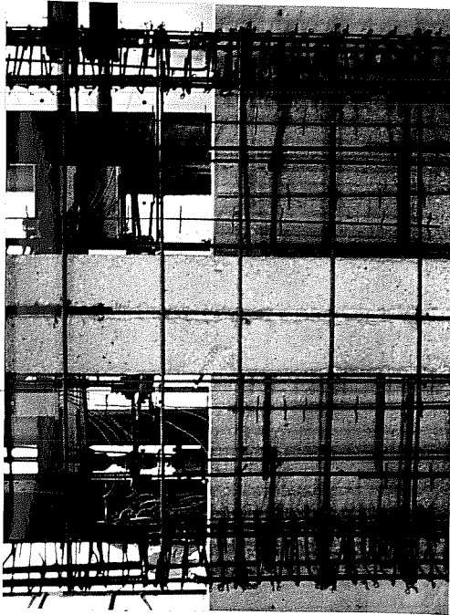
Fig. 2.30 Transverse and longitudinal steel in place.
