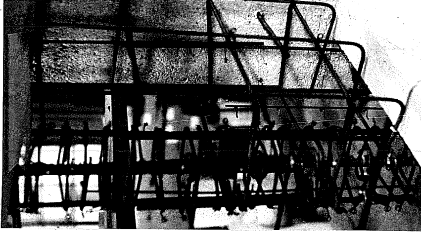
Fig. 2.31 Hooked #3 longitudinal bars in window area.
