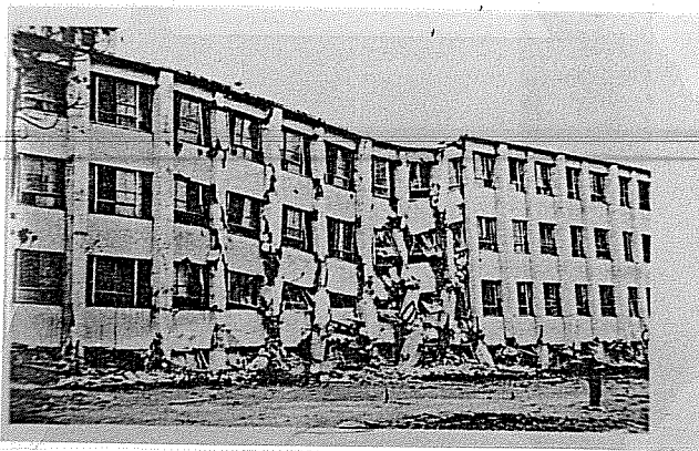
Fig. 1.3 Severe damage due to short column shear failure. Hokodate Coleege, Tokachi-oki 1968. [10]
