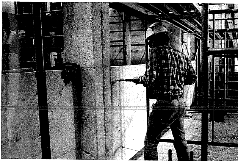
Fig. 2.24 Drilling holes for dowels.
