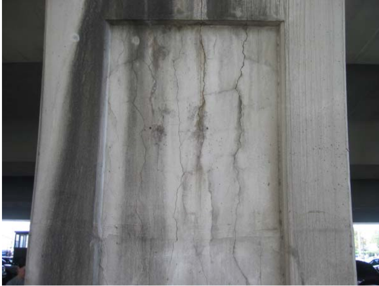
Figure 1.3: DEF Related Damage in DD-6
