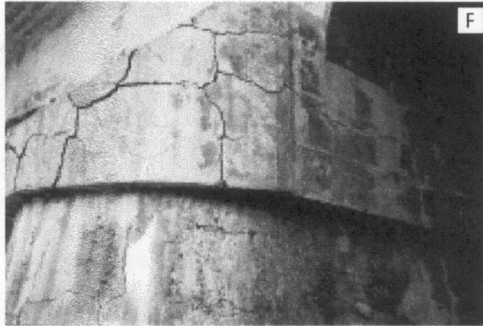
(f) Severe map-cracking in the exposed portion of the pier cap of a 35-year-old highway bridge.
