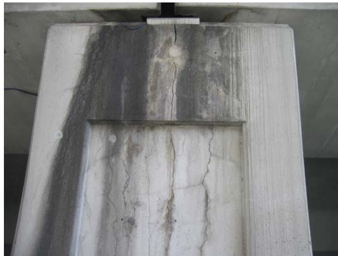
Figure 2.2: Longitudinal Cracking of Spine DD Column
