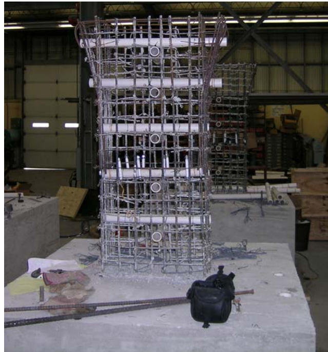
Figure 4.6: Column Reinforcement Cage
