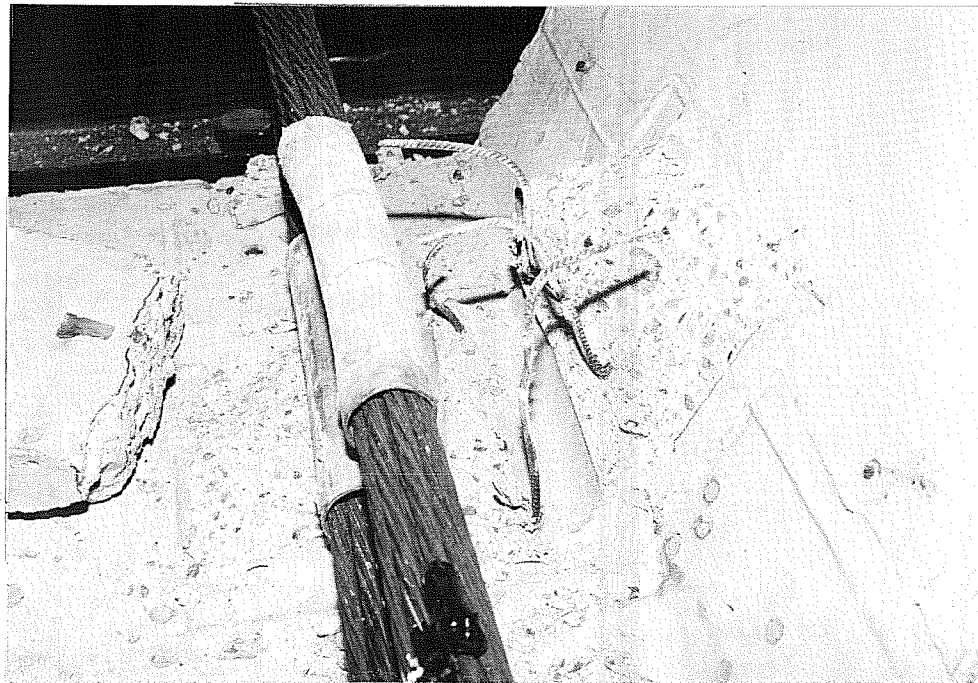
Figure 3.24 Test 2A - Before and After Failure
