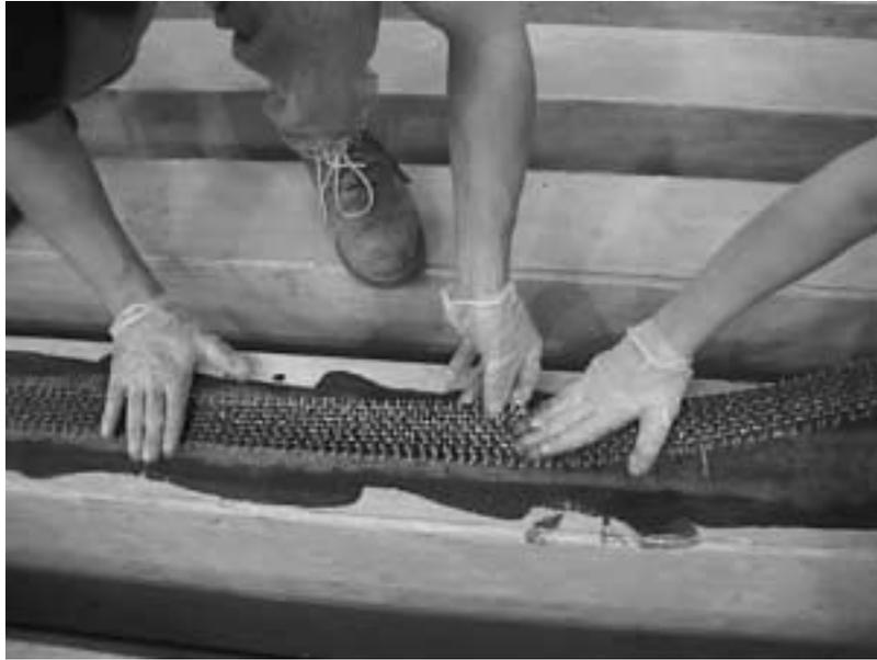
*Figure 4.5 Composite System C: Woven Unidirectional Carbon Fibers*
