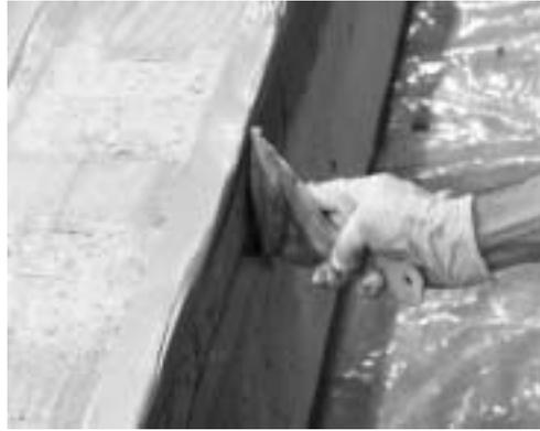
b) CFRP plate cleaning
