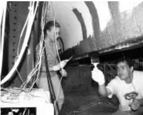
d) Placing carbon fiber sheet on joist
