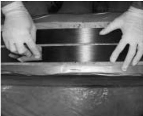
e) Positioning CFRP plate on beam
