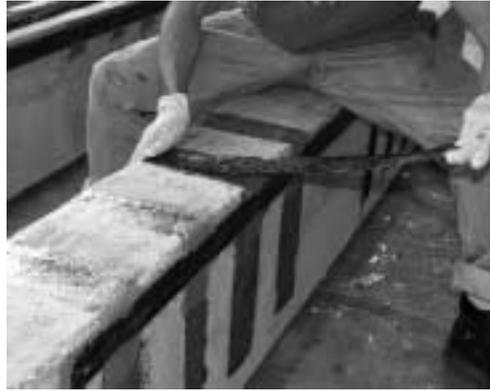
b) Applying epoxy on concrete surface
