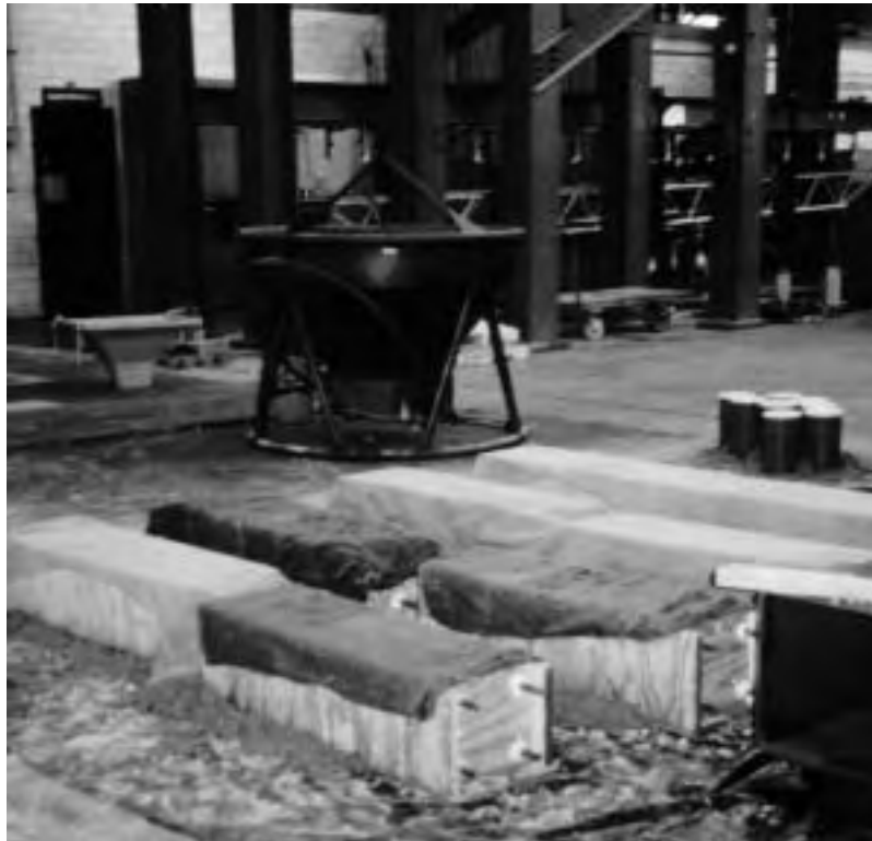
Figure 4.5 Wet-mat curing of beams
