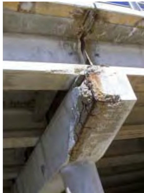
Figure 3.1 Endcap delamination
