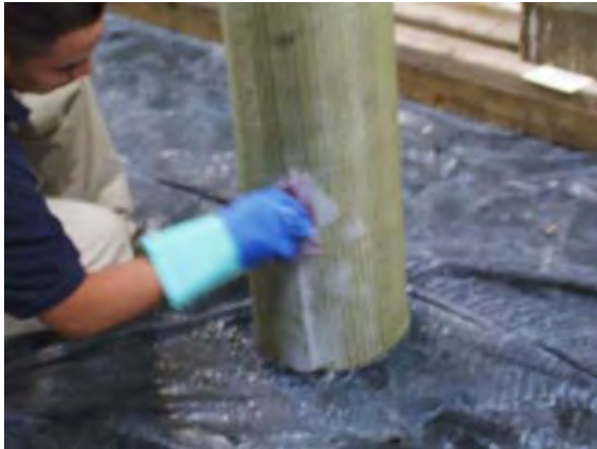
Figure 4.17 Sealing joints of column wrap
