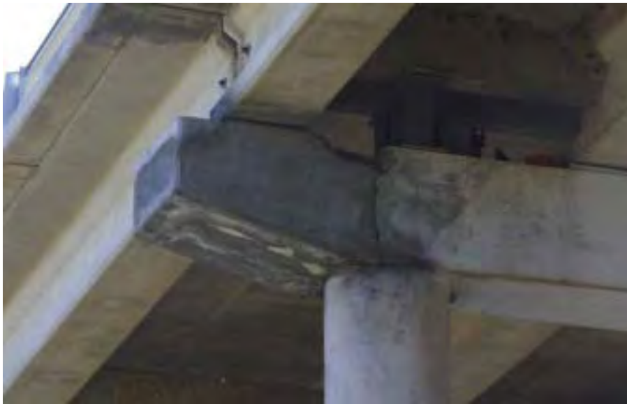
Figure 5.5 Endcap repair material on Structure #3
