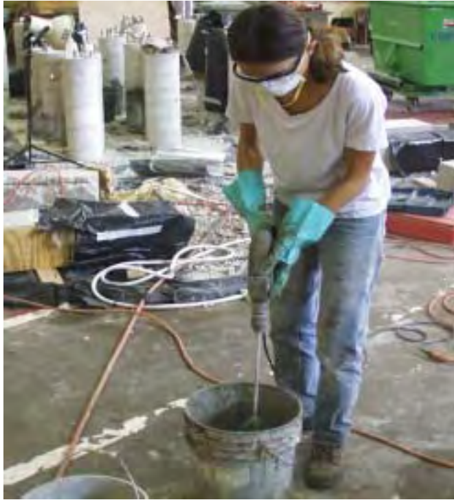
Figure 4.9 Mixing repair materials
