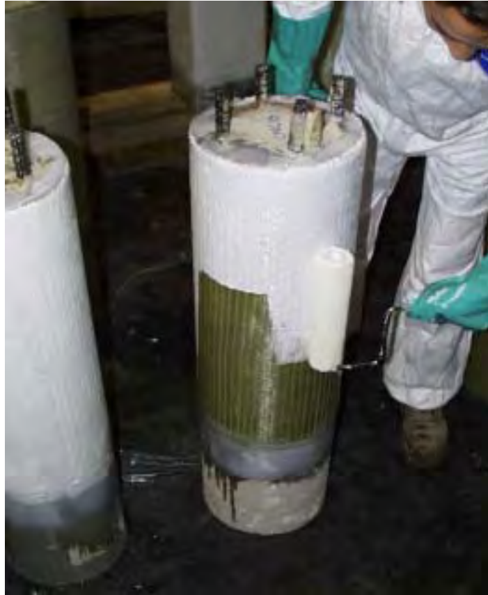
Figure 4.18 Painting wrapped column
