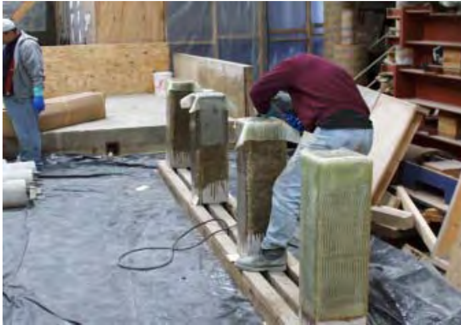
Figure 4.15 Wrapping beams
