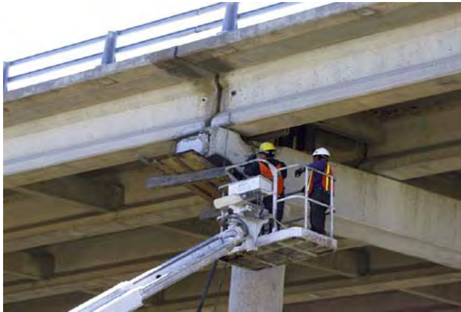
Figure 5.4 Application of Shotpatch® 21F to Structure #3
