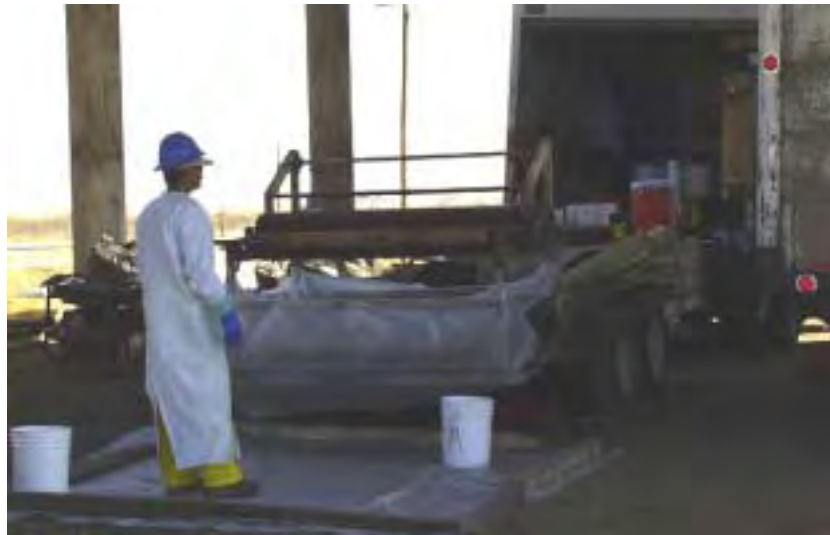
Figure 5.6 Saturation machine used by Delta Structural Technology, Inc.
