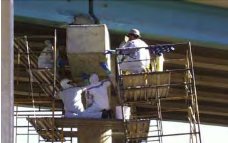
Figure 5.8 Removal of air pockets beneath a layer of Fibrwrap®
