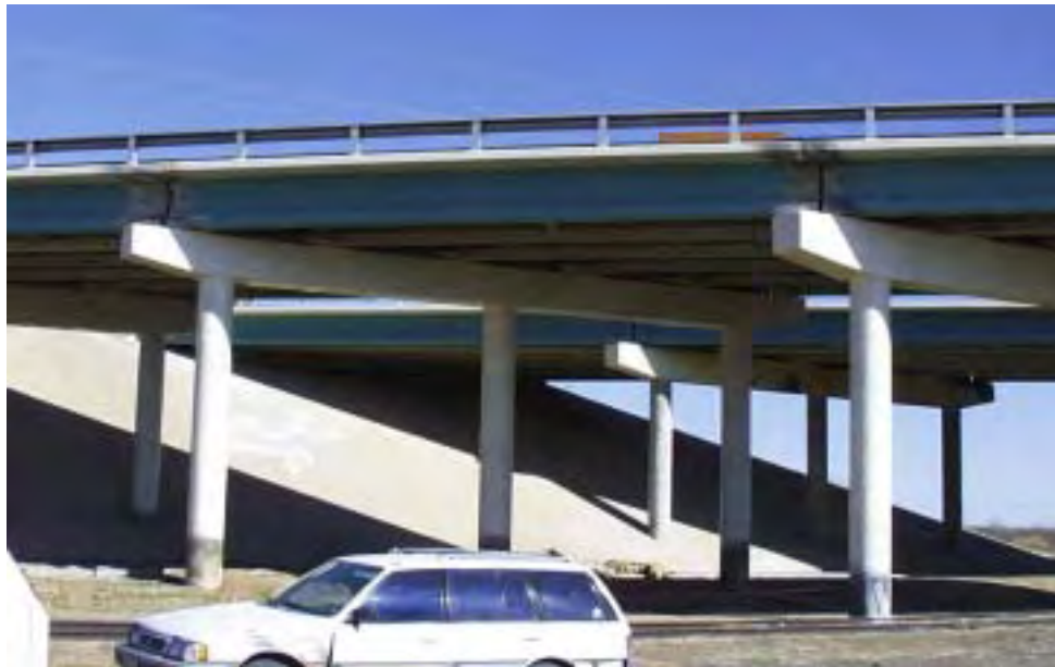
Figure 1.1 Structure wrapped with FRP
