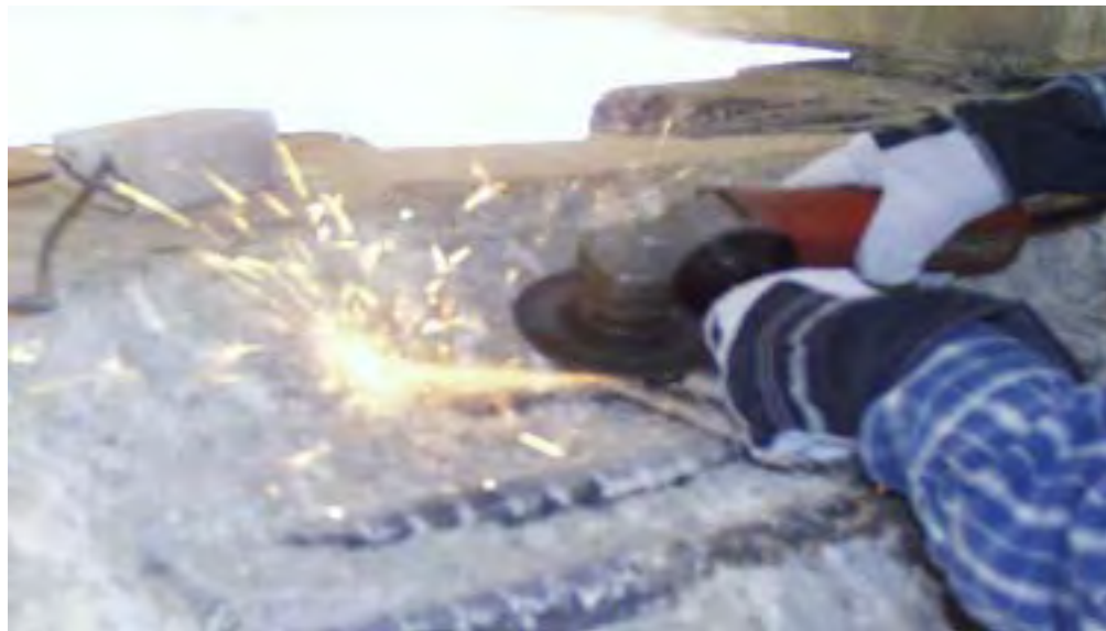
Figure 5.17 Grinding of the reinforcement to prepare for soldering
