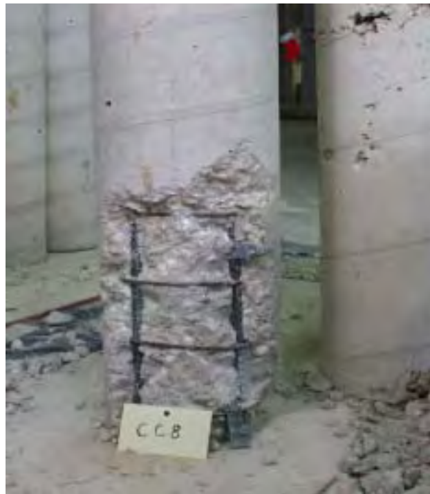
Figure 4.8 Concrete removed prior to repair
