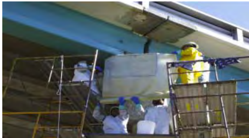
Figure 5.7 Application of Fibrwrap® to endcap on Structure #2
