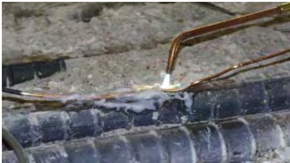
Figure 5.19 Application of flame to the copper-steel interface
