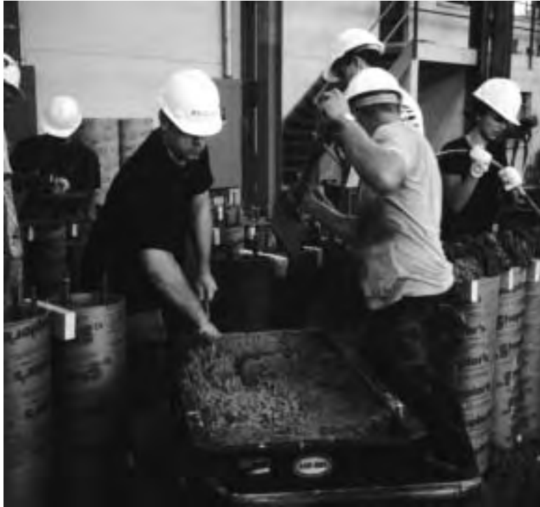
Figure 4.3 Placing concrete in cylindrical forms
