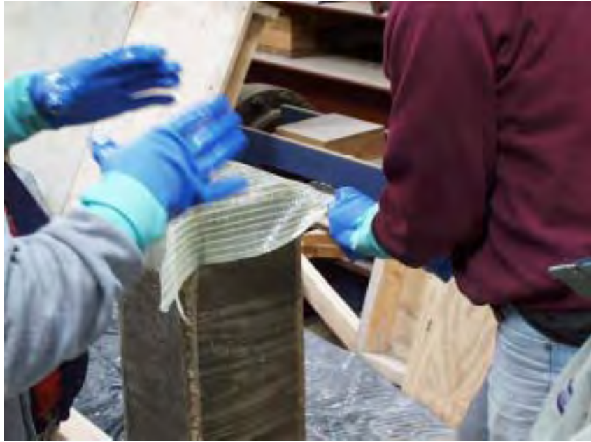
Figure 4.14 Wrapping beam end
