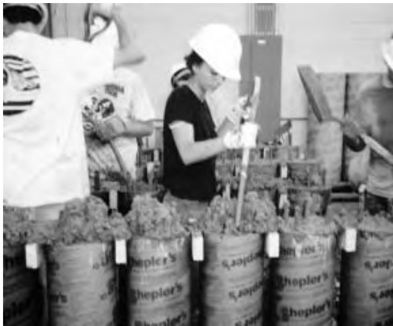
Figure 4.4 Vibrating concrete in columns
