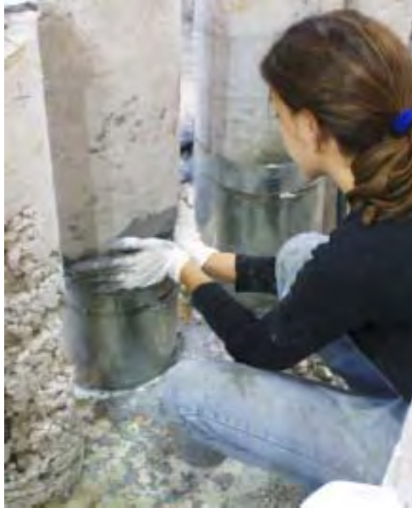
Figure 4.11 Drypacking procedure
