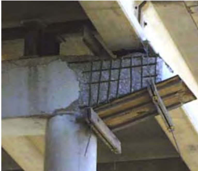
Figure 5.3 Endcap prepared for application of repair material on Structure #3
