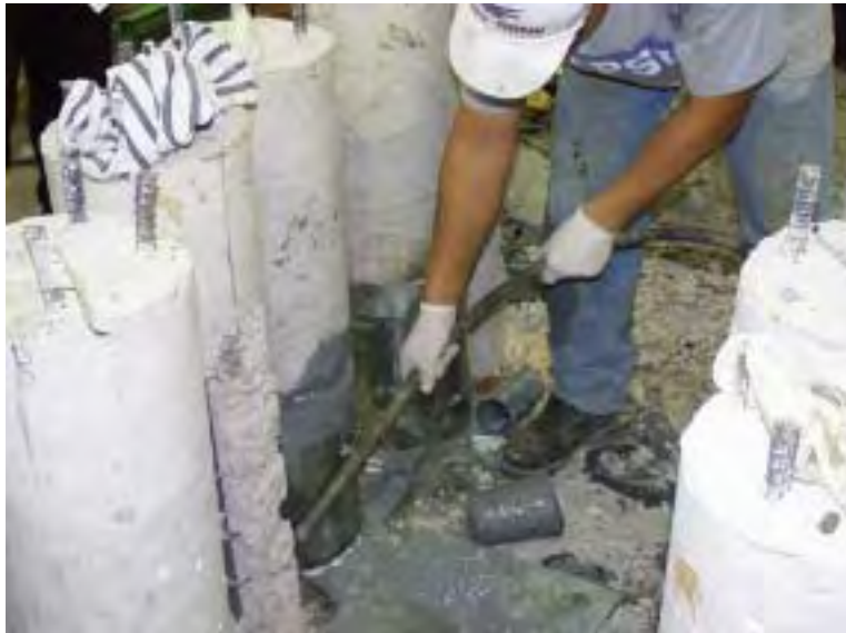
Figure 4.10 Vibrating columns
