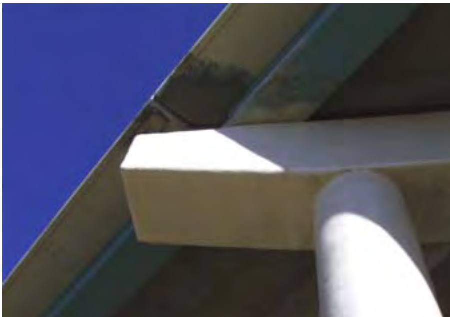
Figure 5.9 Wrapped and painted endcap on Structure #2
