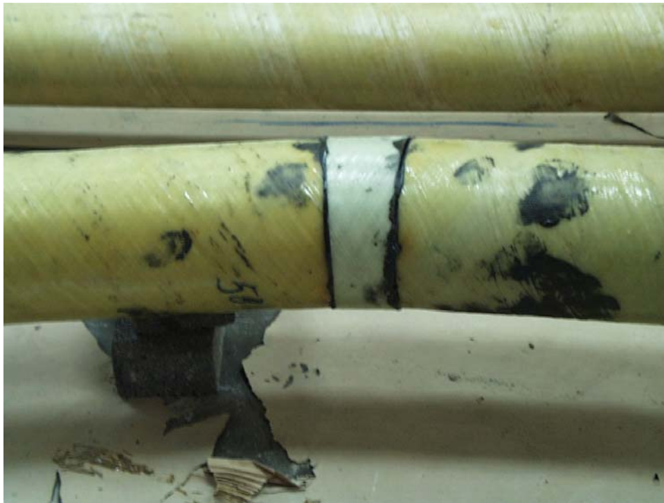
Figure 9.6. Assembled Connection Type 1 Prior to Final Wrap.
