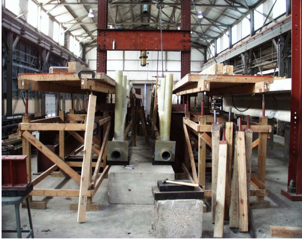
Figure 9.17. Arches in Place prior to Completing Formwork for RC Deck.
