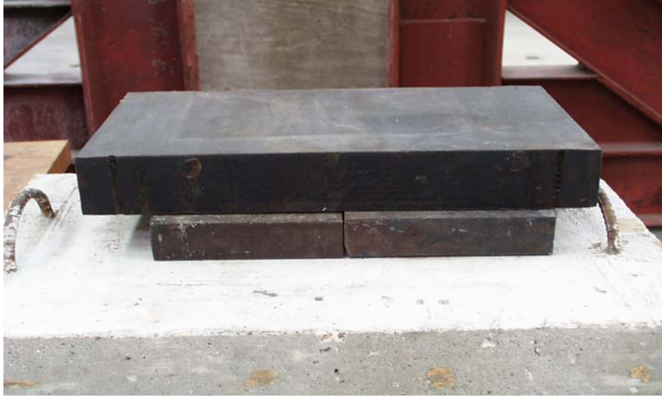
Figure 3.7. Elastomeric Bearing Support.
