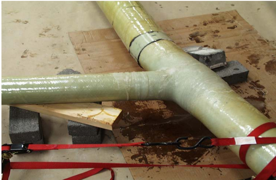
Figure 9.10 Finished Connection Type 2.
