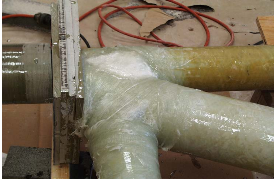
Figure 9.13. Finished Connection Type 3.
