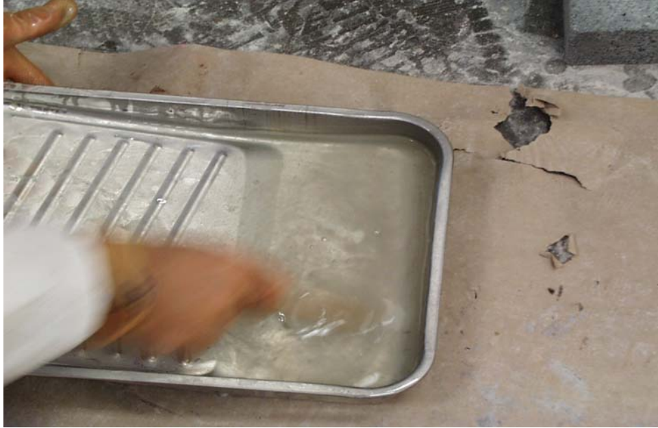
Figure 9.9. Wetting Fiberglass Fabric for Connection Type 2.
