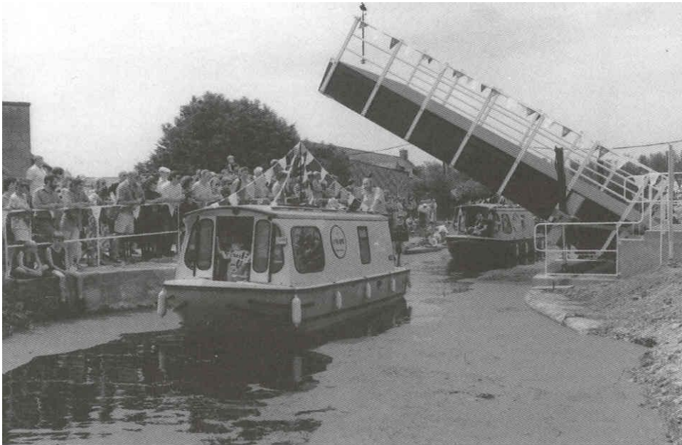
Figure 2.13. Bonds Mill Bridge (FHWA, 1997) .
