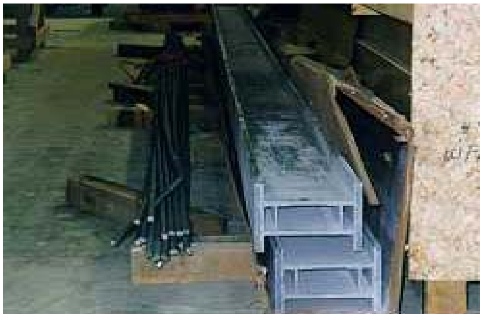
Figure 7.1. FRP Hybrid Girders Laid Sideways.
