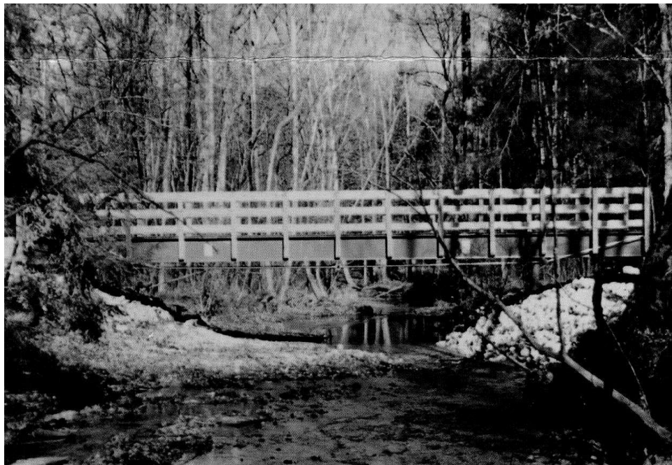
Figure 2.9. Daniel Boone National Park Footbridge (SPI, 1996).
