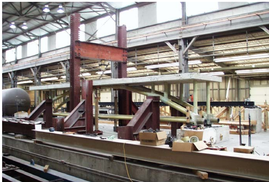
Figure 9.20. Specimen after Formwork Removal.
