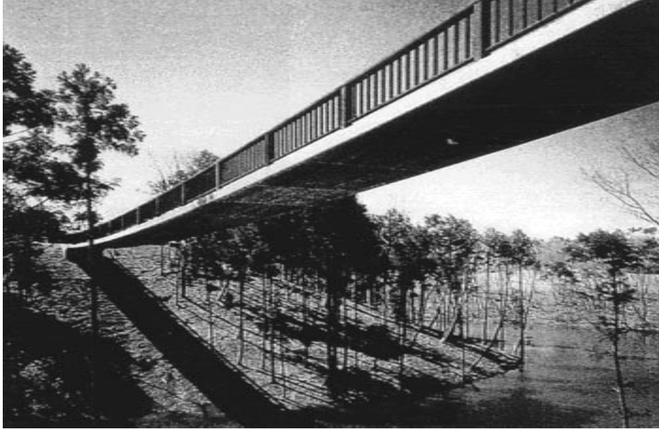
Figure 2.5. Birdie Footbridge (WTEC, 2001) .
