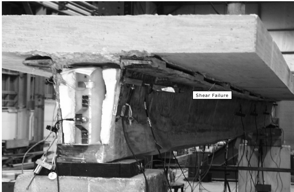
Figure 8.17. Shear Failure at Deck-Girder Interface at South End.
