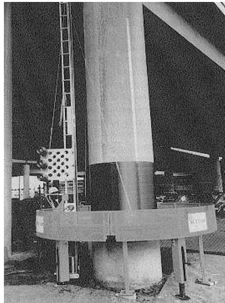
Figure 2.21. Caltrans Bridge Pier Retrofit (Hull, 1996) .
