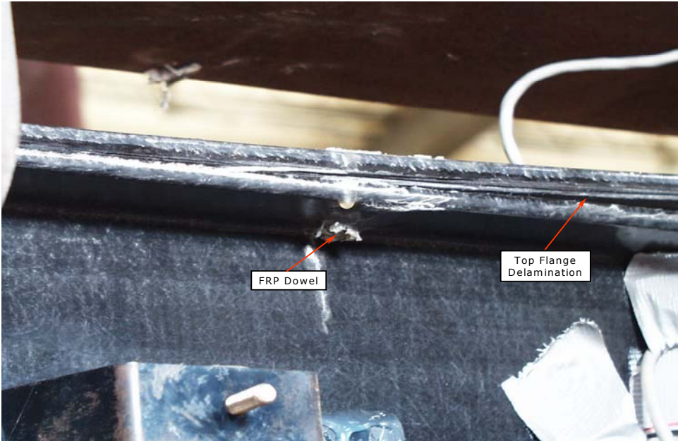
Figure 7.16. Specimen SW2 Top Flange Delamination.
