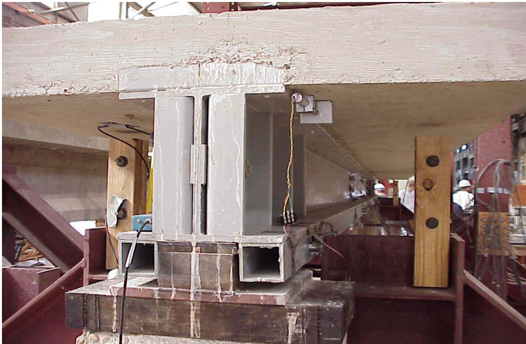
Figure 4.10. South End Support View.
