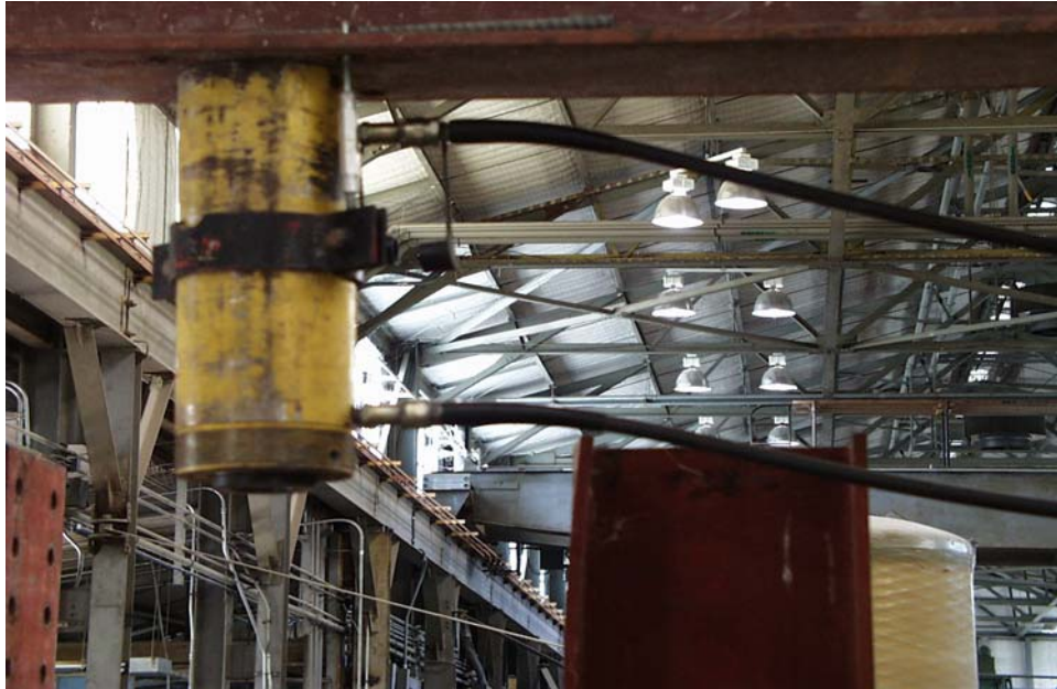
Figure 3.6. Hydraulic Jack and Hose System.
