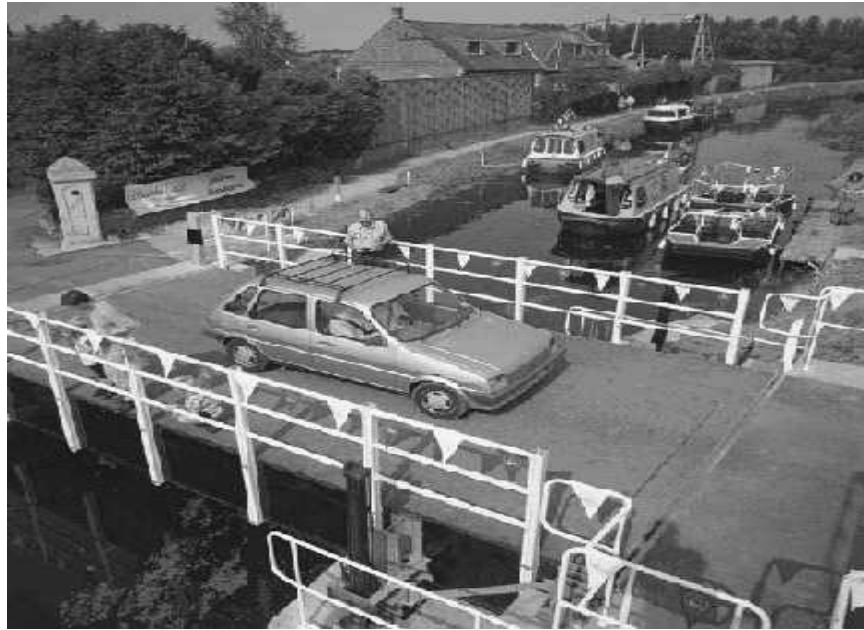
Figure 2.14. Bonds Mill Bridge (FHWA, 1997) .
