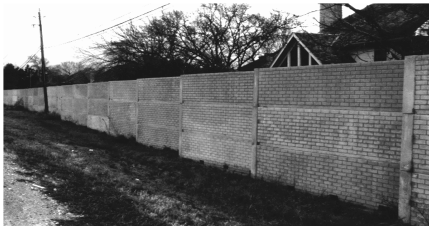
Figure 6.9 Example of staggered-wall system (Houston District)
