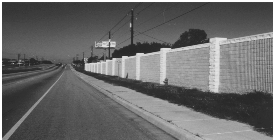
Figure 6.6 Constructed-in-place post-and-panel system (Austin District)
