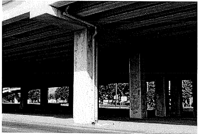
(b) Tacked on drain pipes and peeling paint create a feeling of decay
