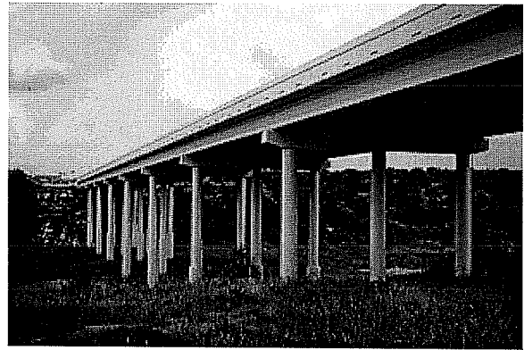
Figure 3. 16 A cluttered forest of columns
