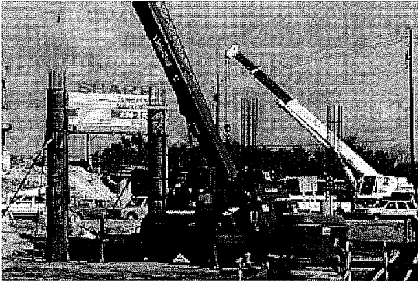
Figure 1.11 Extensive on-site equipment for cast-in-place multi-column bents
