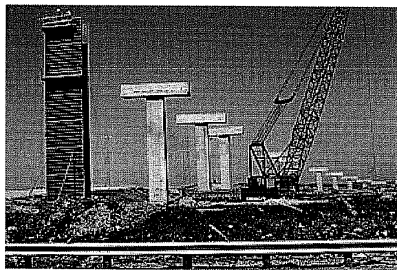
Figure 3. 44 Highly repetitive substructures requiring extremely tall and strong forms
