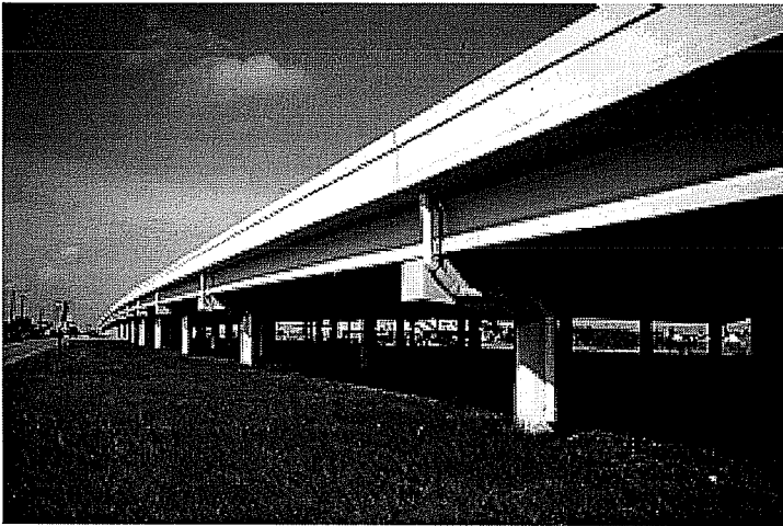
(a) Drain pipes tacked onto the substructure
