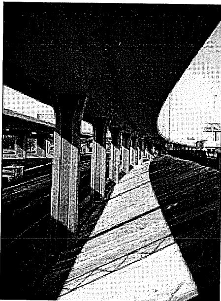
Segmental construction provided attractive and rapid construction for the highly visible and congested urban site
