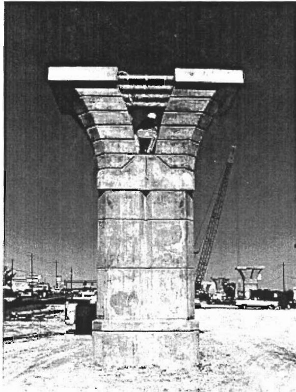
Figure 4.3 Typical mainlane pier.
