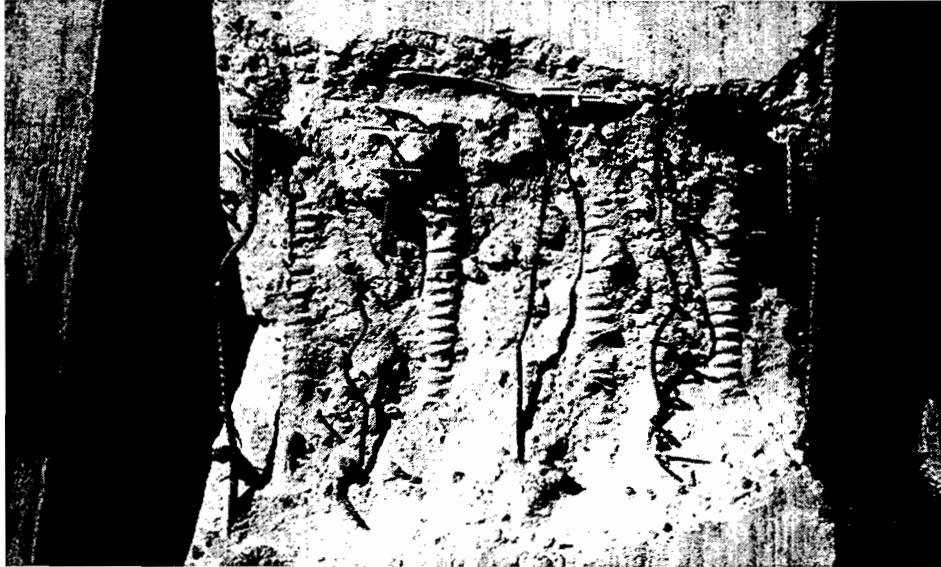
Figure 3. 83 Fractured tension reinforcement in north CO-PS-100S-NA-N-SM overhang
