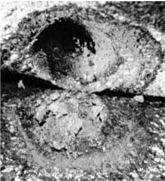
(b) Corrosion product buildup in blister
