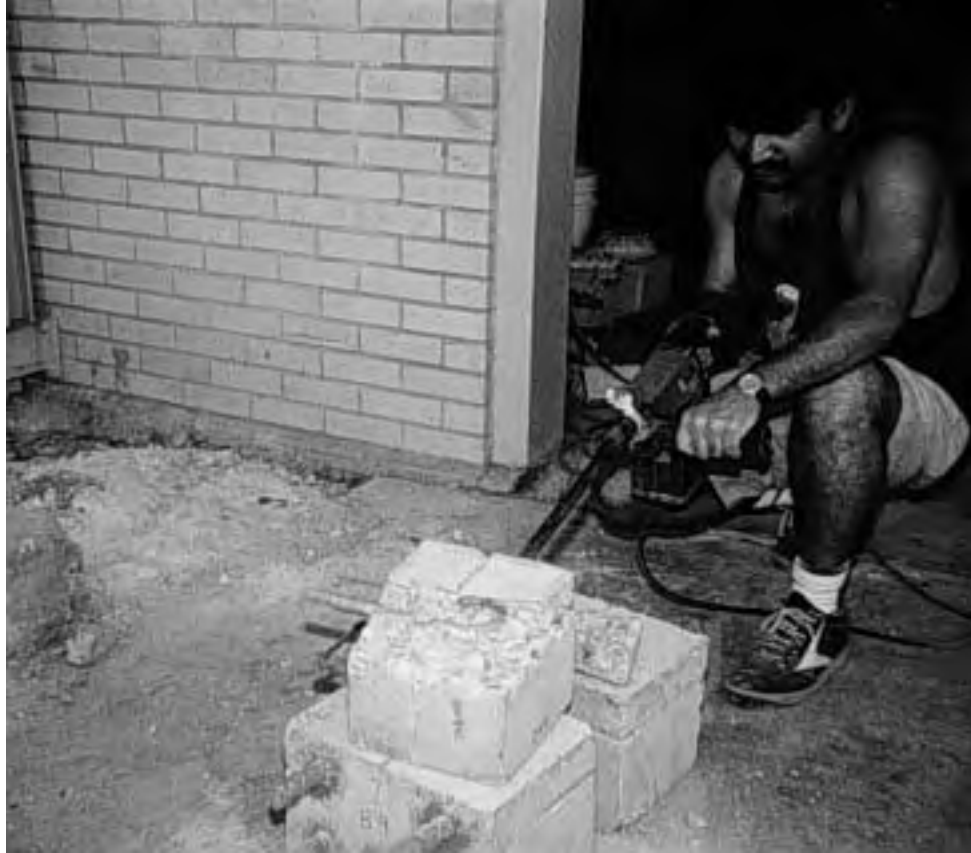
Figure A.27 Demolishing macrocell specimens.
