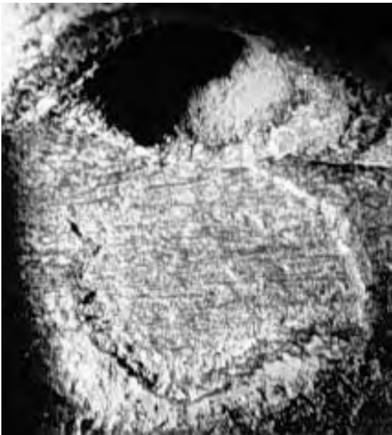
(c) Pitting Inside Blister
