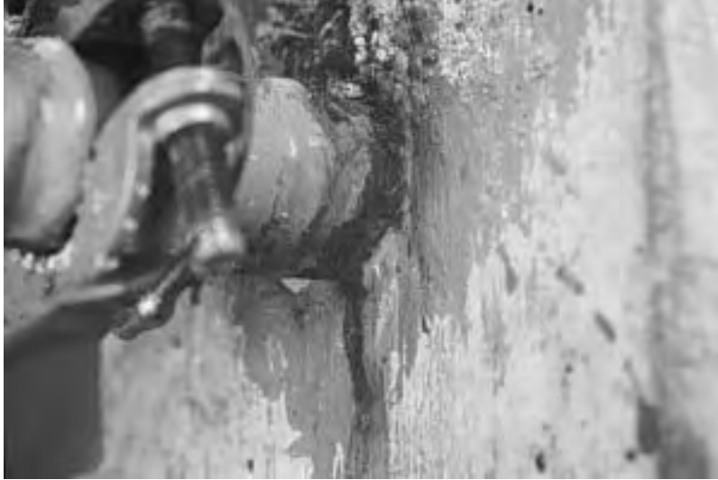
Figure 2.10 Brown solution exuding from protruding bar at front face of specimen.
