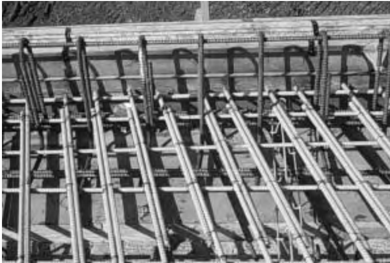
Figure 1.2 Bridge deck construction showing mix of coated and black bars.
