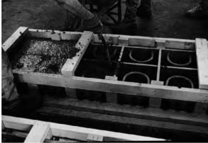
Figure A.15 Casting macrocell specimens.
