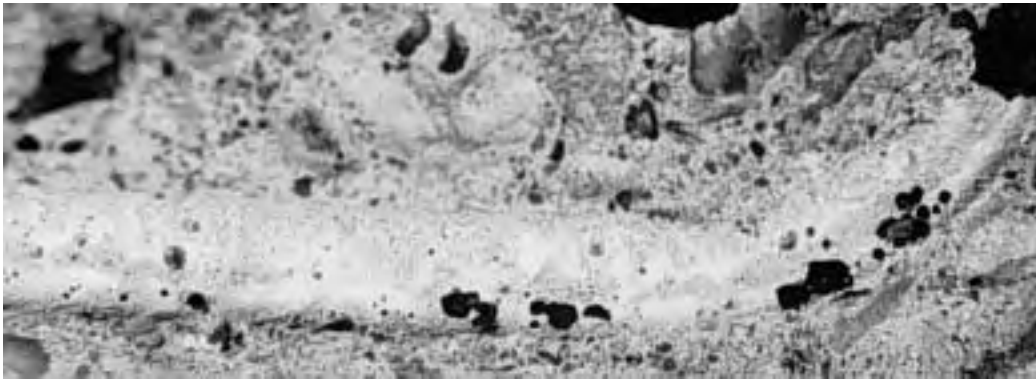
Figure 2.53 White deposits accumulated under coated bar.
