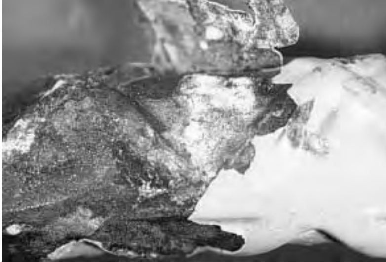
Figure 2.37 Underfilm corrosion (undercutting).
