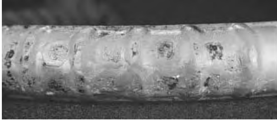
Figure 2.29 Corrosion of patched areas at outside bend on bar 3B.4.
