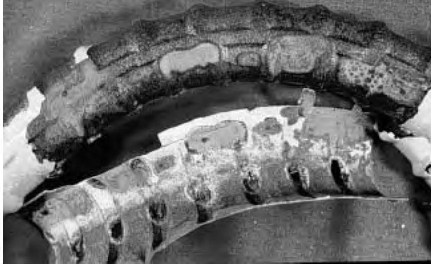
Figure 2.40 Corrosion deposits on bottom side of steel surface.
